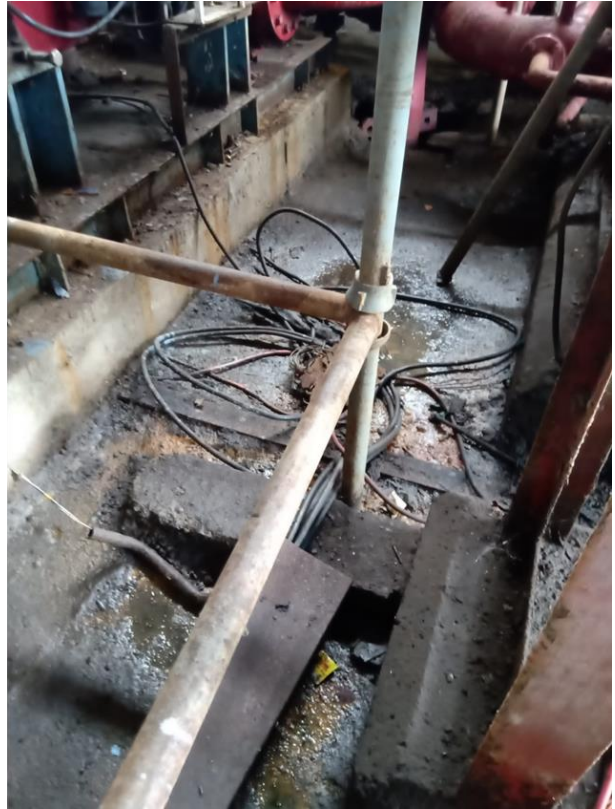
Obstructions for operator's movement due to Scaffolding structure
