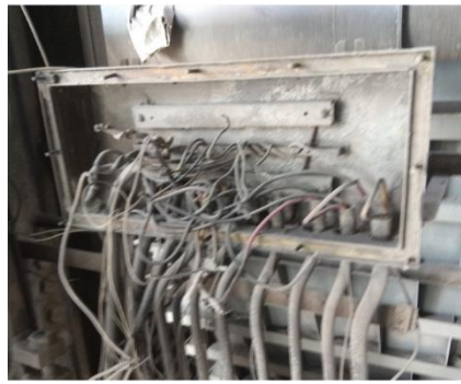
Pulverize fuel leakage from Mills
