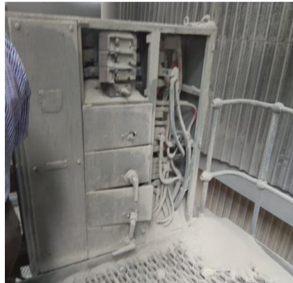
Open electrical boxes on boiler
