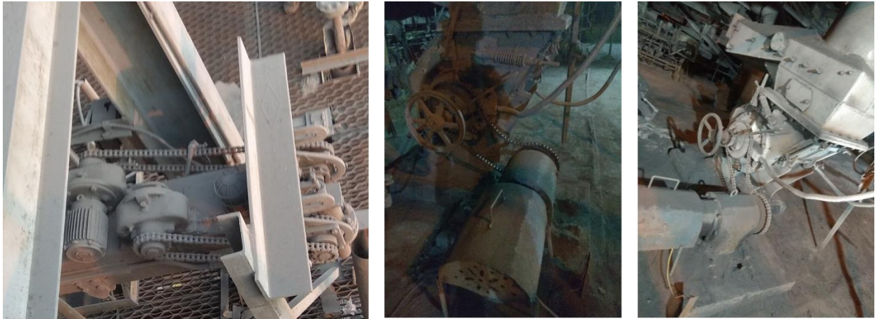
Ash accumulation around hangers in boiler pent house area
