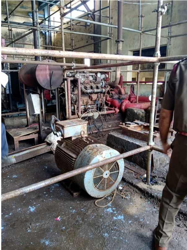
Obstructions for operator's movement due to Scaffolding structure
