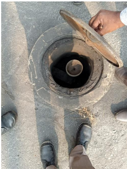
Poorly maintained Earth Pit in Generator Transformer Area
