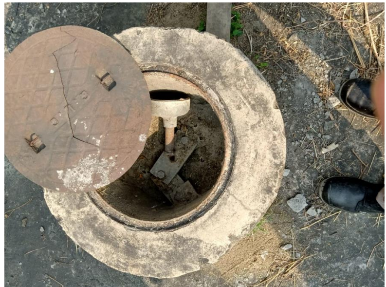
Poorly maintained Earth Pit in Generator Transformer Area
