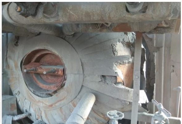
Condition of Insulation in boilers
