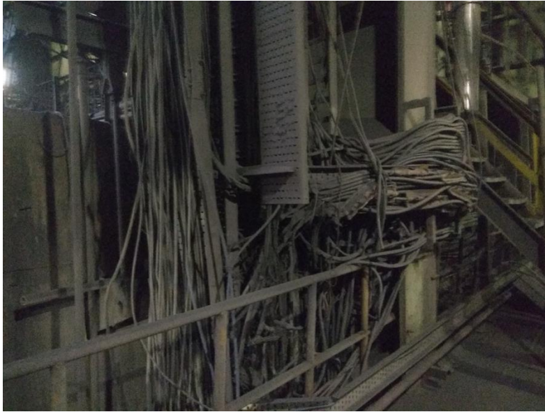
Unorganized cables on boiler
