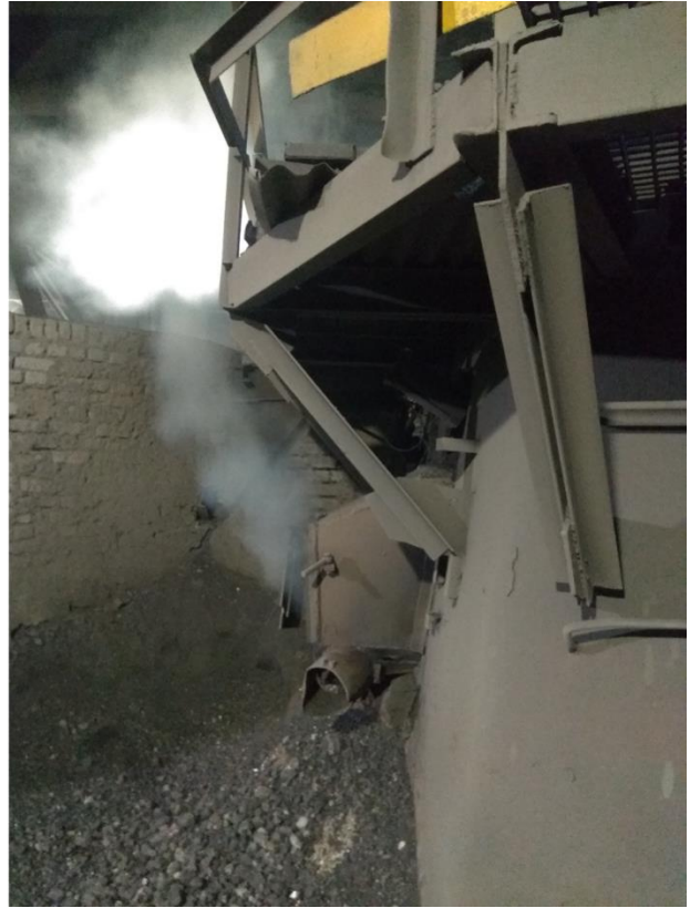
Pulverize fuel leakage from Mills
