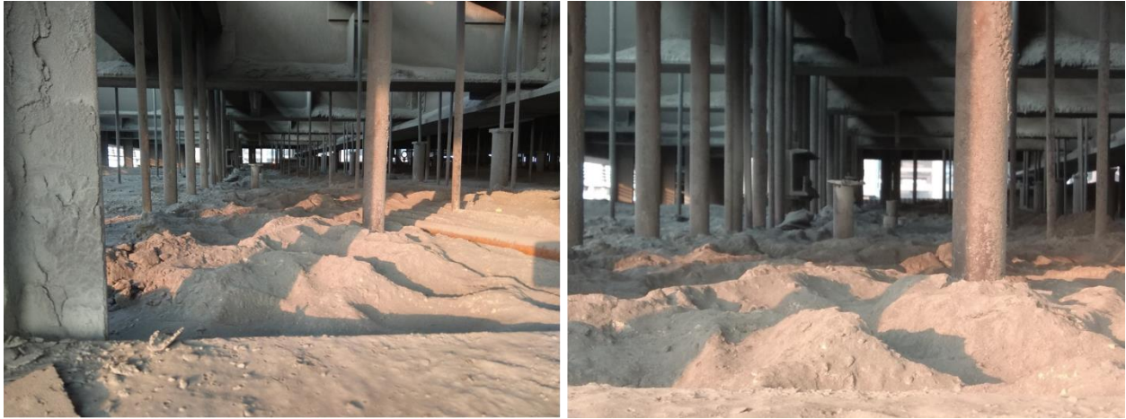
Ash accumulation around hangers in boiler pent house area
