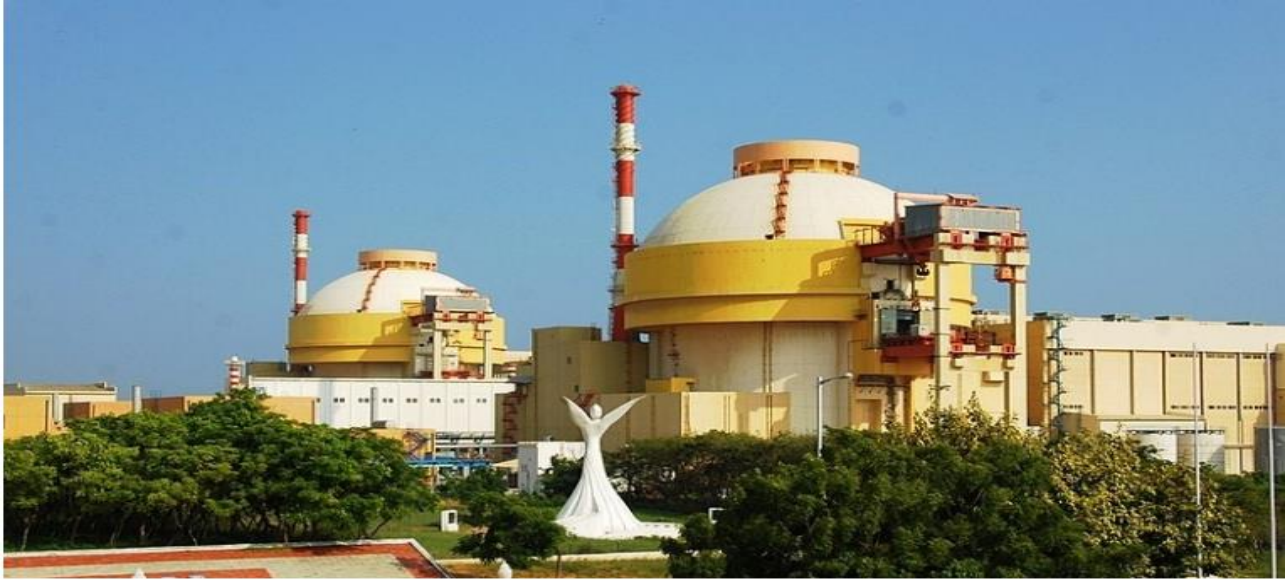
Kudankulam nuclear power plant in Tamil Nadu, southern India. Credit: Reetesh Chaurasia
