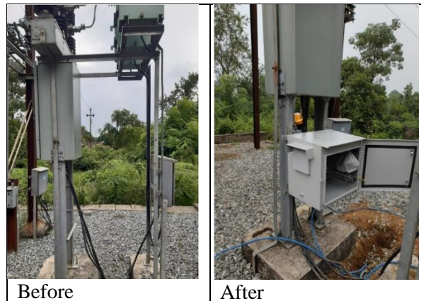
Figure 3. Installation of micro-CRP
