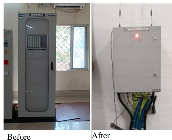
Figure 4. Installation of RTU
