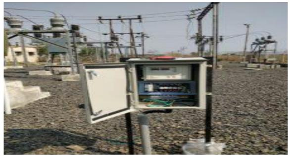
Figure: RT-DAS- Sub-station Monitoring
