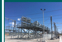
Fixed Series Compensation [FSC]
