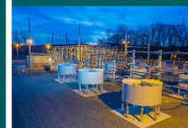
Static VAR Compensator [SVC]
