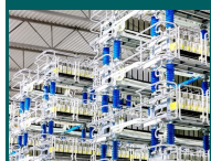
On-shore Voltage Source Converter [VSC]
