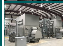
Synchronous Condensers
