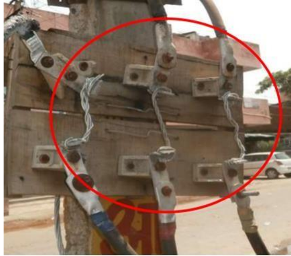
Figure 13: Installation of inappropriate rating & size of fuses
