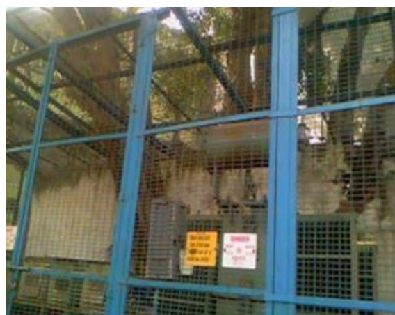
Figure 5: Top Covering by fence
