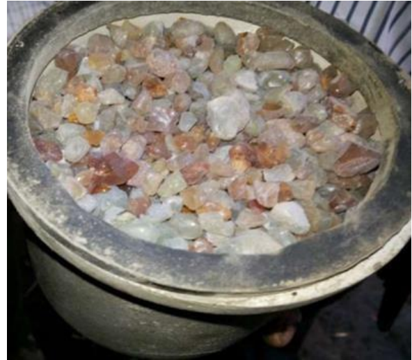
Figure 16: White Silica Gel in Breather
