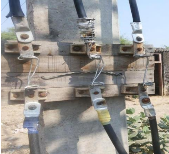
Figure 13: Installation of inappropriate rating & size of fuses
