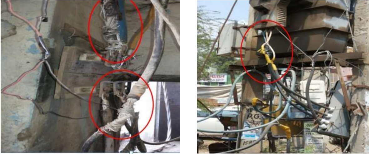
Figure 8: Loose jointed LT Leads
