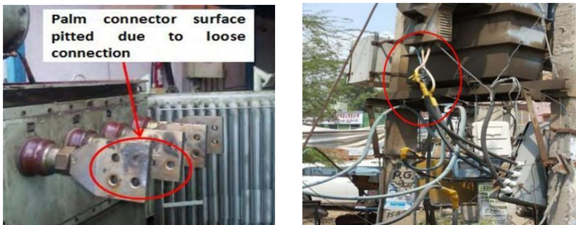
Figure 7: Loose Connection
