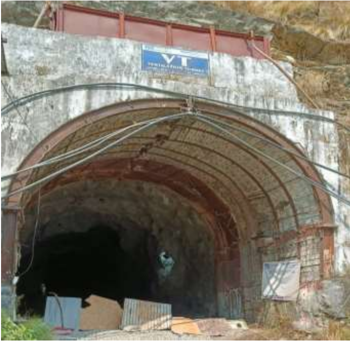
Ventilation Tunnel (VT)
