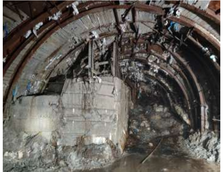
Face 4B (Pedestal of Electrical Tower)
