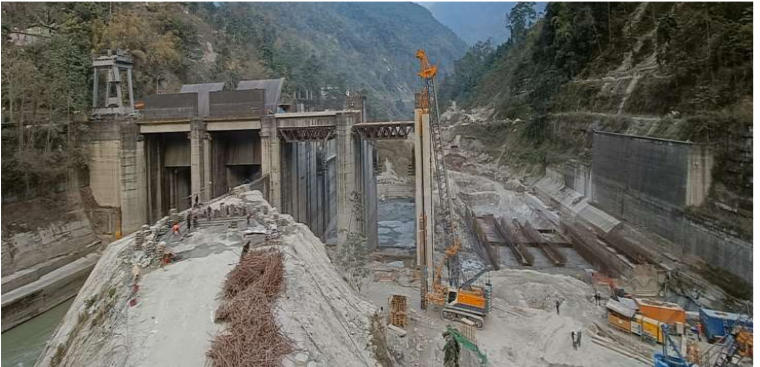
Bays and Cofferd Dyke
