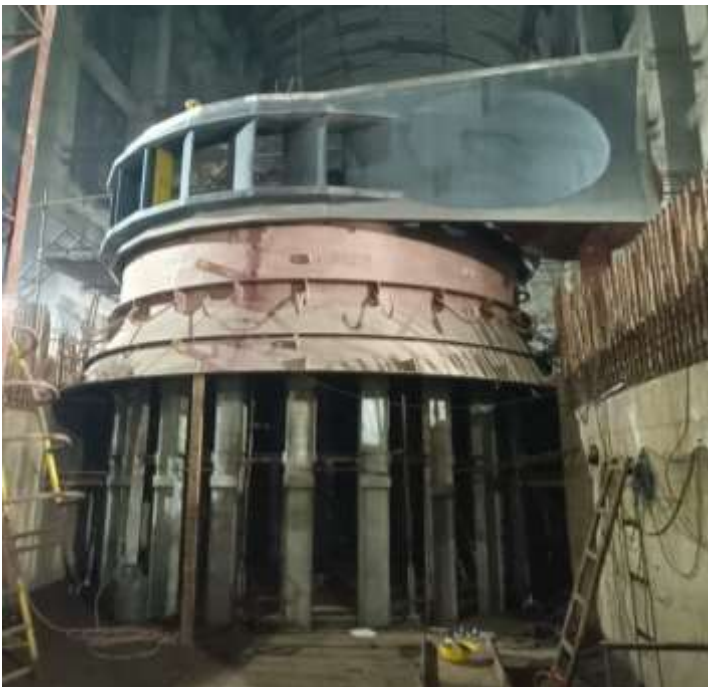
Reinforcement works around Stay Ring
