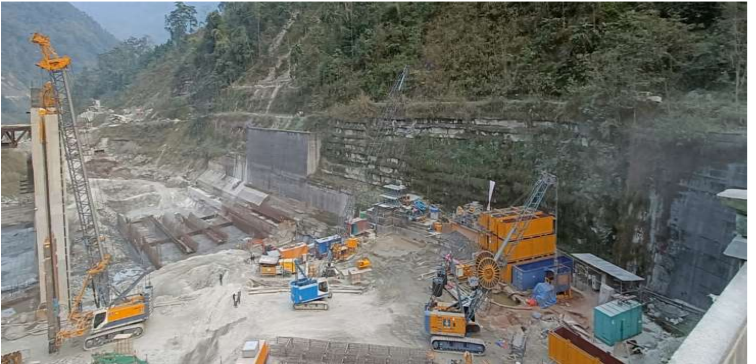
Desilting Basin and Cut-Off Wall
