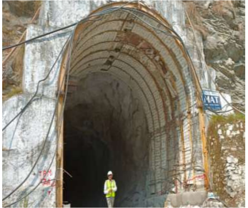
Main Access Tunnel (MAT)
