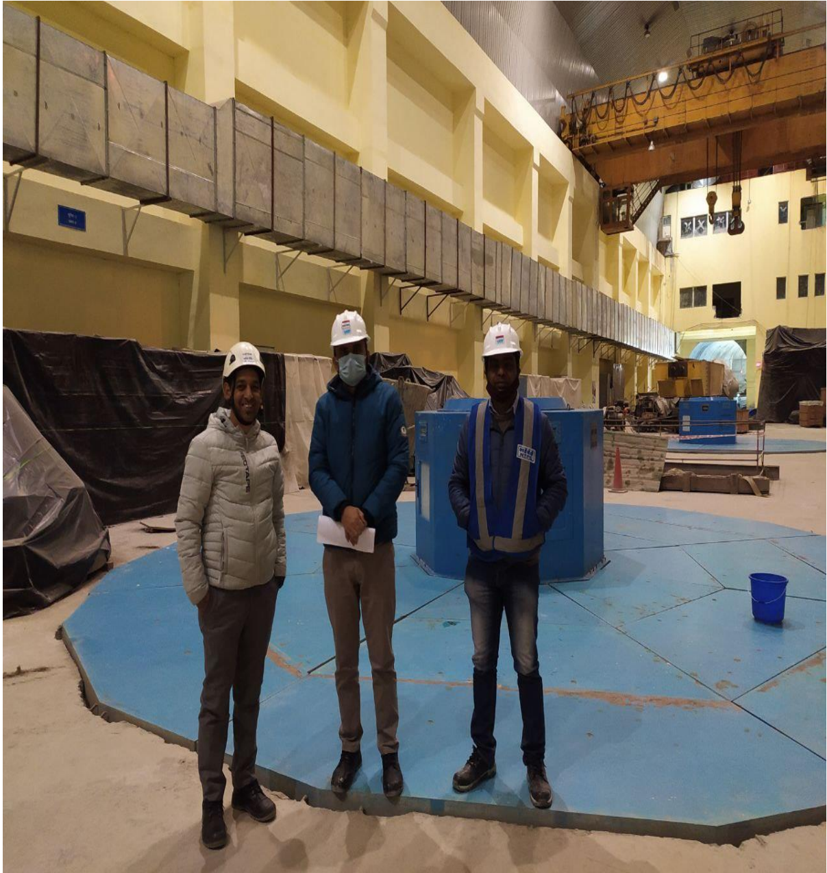
Power House UNIT-1 and Unit-2 Boxed Up
