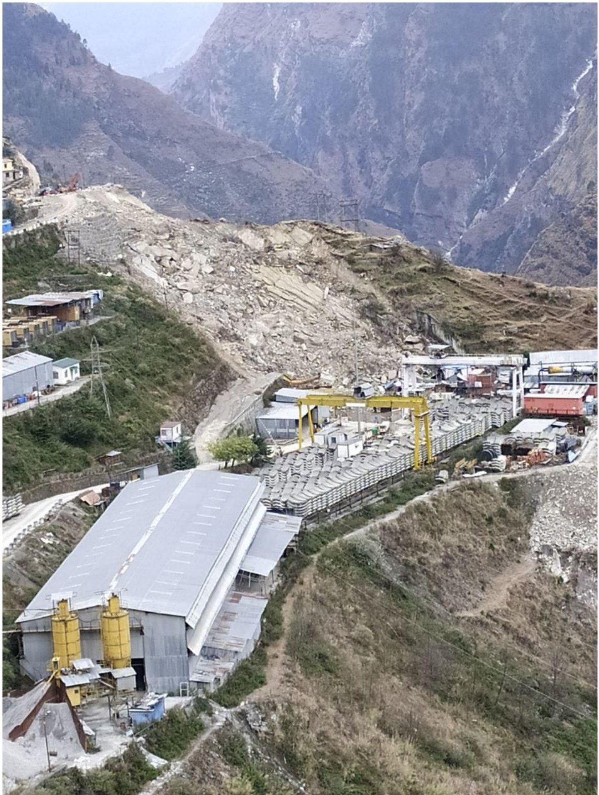
Landslide on TBM portal
