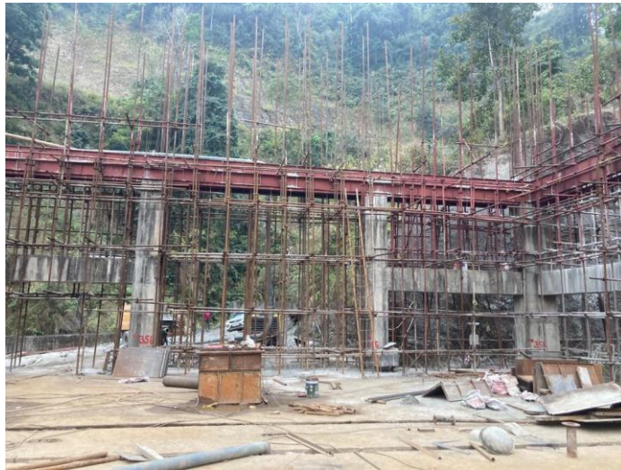
Service bay area
