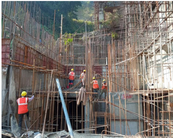
Staircase/lift well area
