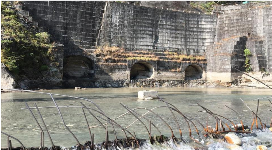
After river diversion
