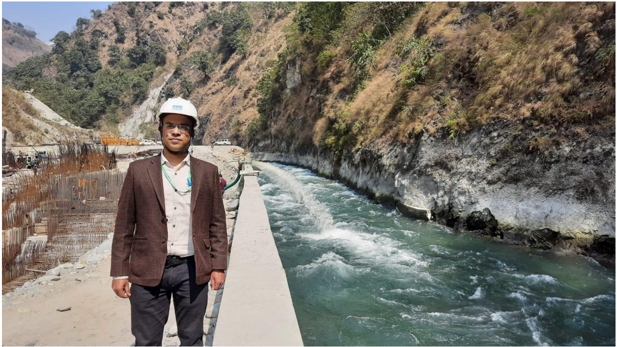
3. View of Diversion channel (1st stage)
