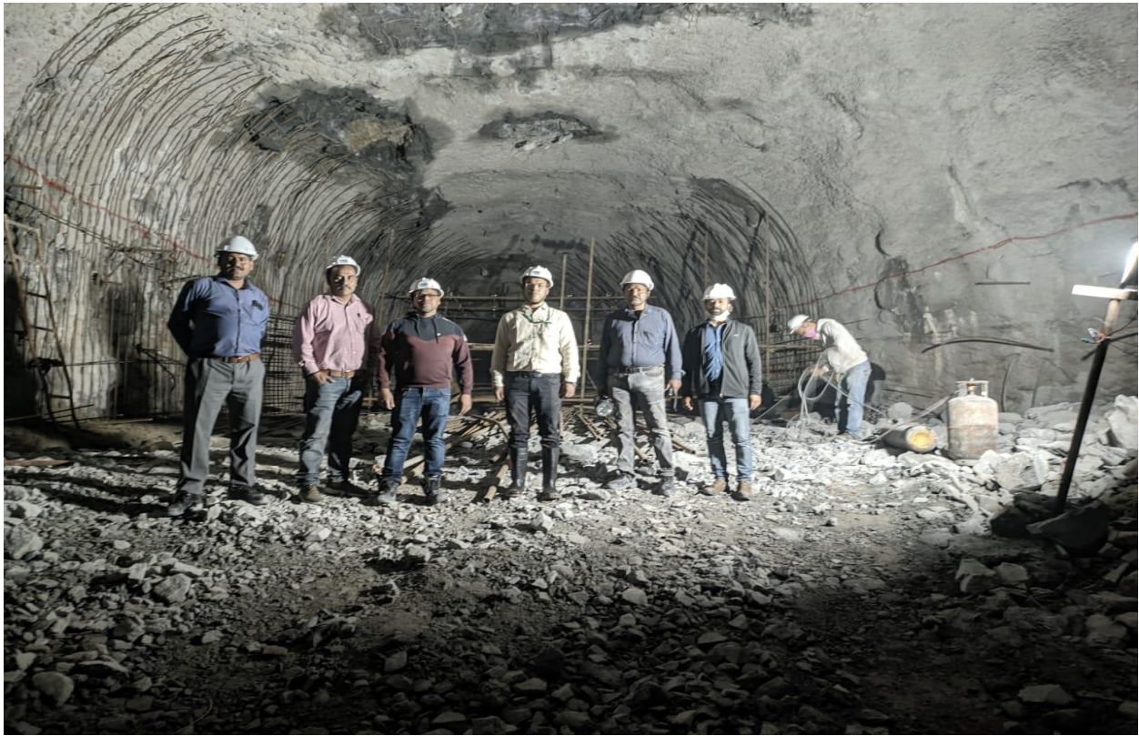
5. View of Desilting Chamber-2 ongoing inlet transition reinforcement works.
