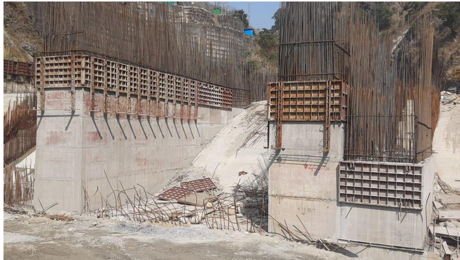
View of Dam structure from D/s
