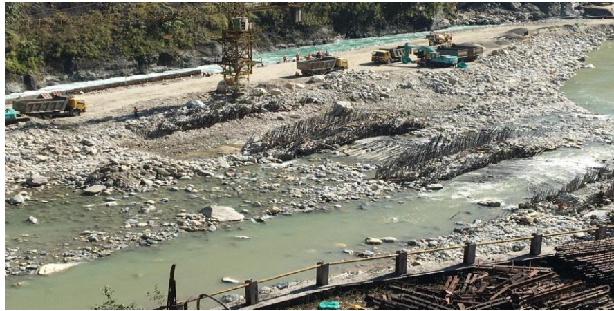
Status of Dam site area after River Diversion
