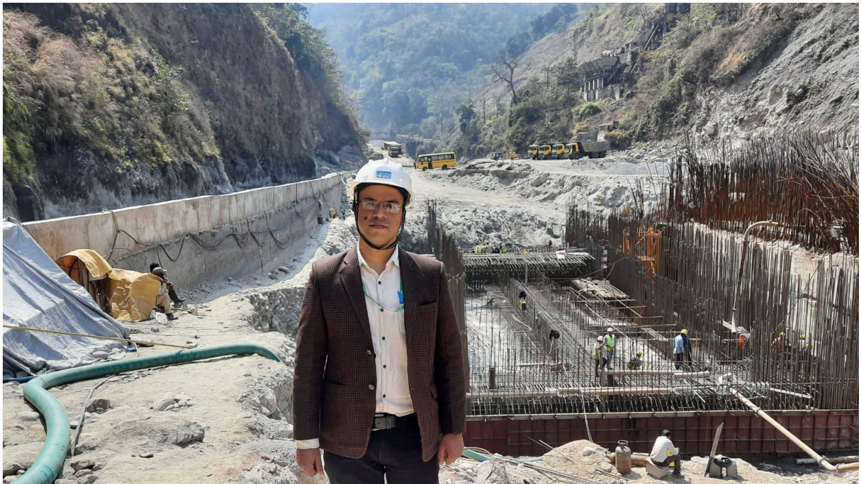
4. Balance work in overflow block no 3 (spillway no 1) is in progress
