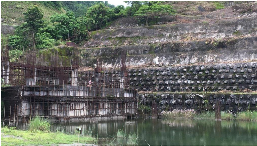
At the time of start of work by NHPC
