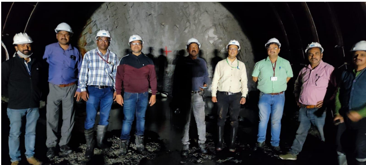
6. View of HRT face-2 ongoing excavation works
