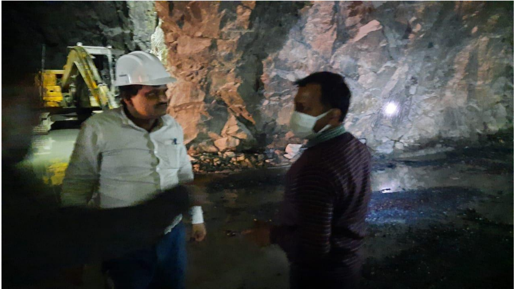
Adit for TRT
