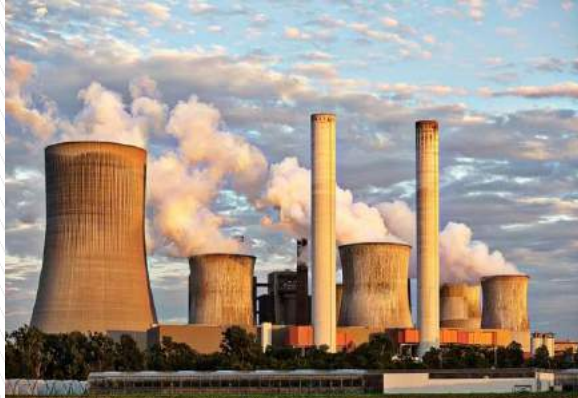
Thermal Power Plants
