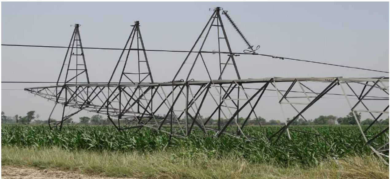
Tower at Loc. No. 272
