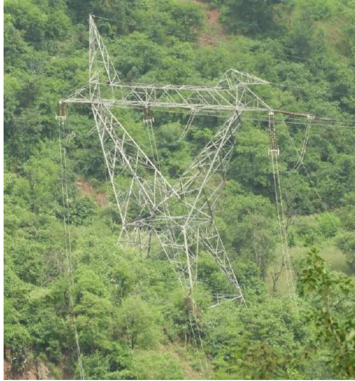
Tower at Loc. No. 239
