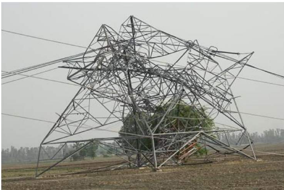
Tower at Loc. No. 60
