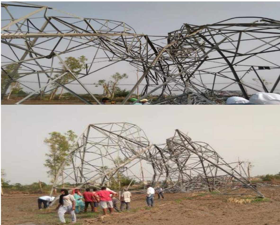
Tower at Loc. No.58
