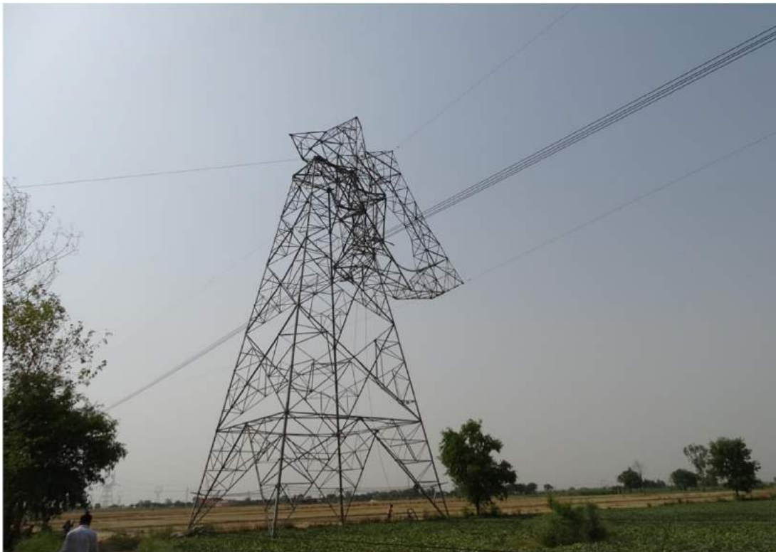
Tower at Loc. No 568 (A+0)
