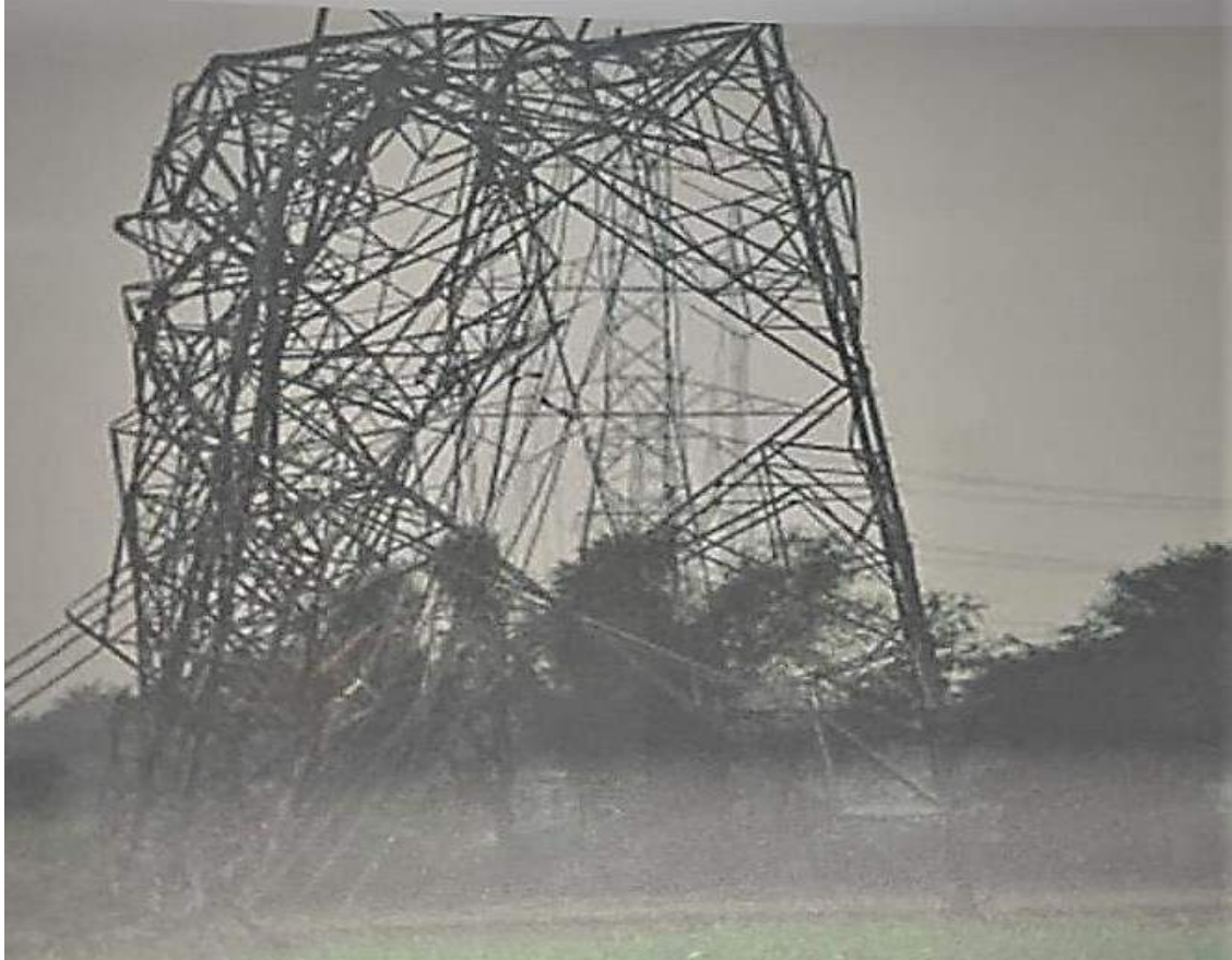
Tower at Loc. No. 63
