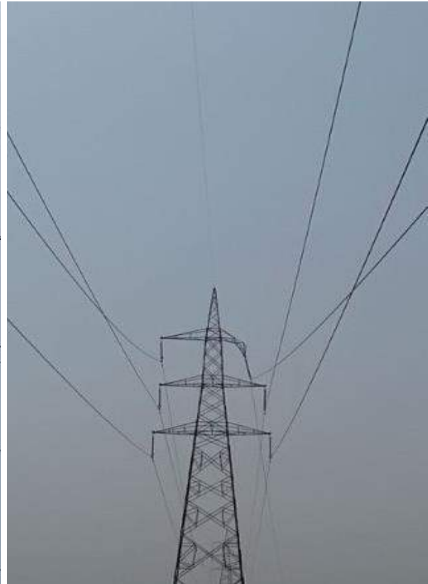
Tower at Loc. No. 267
