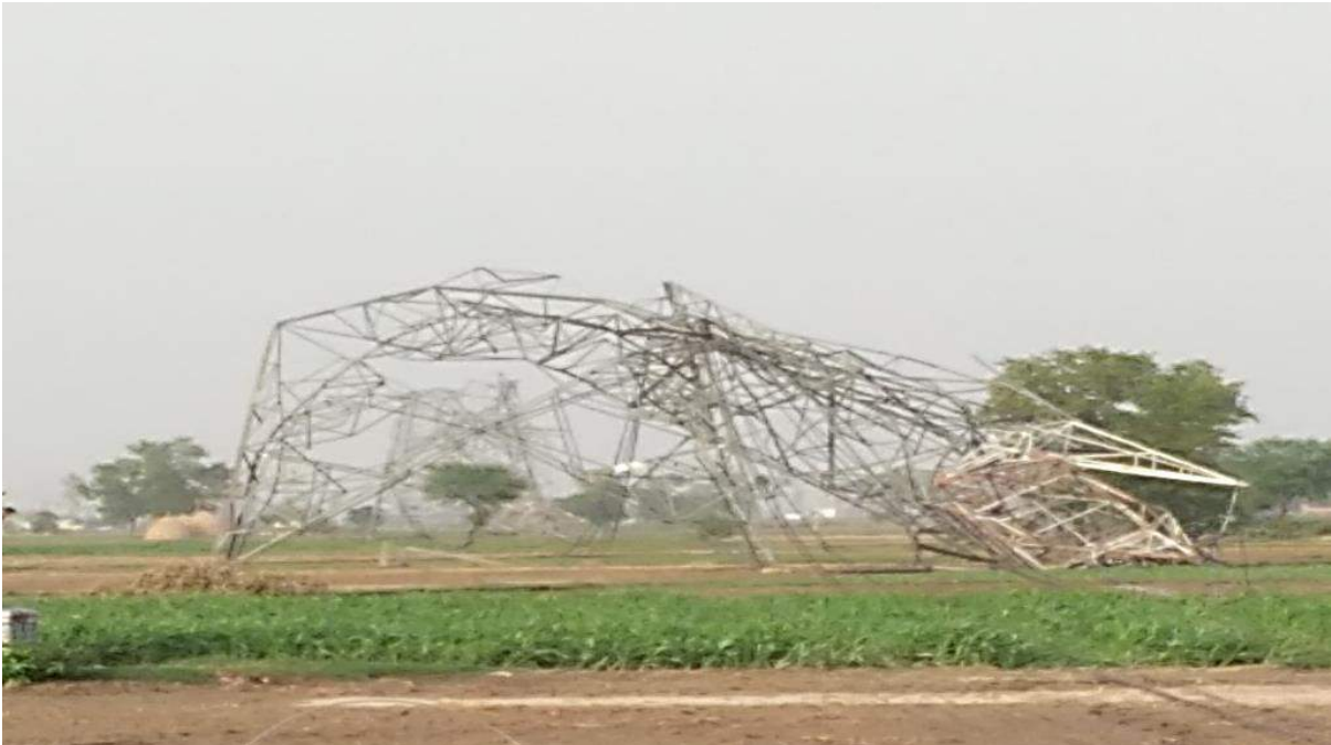
Tower at Loc. No. 62
