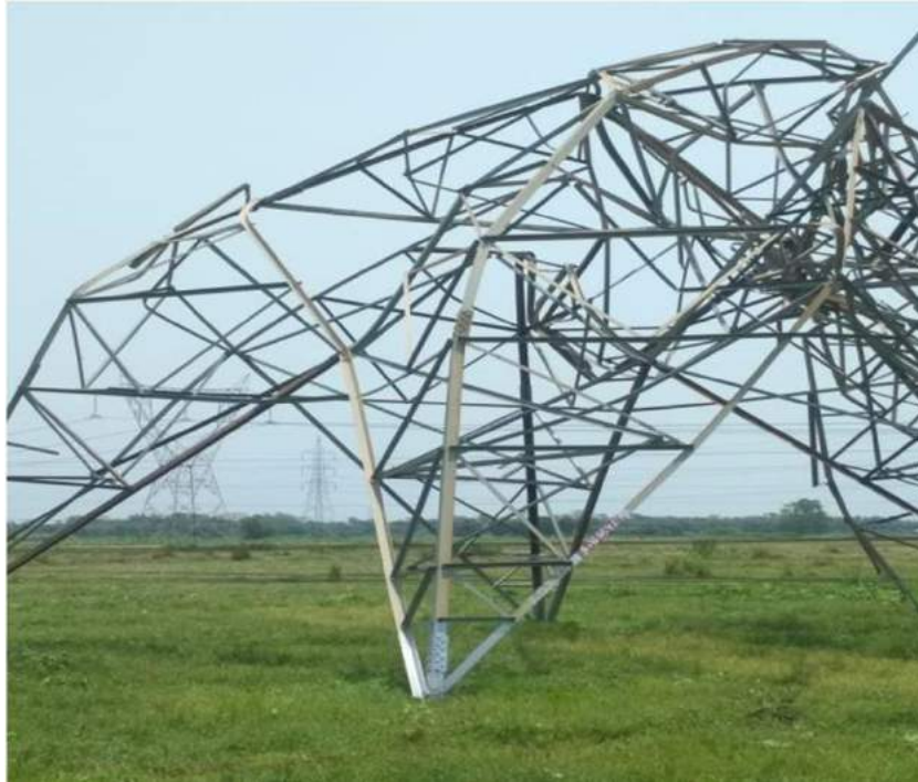
Tower at Loc. No. 378 (A+0)
