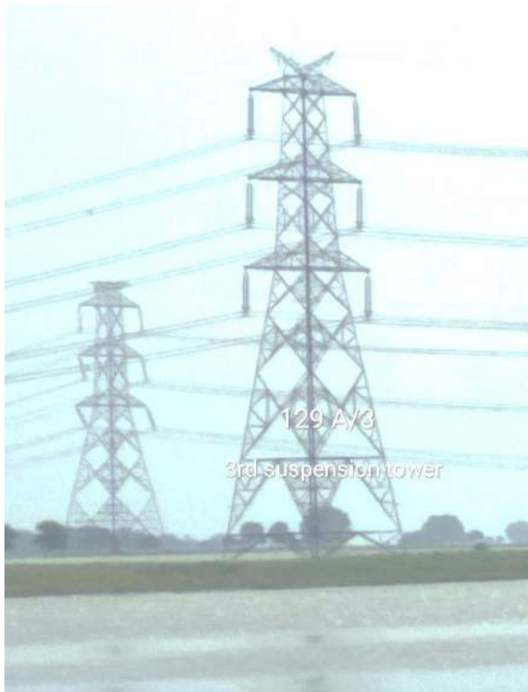
Tower at Loc. No. 129A/3
