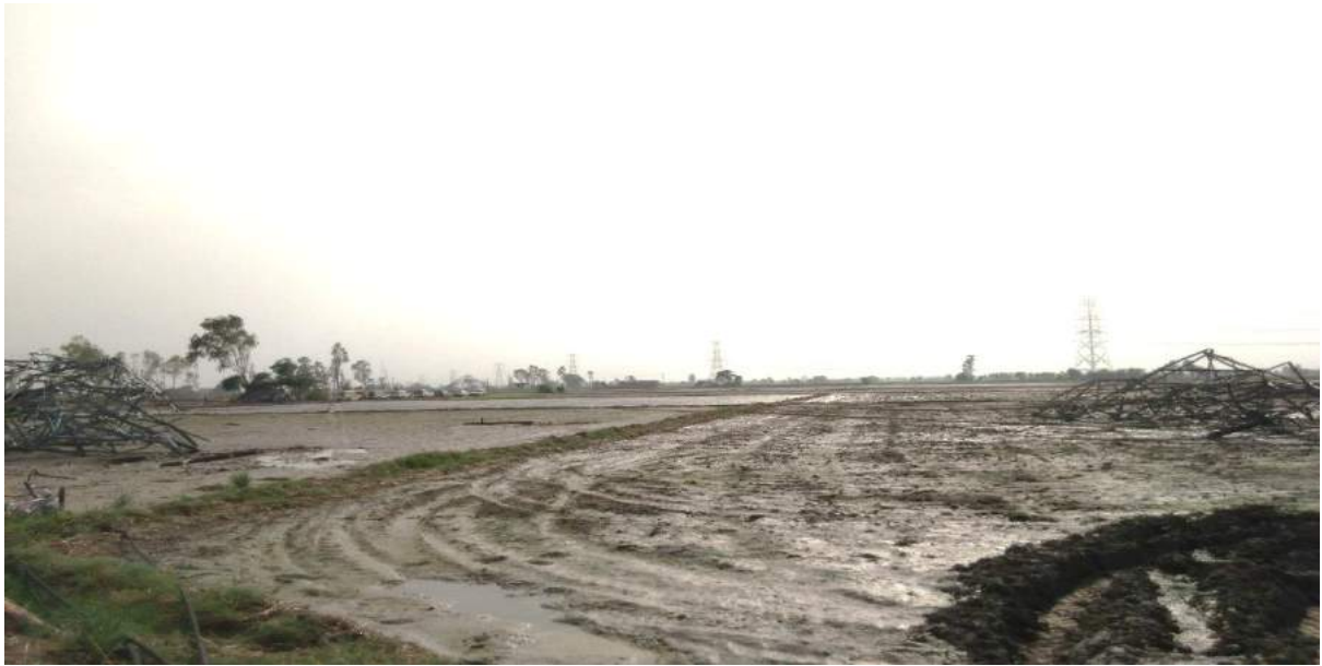
Tower at Loc. No. 57
