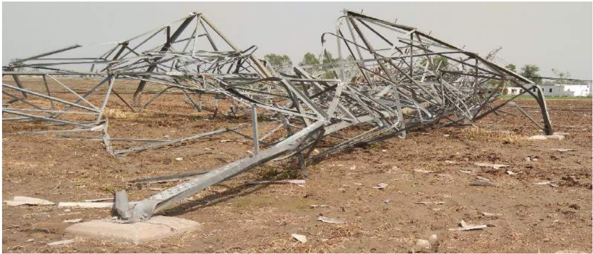
Tower at Loc. No. 55
