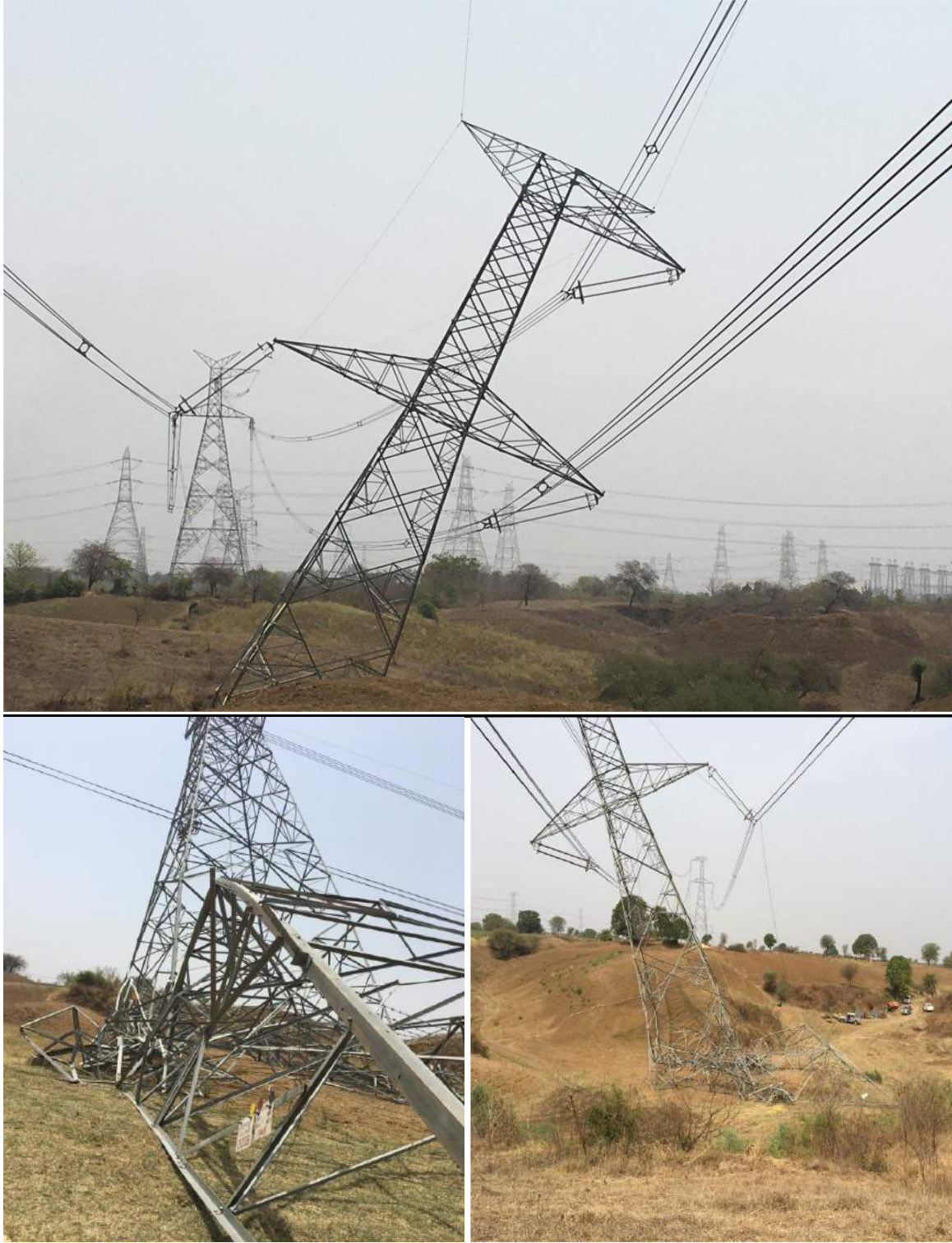
Tower at location no 2A/3
