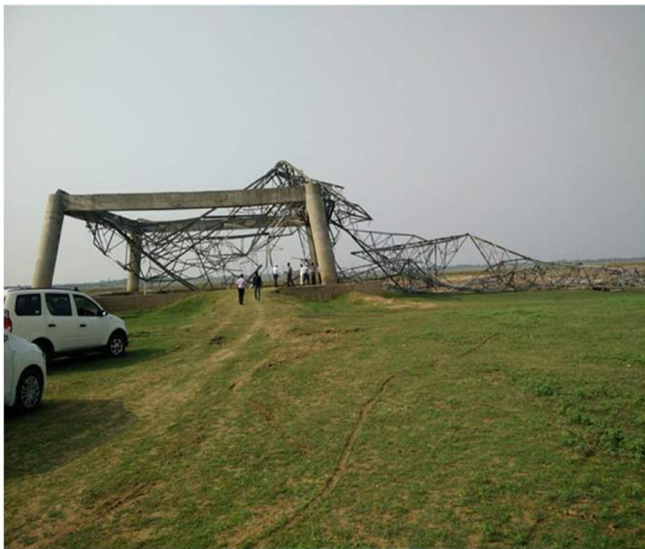
Tower at Loc. No. 64
