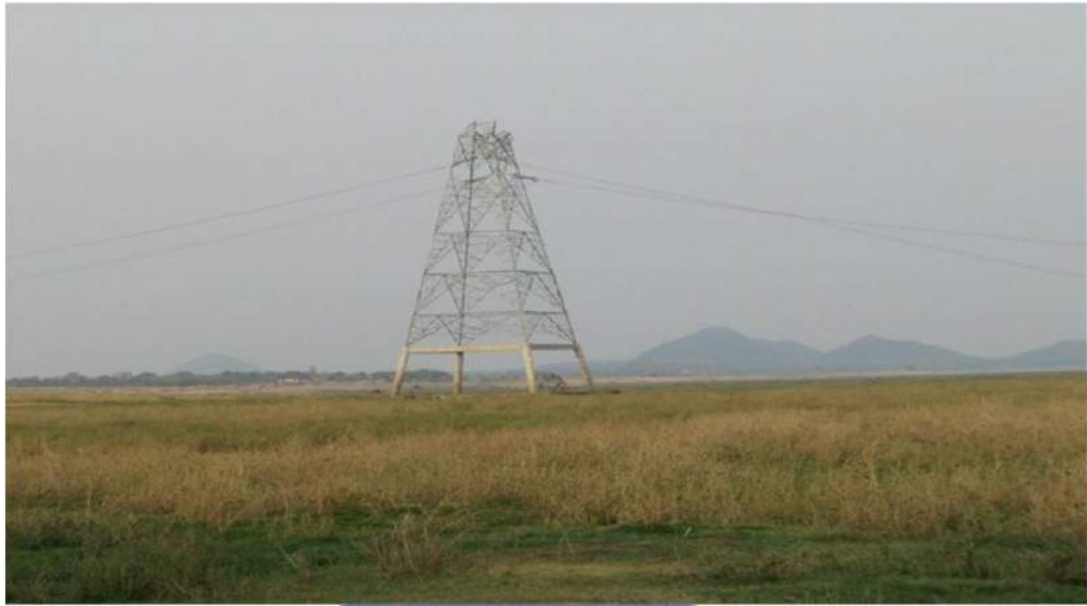
Tower at Loc. No. 63
