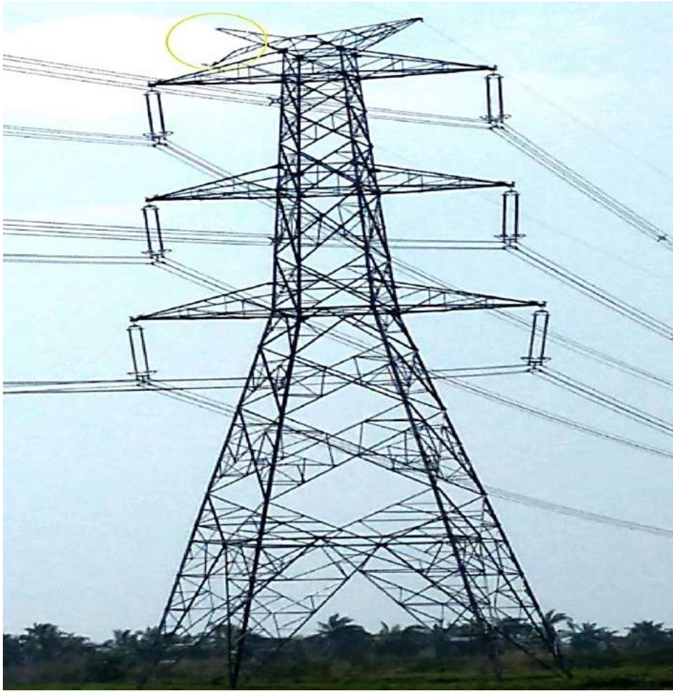
Tower at location no. 15/2
