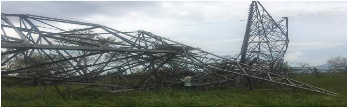
Tower at location no 952 (DA+3)
