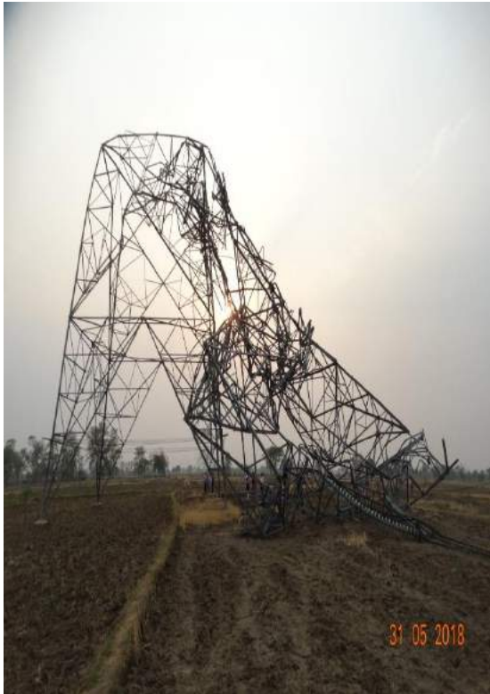
Tower at Loc. No. 184
