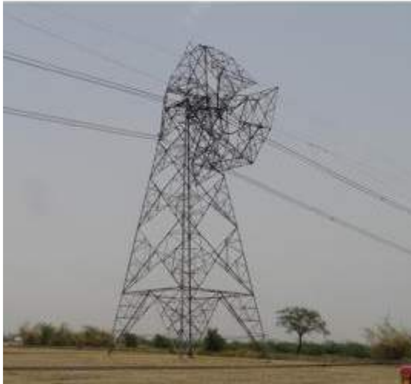
Tower at Loc. No. 17 (A+0)
