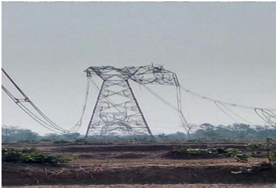
Tower at Loc. No. 121
