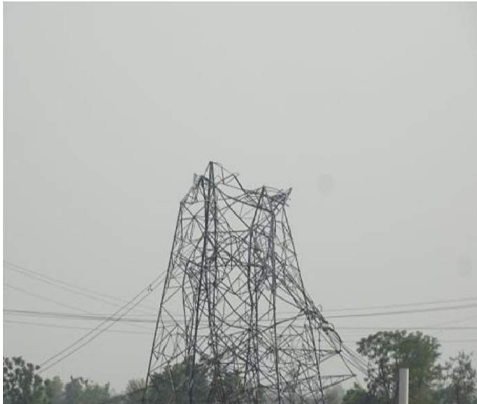
Tower at Loc. No. 61
