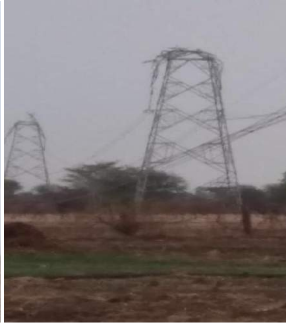
Tower at Loc. No. 573
