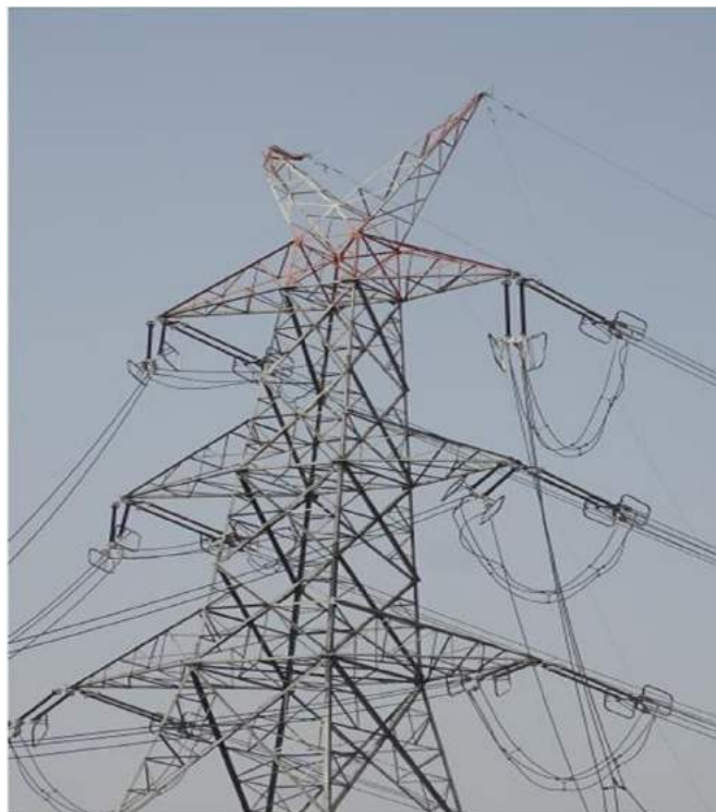
Tower at Loc. No. 54
