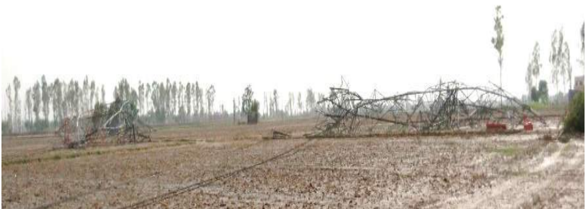
Tower at Loc. No. 56
