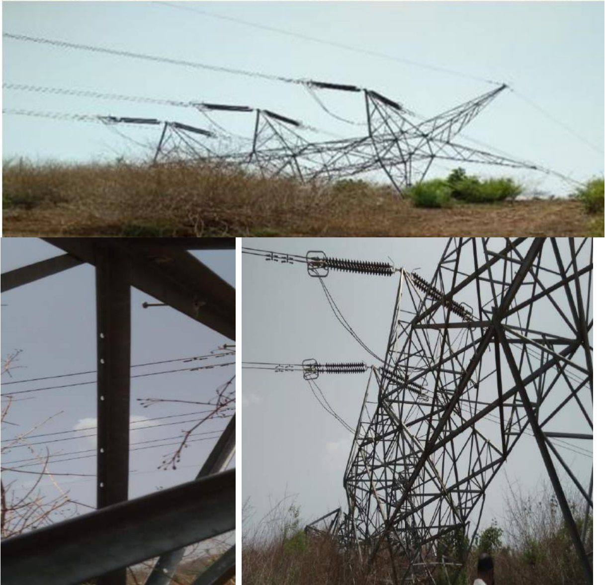
Tower at Loc. No. 219
