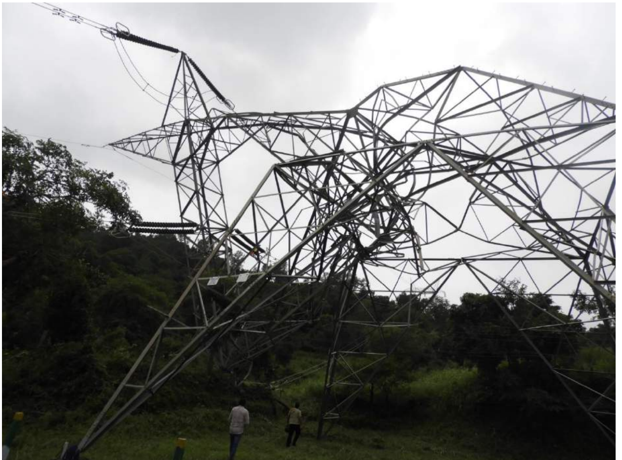
Tower at Loc. No. 238
