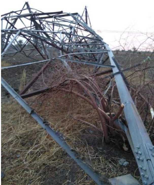
Tower at Loc. No. 570
