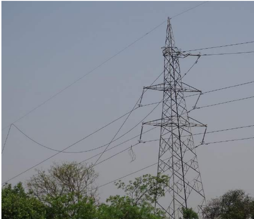
Tower at Loc. No. 269
