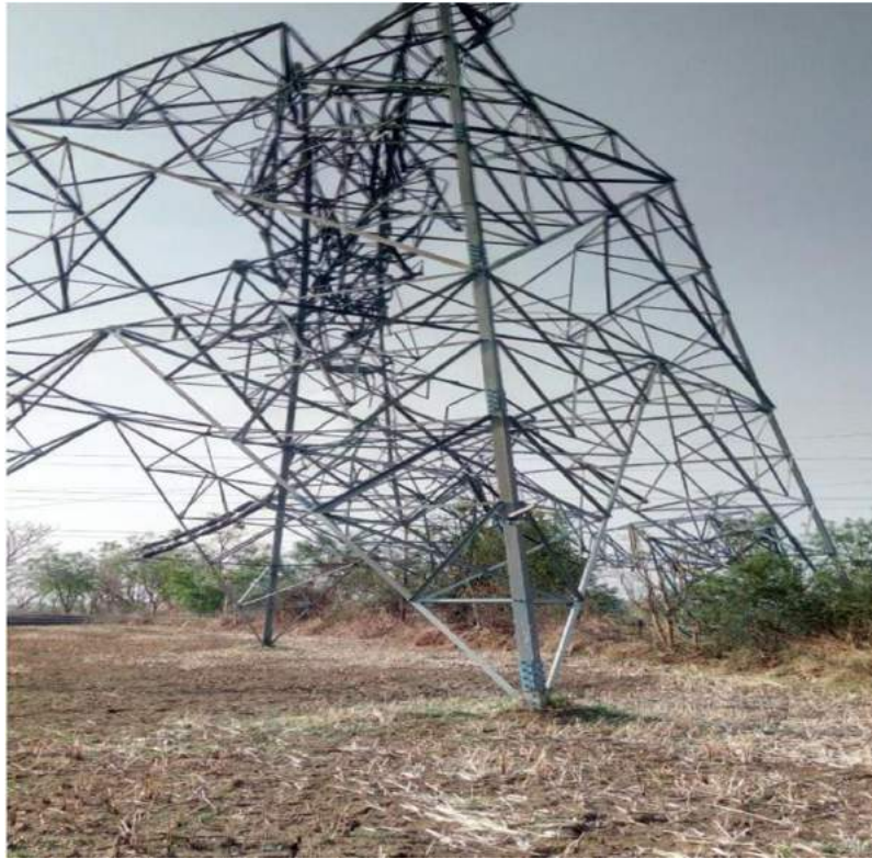
Tower at Loc. No. 120
