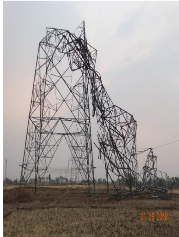
Tower at Loc. No. 186
