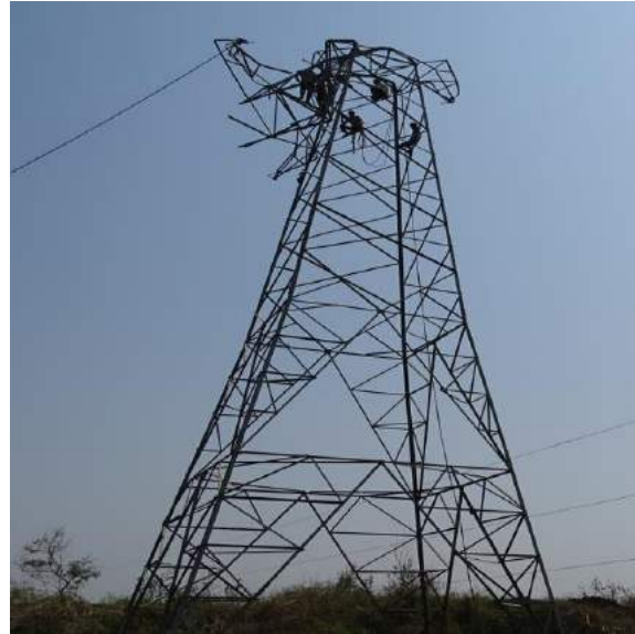
Damaged APTRANSCO's transmission line
