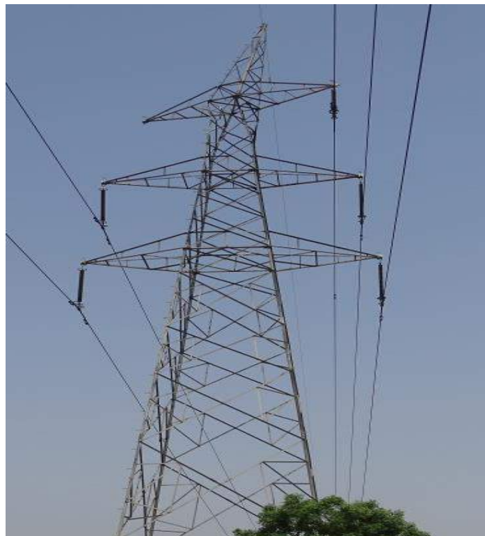
Tower at Loc. No. 268
