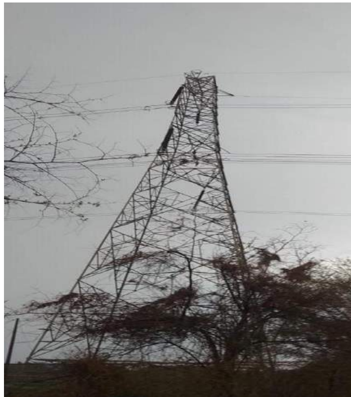
Tower at Loc. No. 574
