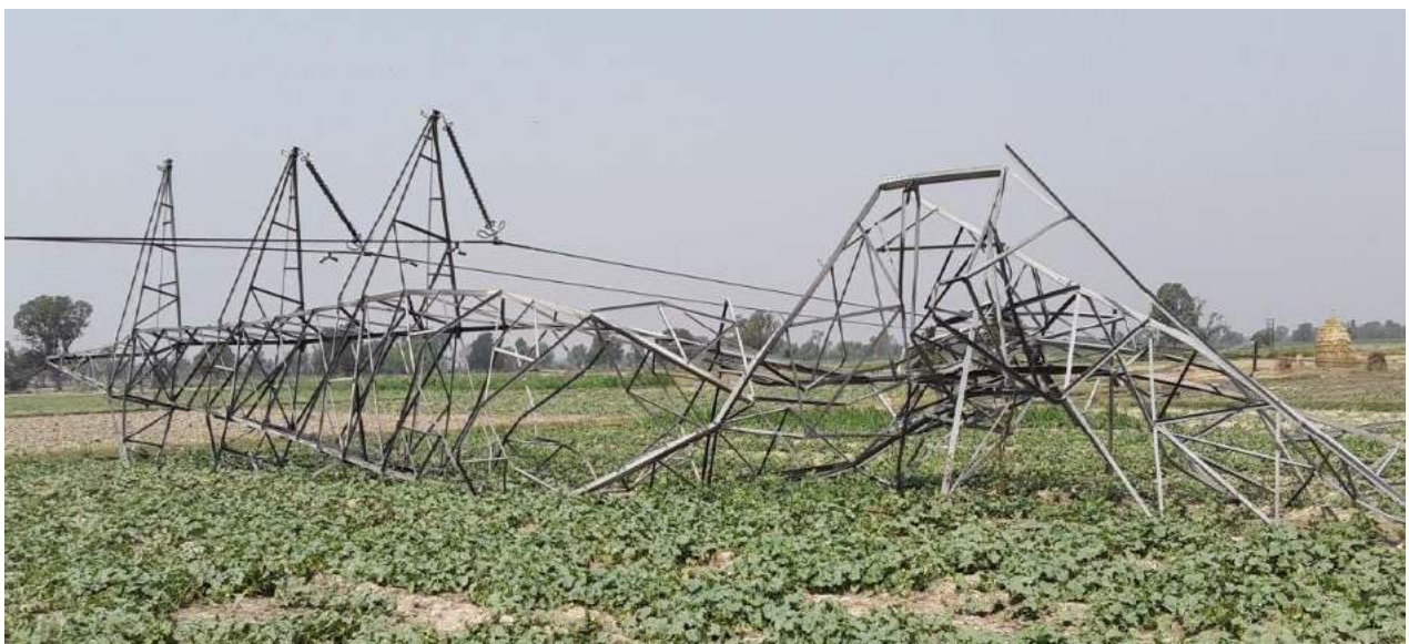
Tower at Loc. No. 270
