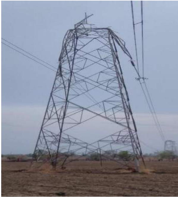
Tower at Loc. No. 572
