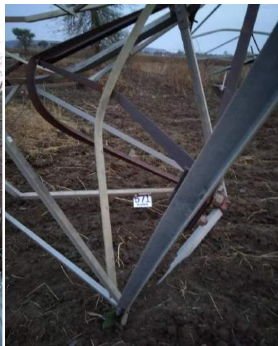
Tower at Loc. No. 571
