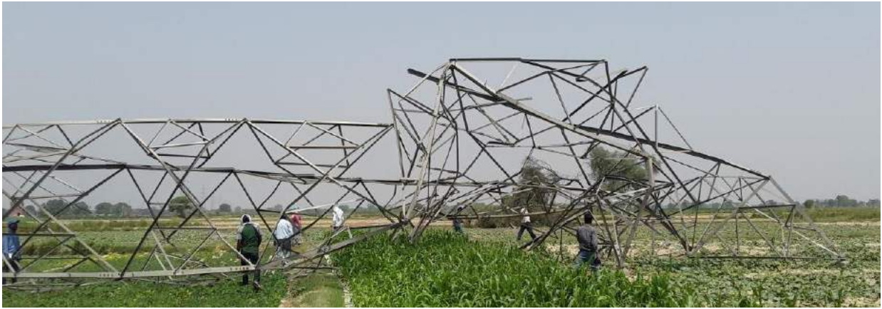
Tower at Loc. No. 271
