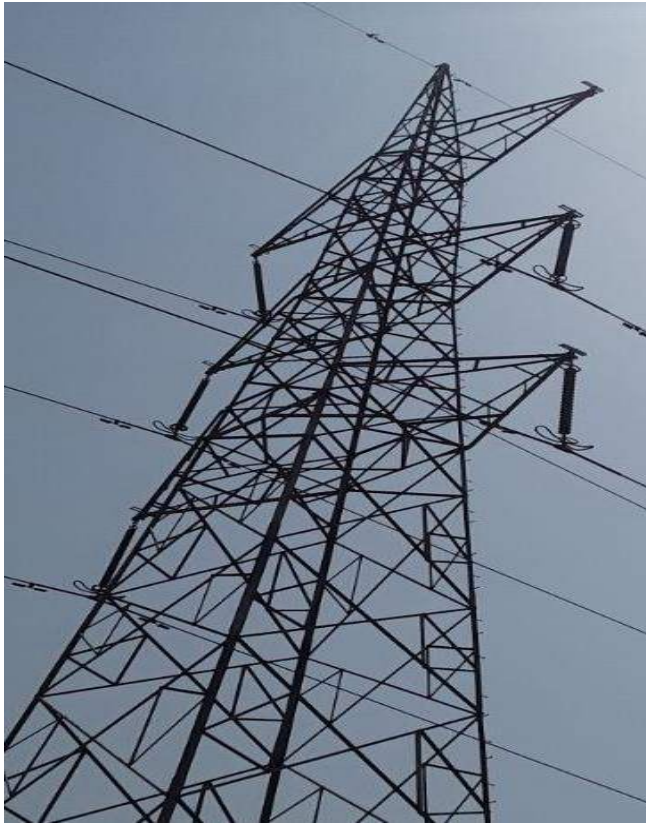
Tower at Loc. No. 266
