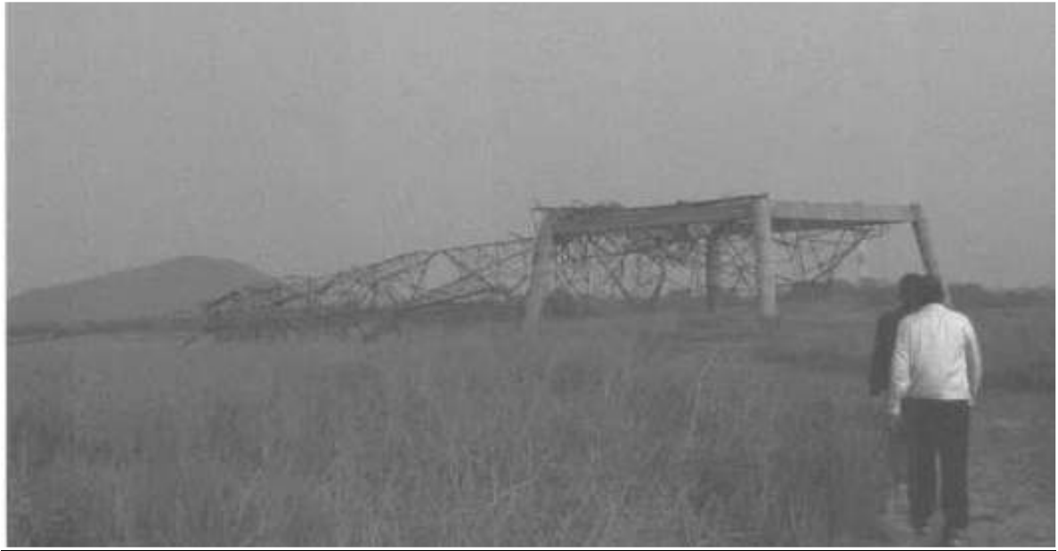
Probable Cause of Tower at Loc. No. 64
