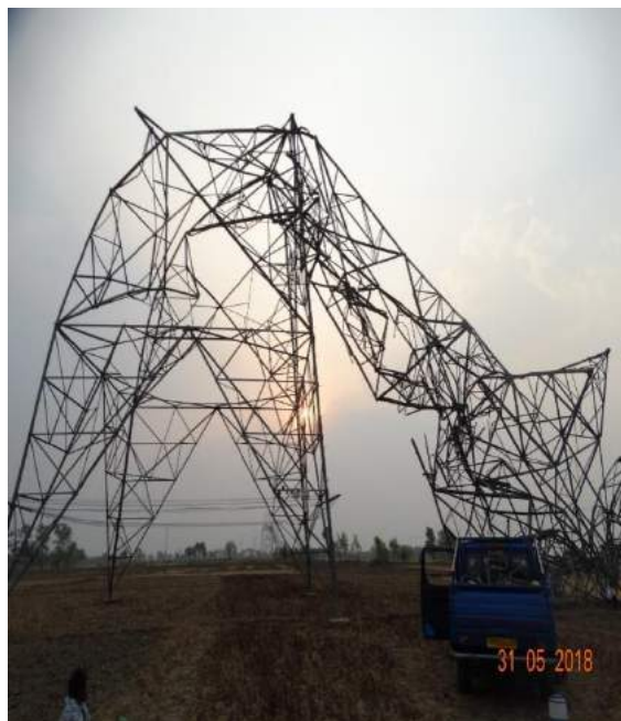
Tower at Loc. No. 185
