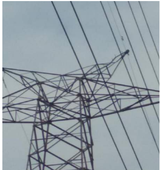
Tower at Loc. No. 38
