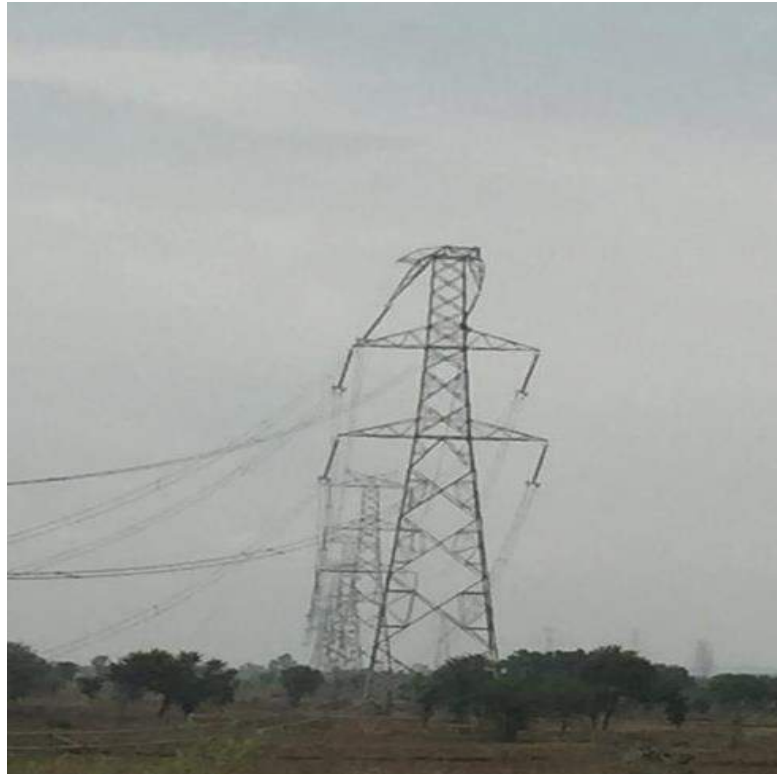
Tower at Loc. No. 569
