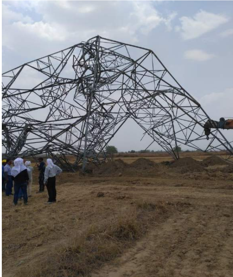
Tower at Loc. No. 63(A+0)
