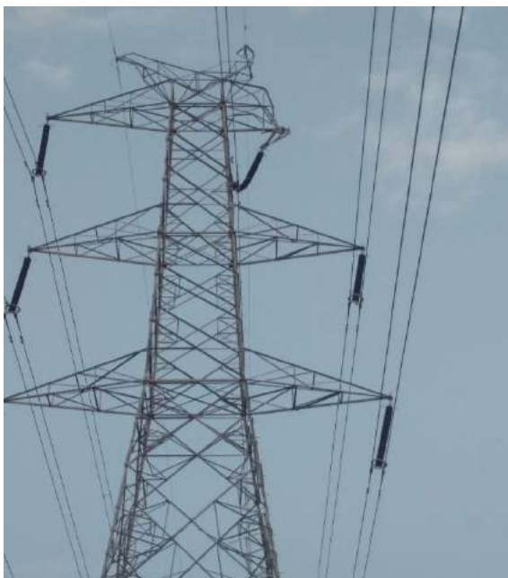
Tower at Loc. No. 37
