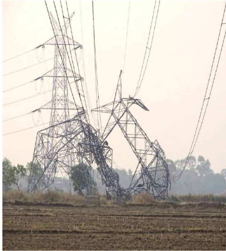
Tower at Loc. No. 36
