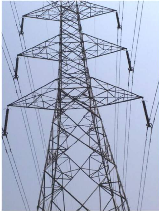
Tower at Loc. No. 407(DA+0)
