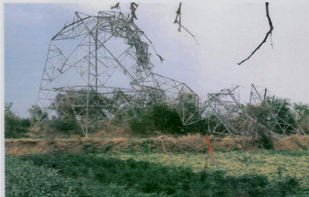
Tower at Loc. No. 122
