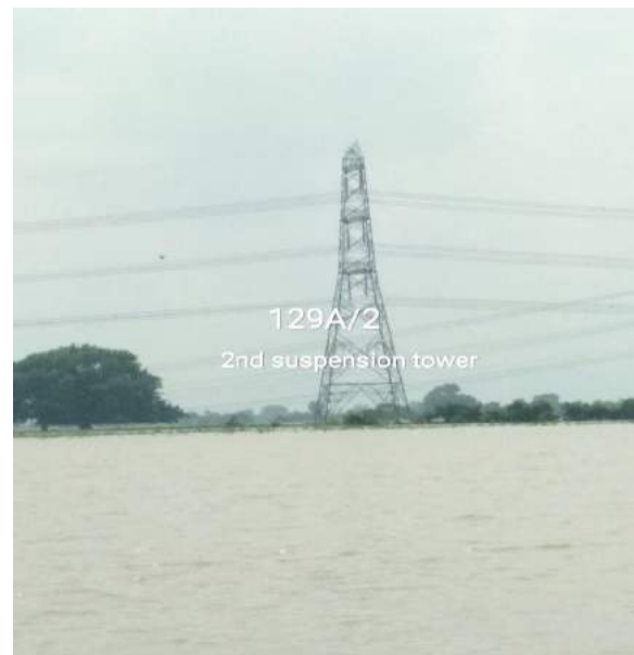
Tower at Loc. No. 129A/2
