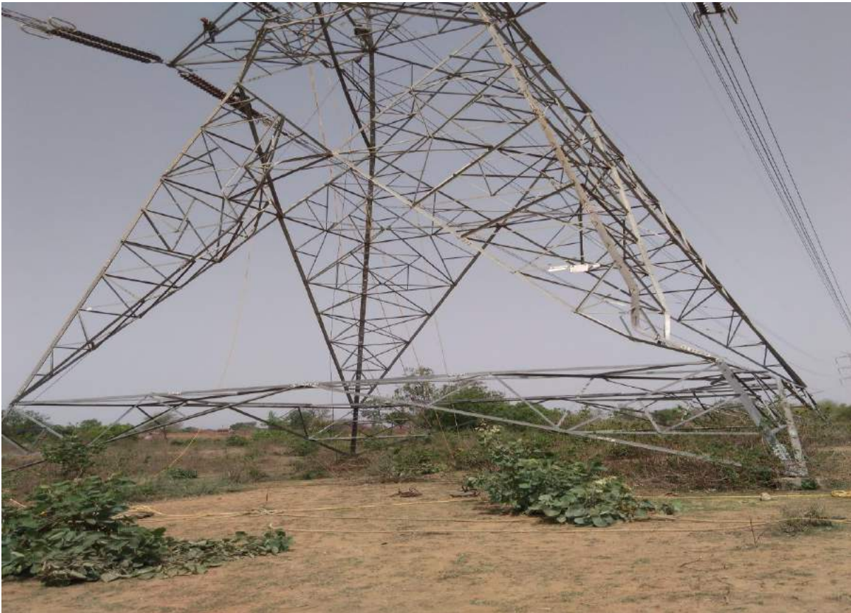
Tower at Loc. No. 220
