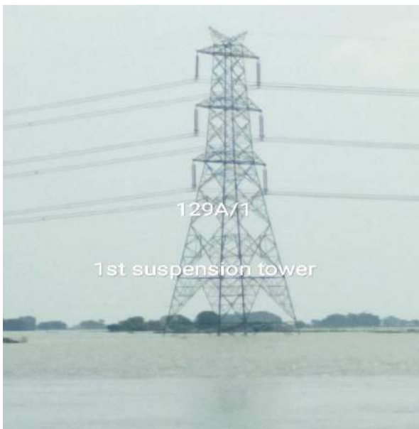
Tower at Loc. No. 129A/1
