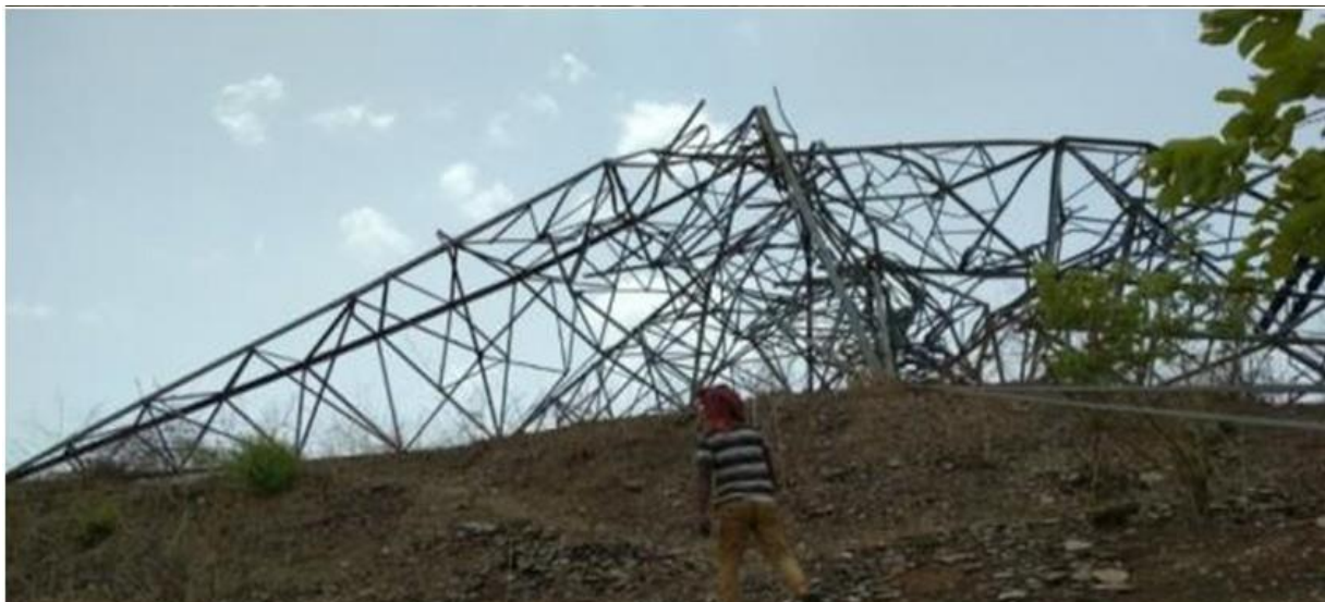
Tower at Loc. No. 218
