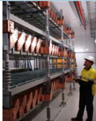
Full Bridge MMC as used for power frequency conversion and reactive power compensation in Industry and Energy applications
