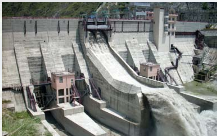
Nathpa Jhakri - Dam
