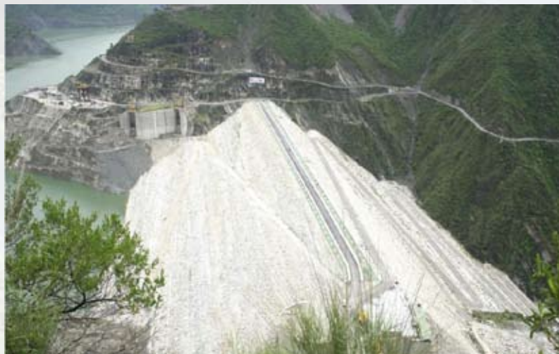
Tehri HPP - Dam
