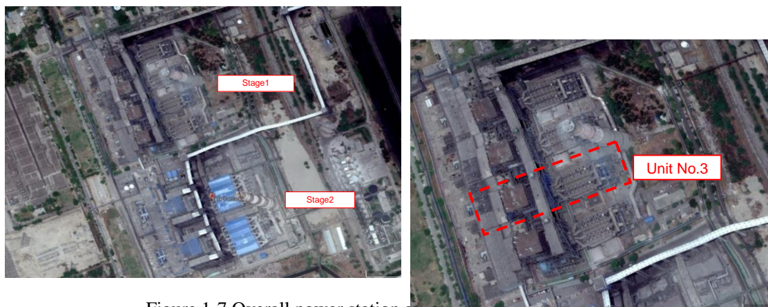
Figure 1-7 Overall power station area (left), the plant area (right)
