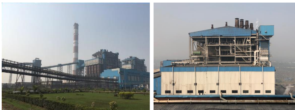
Figure 1-1 Full view of the power plant and boiler building
