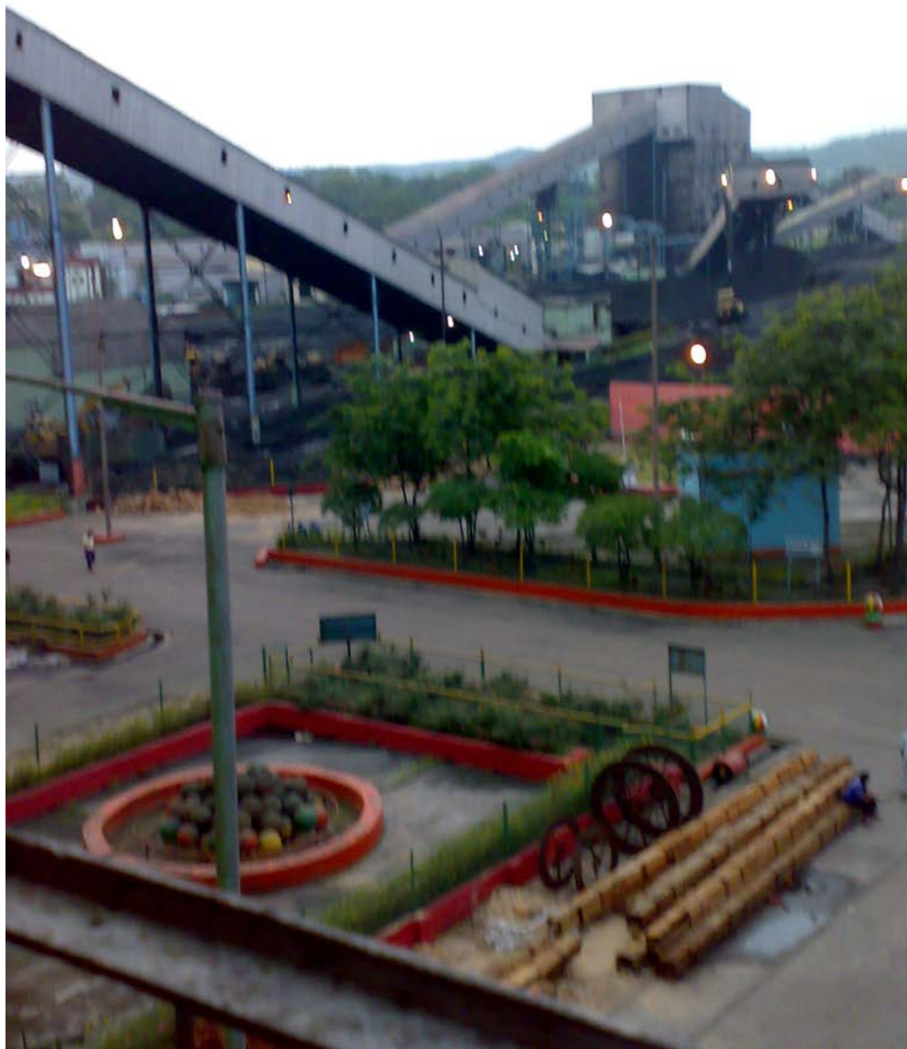
A Typical Coal Handling Plant
