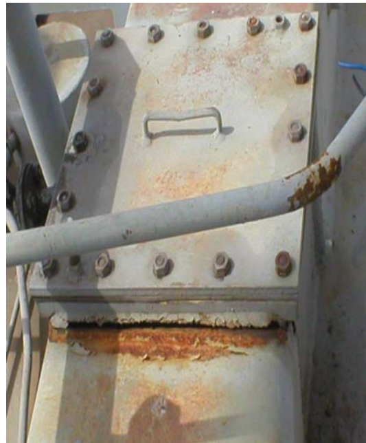
Exhibit-6 Lifted inspection window
