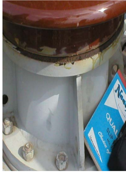
Exhibit-4 Displacement of bushing from cemented portion
