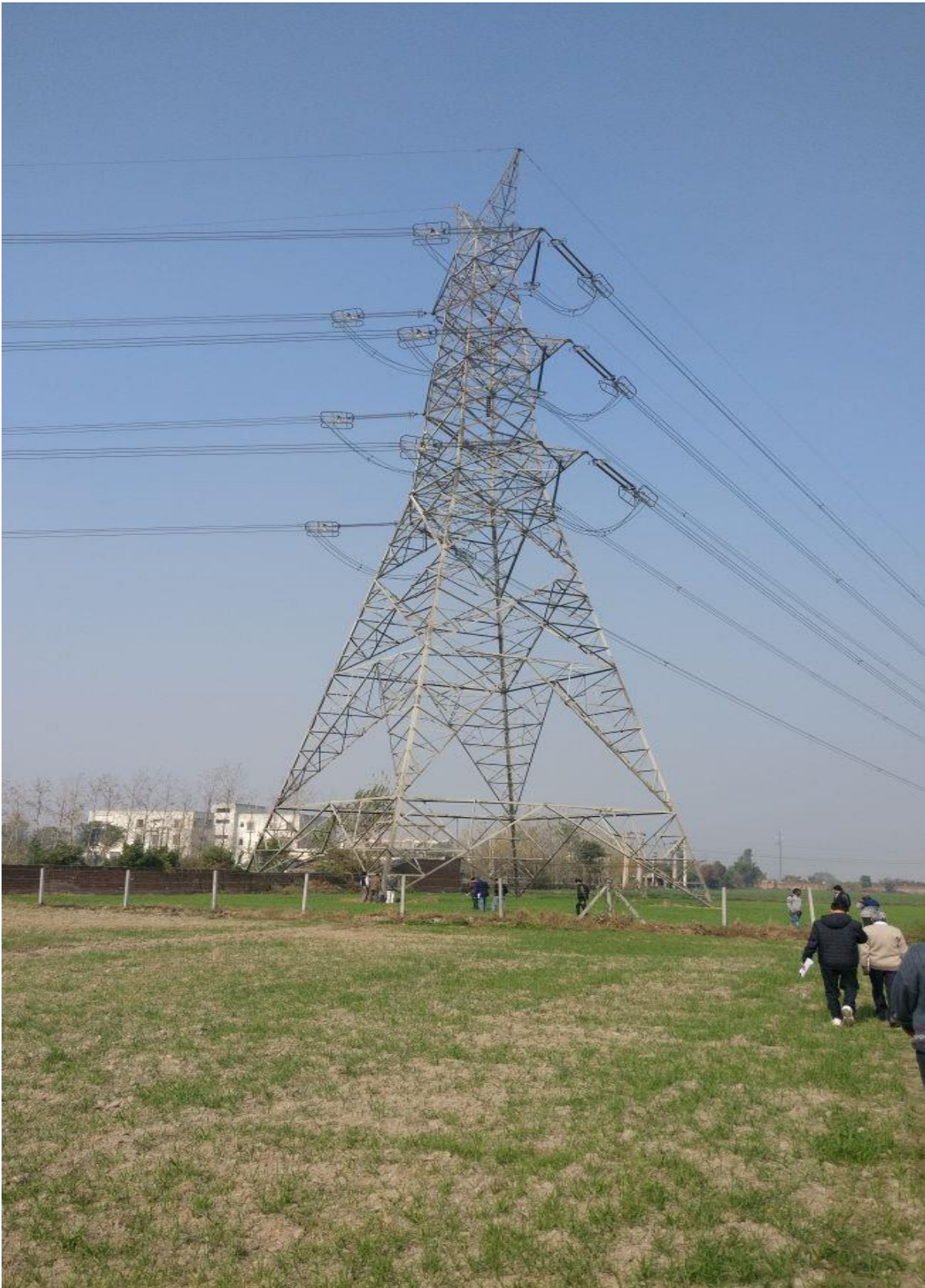
Fig. 1.2. Larger view of the tower for inspecting verticality
