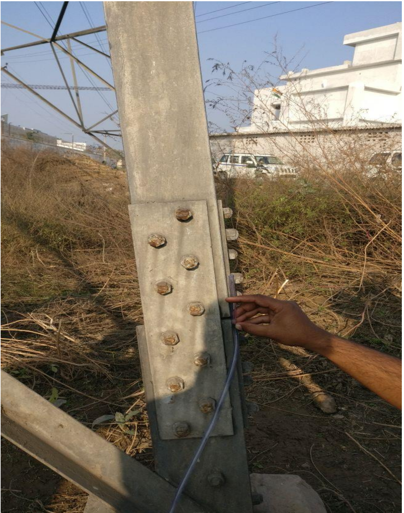
Fig. 2.1. Measurement of differential settlement of tower
