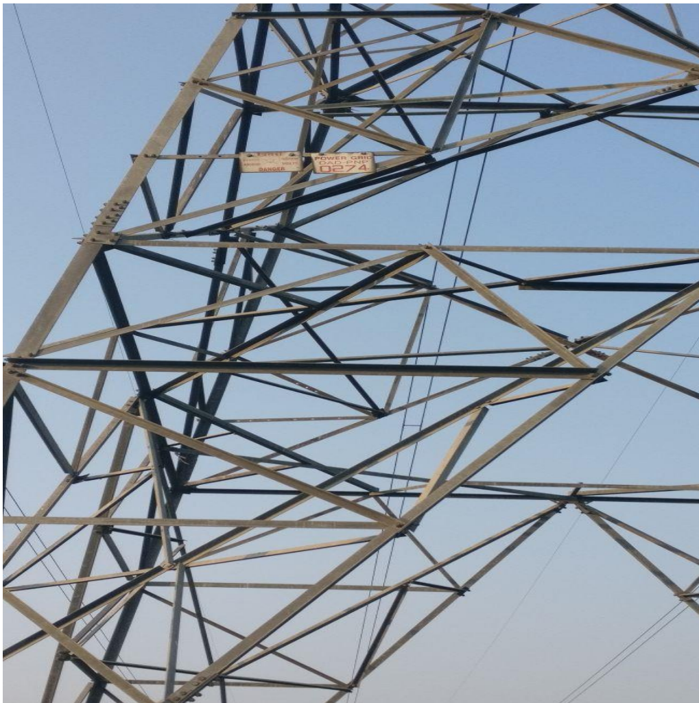
Fig. 3.1. Visual inspection of towers by binoculars
