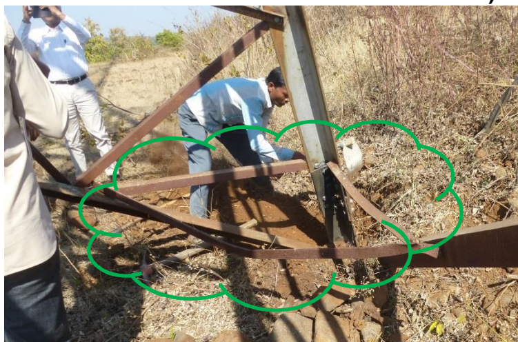
Fig. 2 Tower-1 Audited on 16/01/2019
