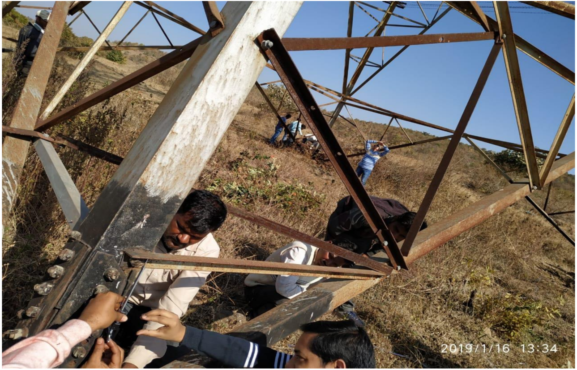
Figure 3. Corroded Members
