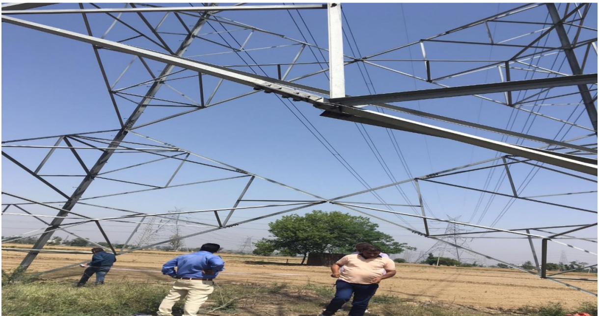
Figure 5. Measurement of base width
