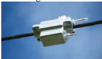
Fig1: DLR Sensor, Source: Ampacimon
