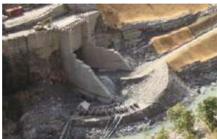
Pumps installed for HRT filling at Spill tunnel portal
