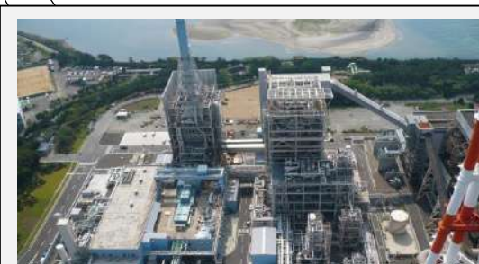
Joban Joint Power Co. Nakoso #10, 250MW (Demo. 2007 -, Commercial 2013 -)
