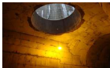
Orifice as seen from Surge shaft Bottom
