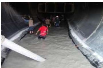
Cleaning of pressure shaft
