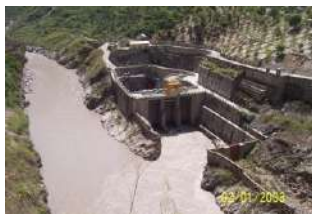
Picture 3 : (TRT Out-Fall, Nathpa-Jhakri HEP)
