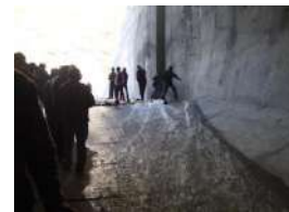
View from Spill tunnel
