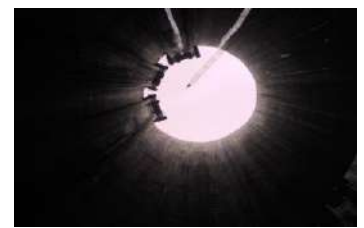
Surge Shaft viewed from orifice slab
