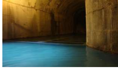
Surge shaft bottom and rock trap seen in upstream
