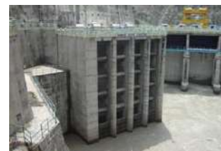
Picture 4 : (Intake Structure, Rampur HEP)
