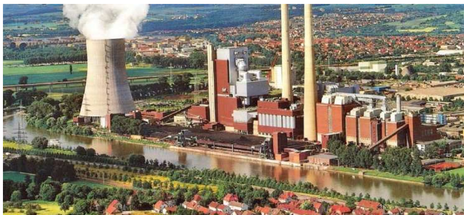
Figure 17: EnBW Energie Heilbronn PP
