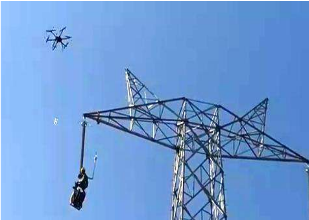
UAV dropping the guide wire on the tower.
