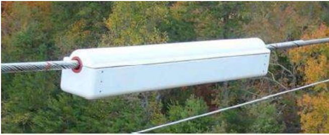
Figure 5: Series FACTS device clipped on Transmission Line Source: Ref [2]
