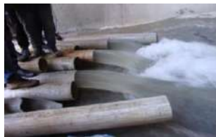
Start of flushing operation
