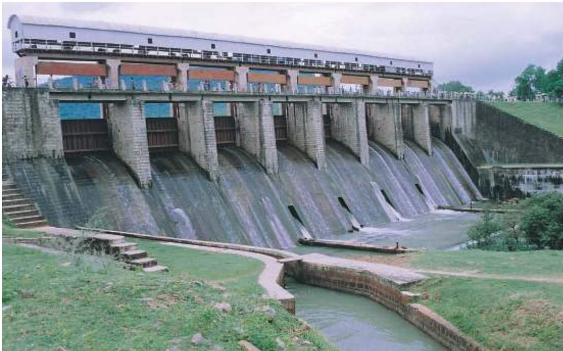
Kohima Dam Pumped Storage Project (3x38 MW), Distt. Kamur
