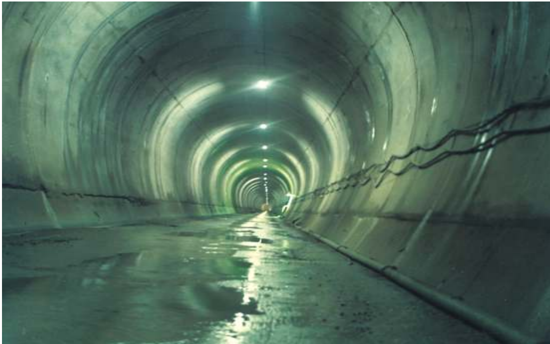
Head Race Tunnel Under Construction.
