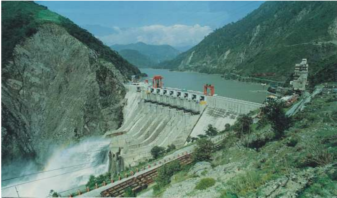
Chamera Hydro Power Station, Stage-I, 540 M (HP) Dam
