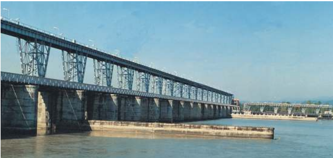
120 MW Tanakpur Power Station (Uttaranchal) - Barrage
