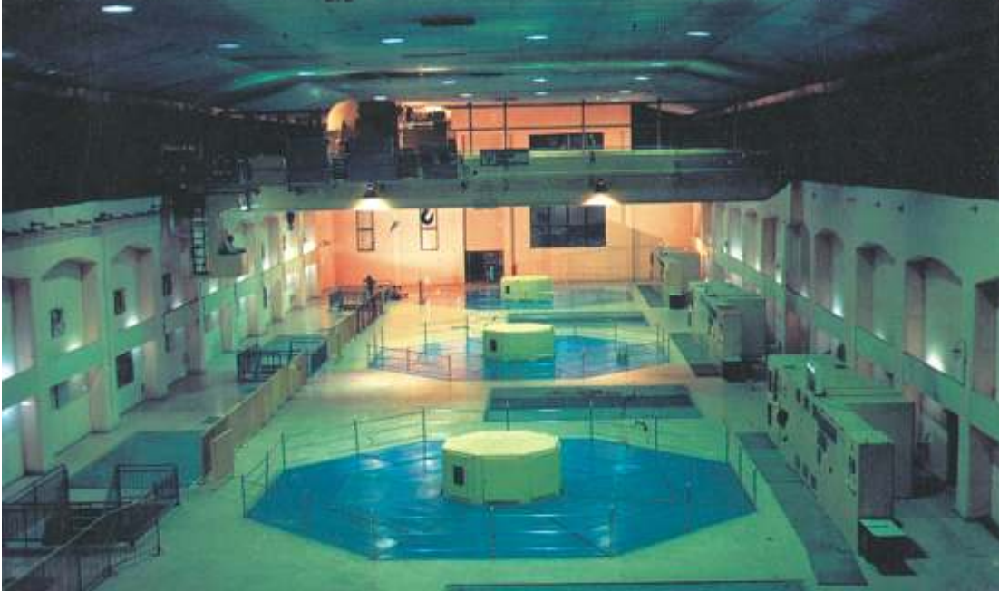
Chamera Hydro Electric Project Stage-I, 540 MW (H.P.)
