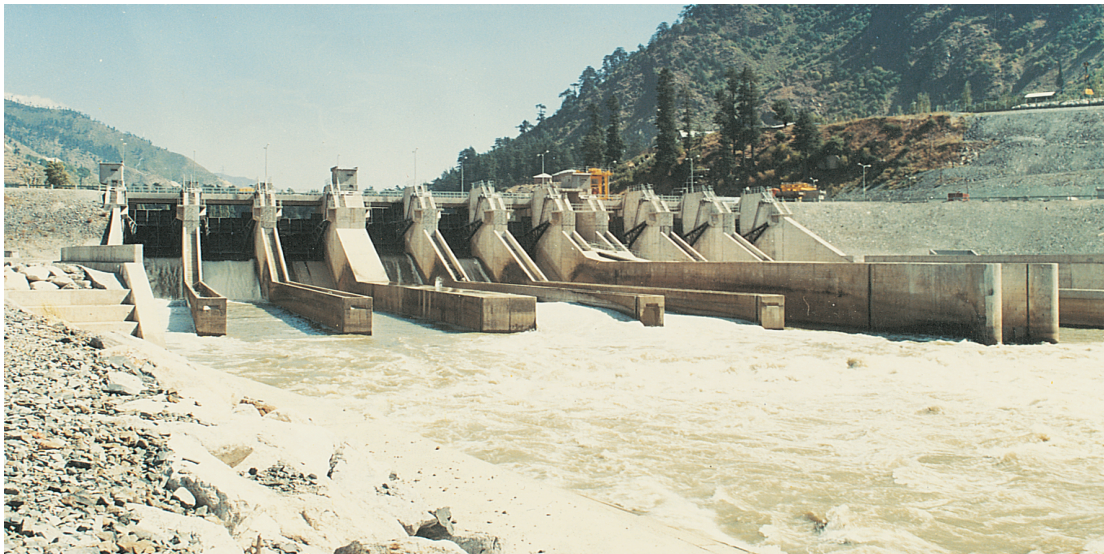
Barrage of Uri Hydro Power Station - 480 MW (J&K)
