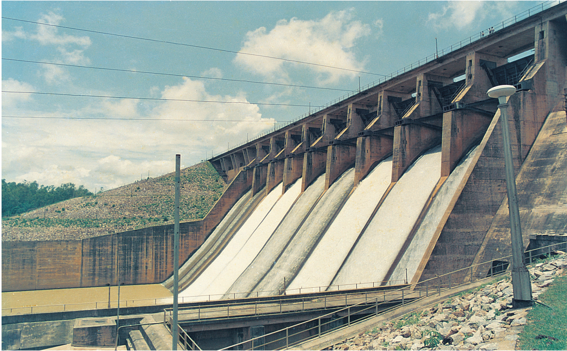
Tilaiya Dam-Damodar Valley Corporation.
