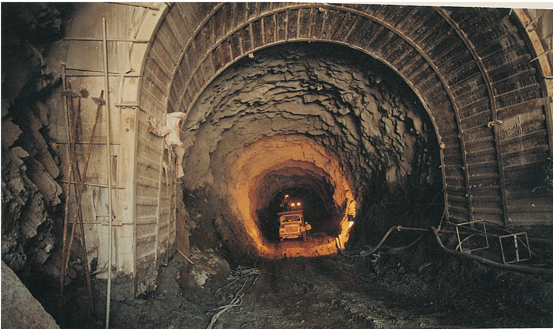
510 MW Teesta Stage-V Project (Sikkim)-Tail Race Tunnel Under Construction.
