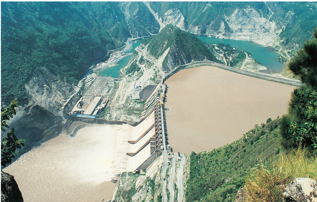
Salal Power Station, 345 MW (J&K) Dam
