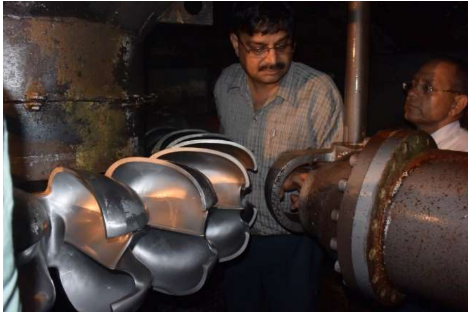
Inspection of Pelton Turbine
