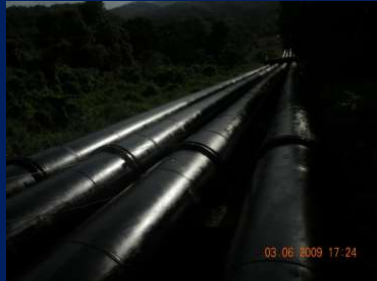
Penstocks under process of painting
