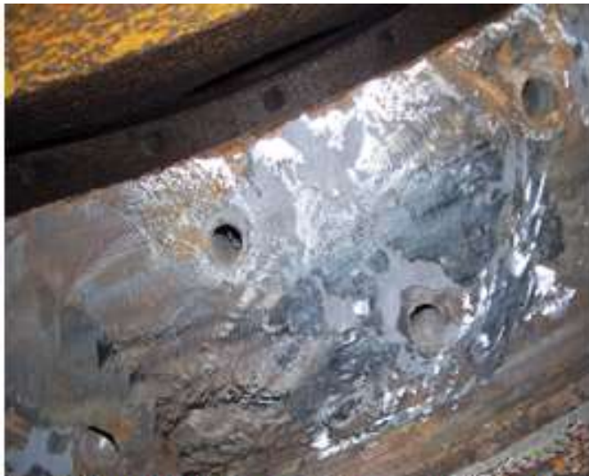
After Welding and Manual Grinding
