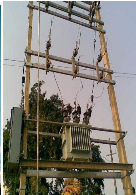
Figure-1(b) Three phase Pole Mounted DT substation (H pole)
