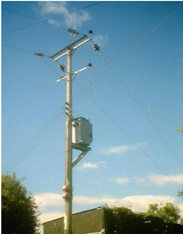
Figure-1(a) Single phase Pole Mounted DT substation
