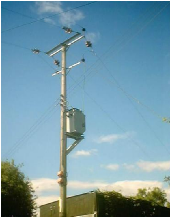
Figure-1(a) Single phase Pole Mounted DT substation
