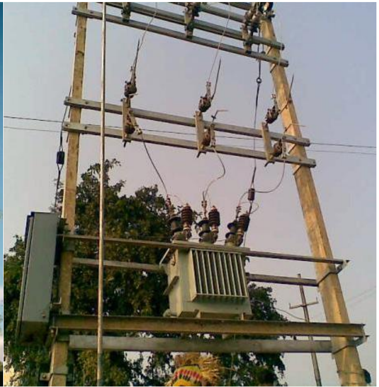
Figure-1(b) Three phase-Pole Mounted DT substation (Hole)
