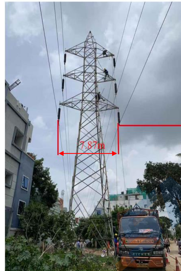
Before replacing the CICA
