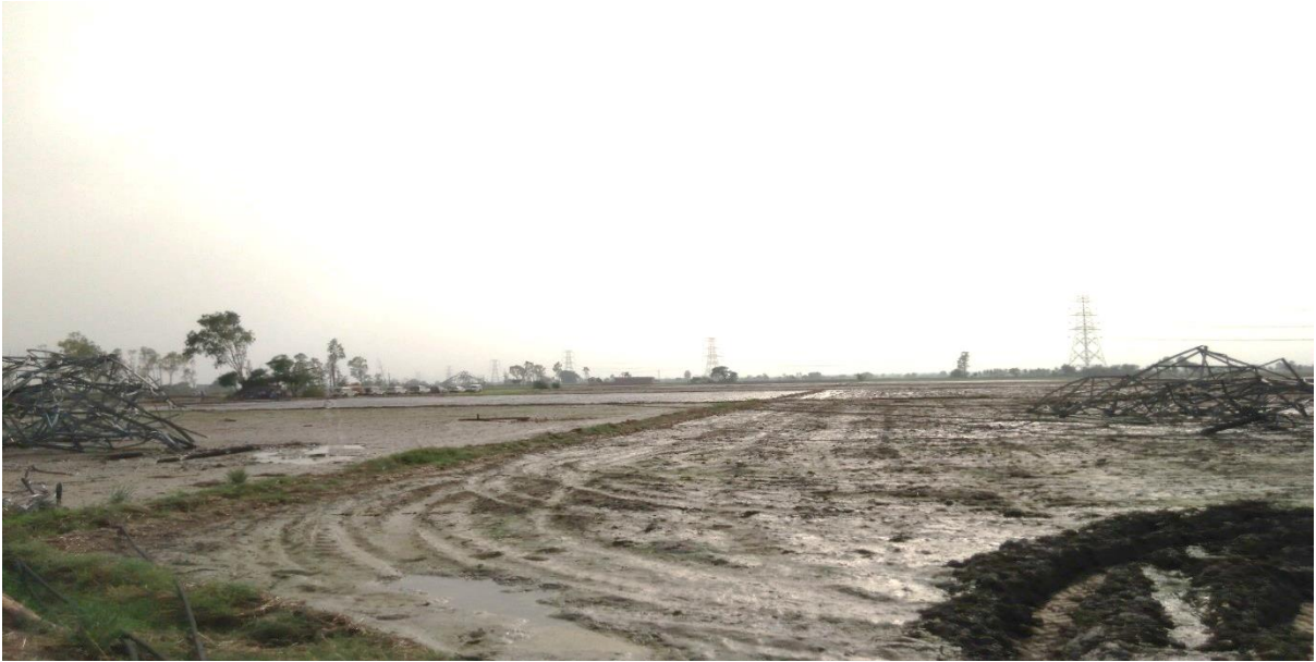
Tower at Loc. No. 57
