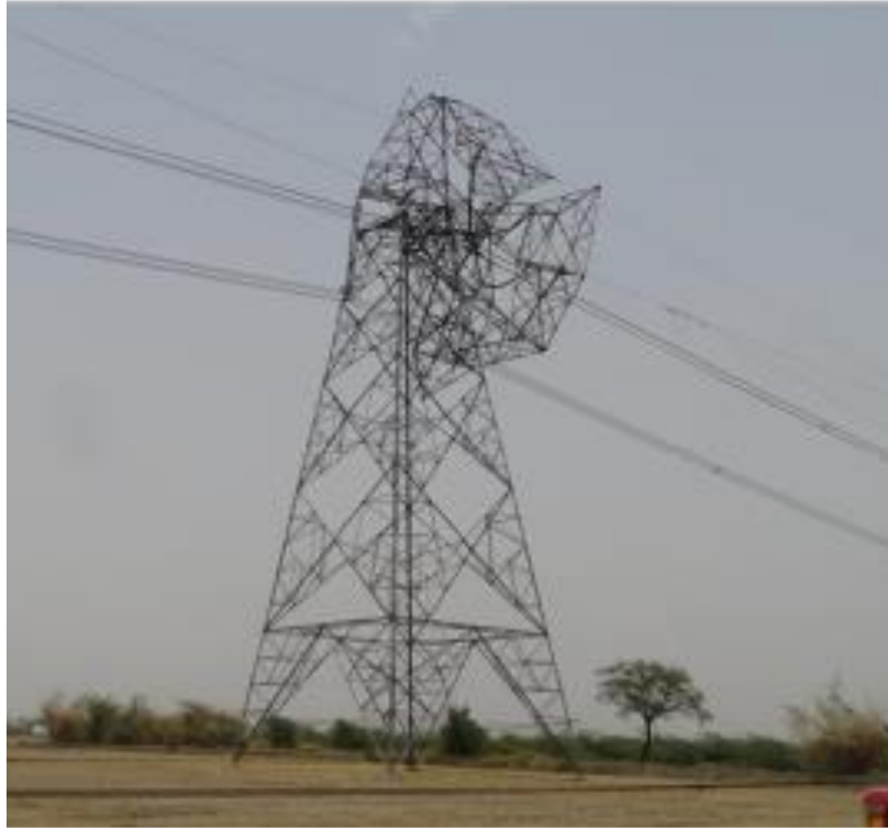
Tower at Loc. No. 17 (A+0)
