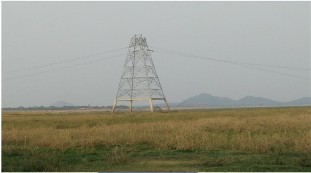
Tower at Loc. No. 63
