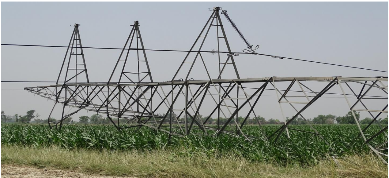
Tower at Loc. No. 272
