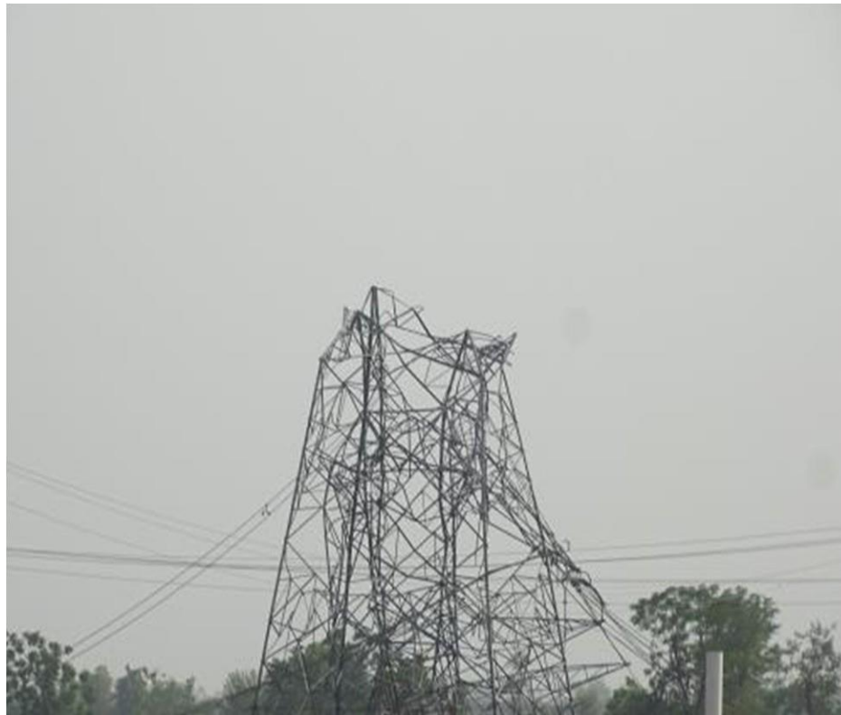
Tower at Loc. No. 61
