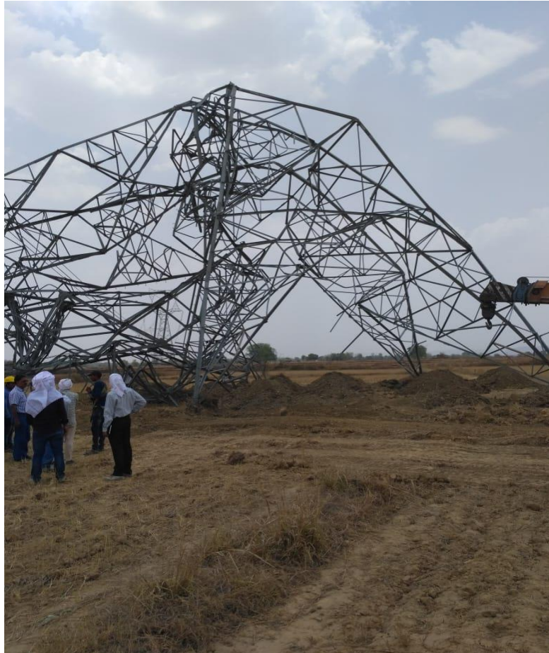
Tower at Loc. No. 63(A+0)
