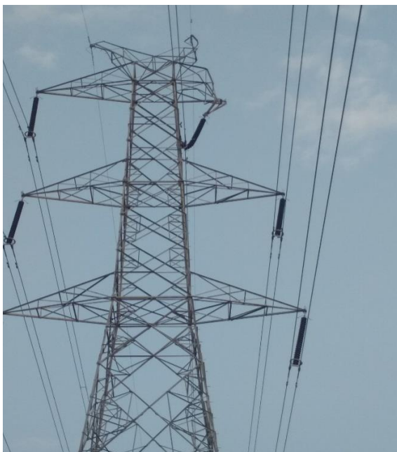
Tower at Loc. No. 37
