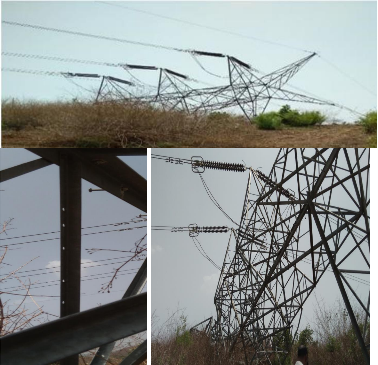
Tower at Loc. No. 219
