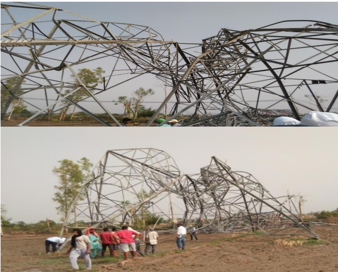
Tower at Loc. No.58
