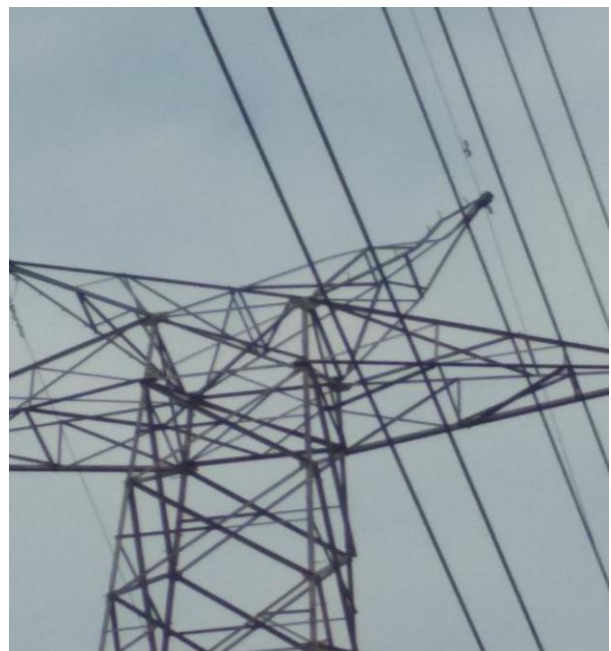
Tower at Loc. No. 38
