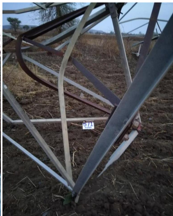
Tower at Loc. No. 571
