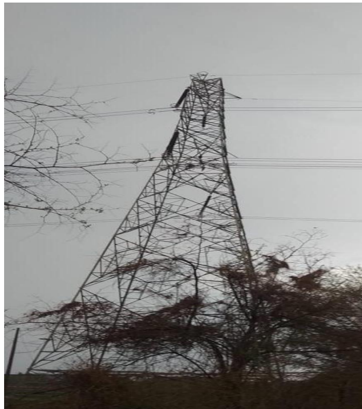
Tower at Loc. No. 574
