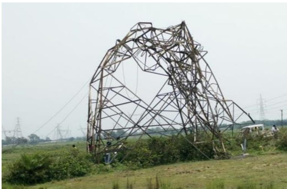
Tower at Loc. No. 377 (A+0)
