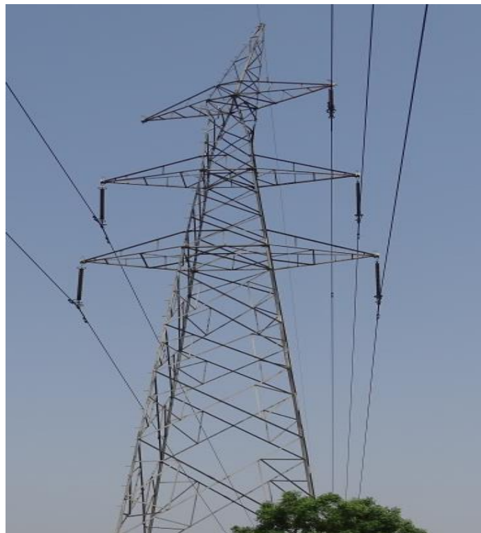
Tower at Loc. No. 268
