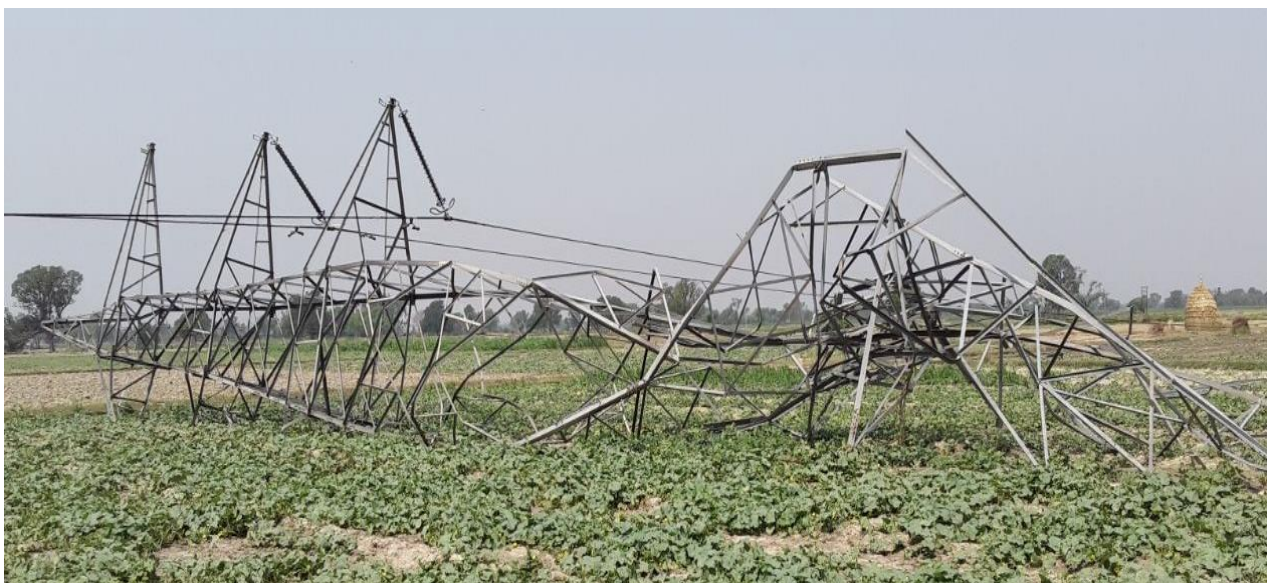
Tower at Loc. No. 270
