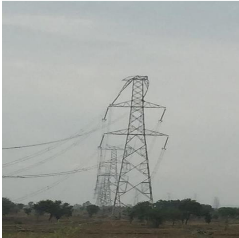
Tower at Loc. No. 569
