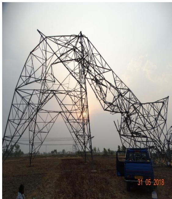
Tower at Loc. No. 185
