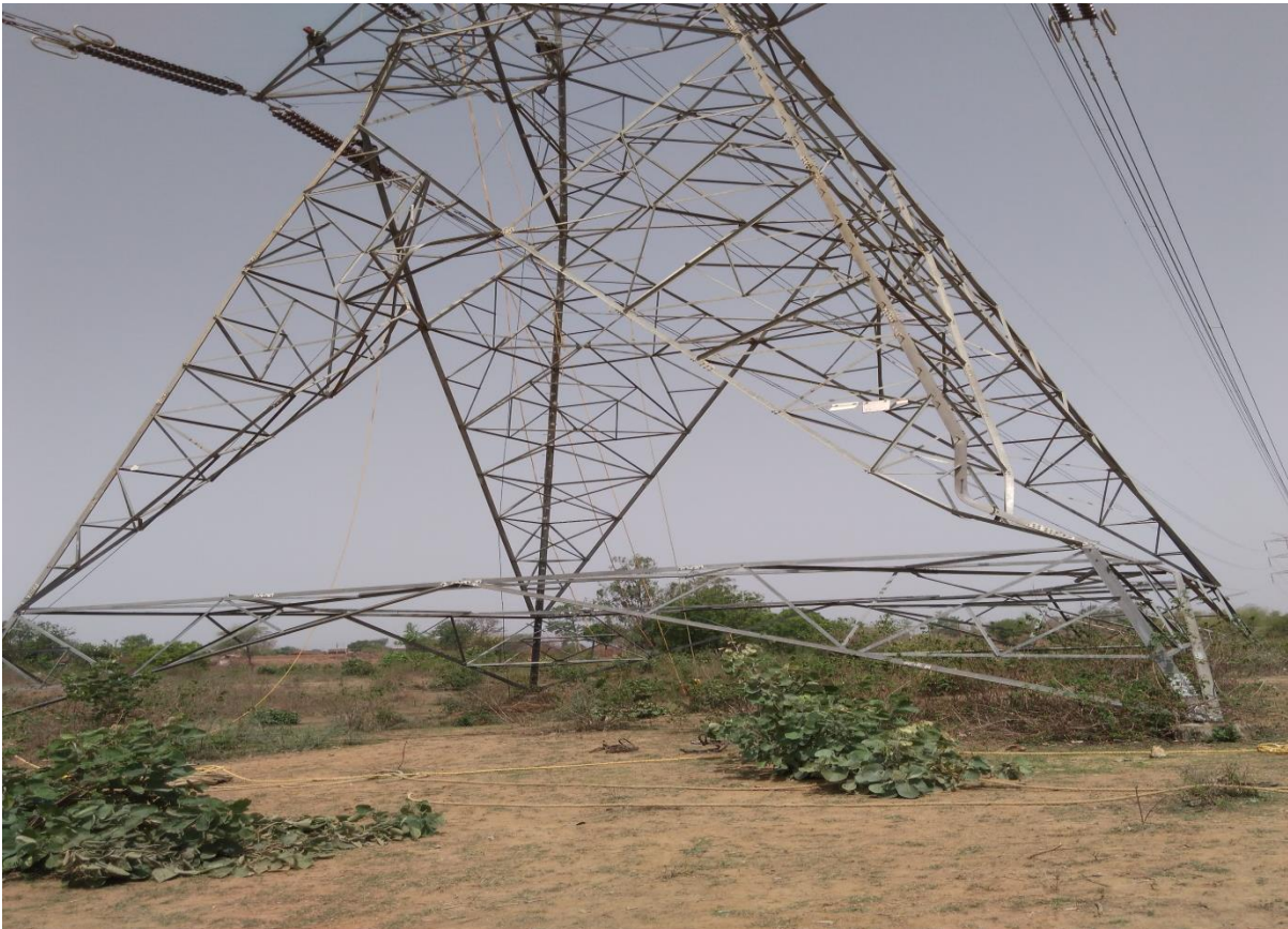
Tower at Loc. No. 220
