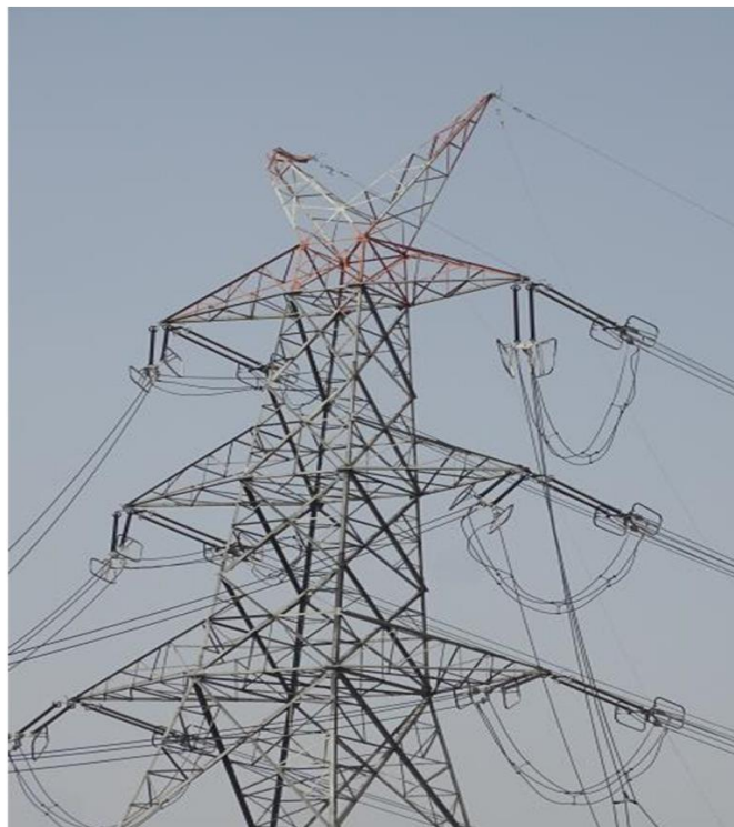
Tower at Loc. No. 54
