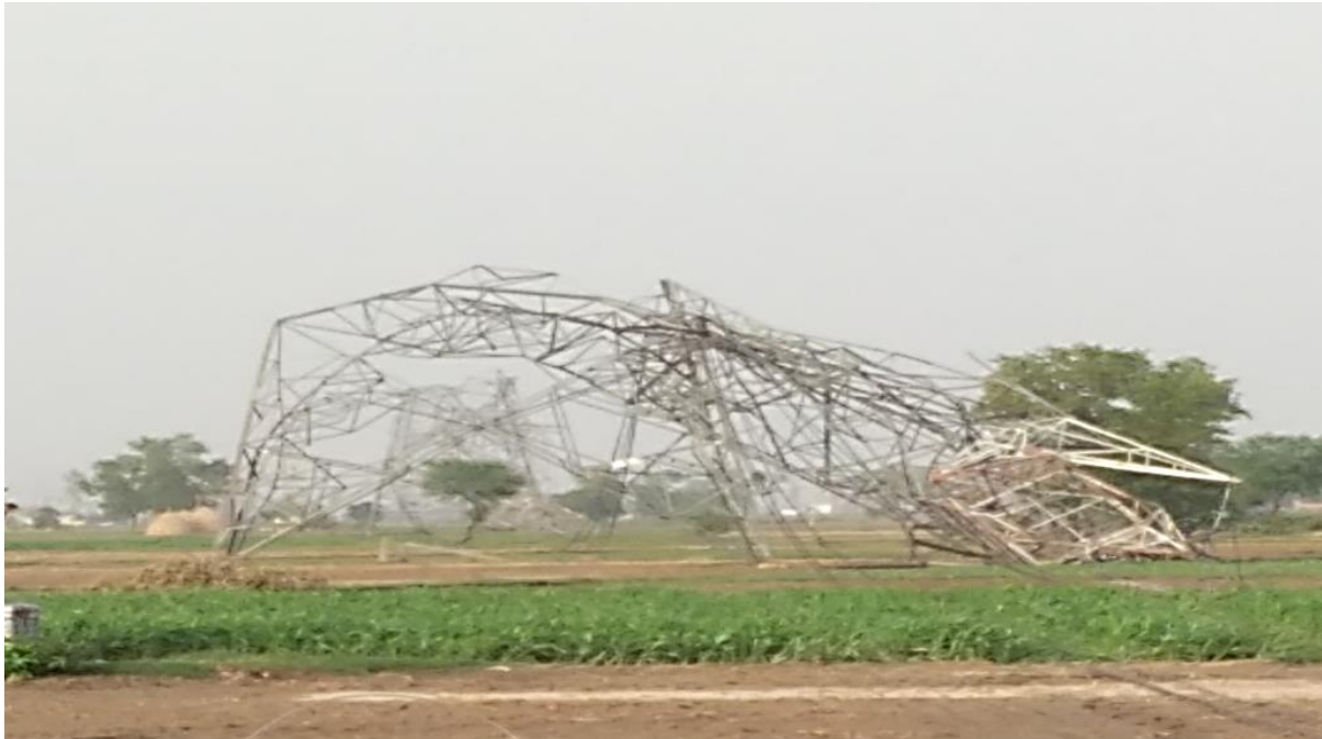
Tower at Loc. No. 62
