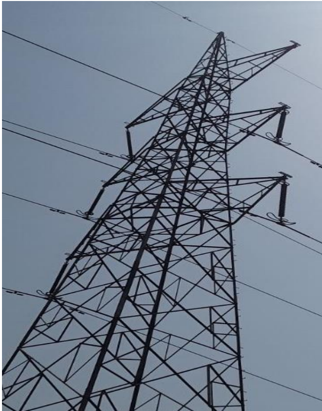
Tower at Loc. No. 266
