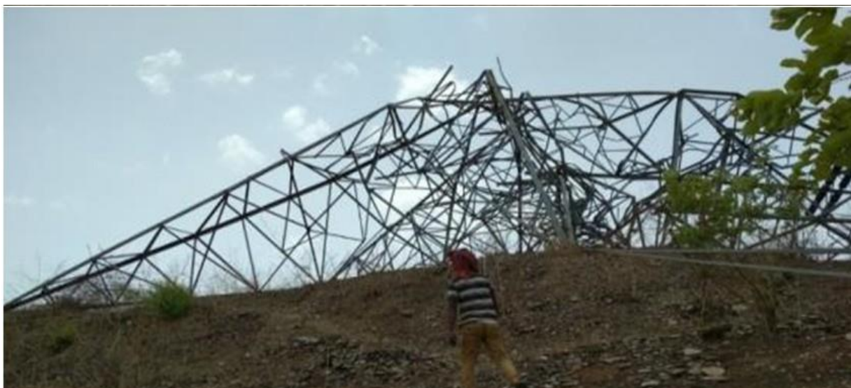
Tower at Loc. No. 218
