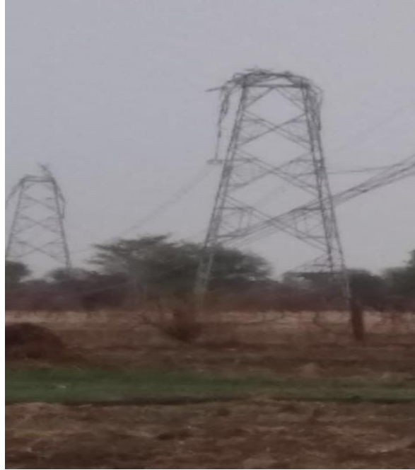
Tower at Loc. No. 573
