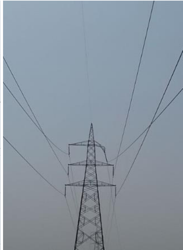
Tower at Loc. No. 267
