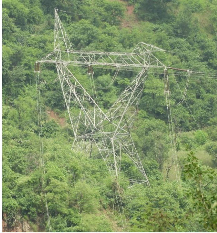
Tower at Loc. No. 239
