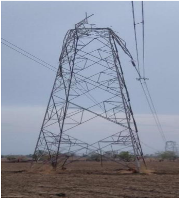
Tower at Loc. No. 572
