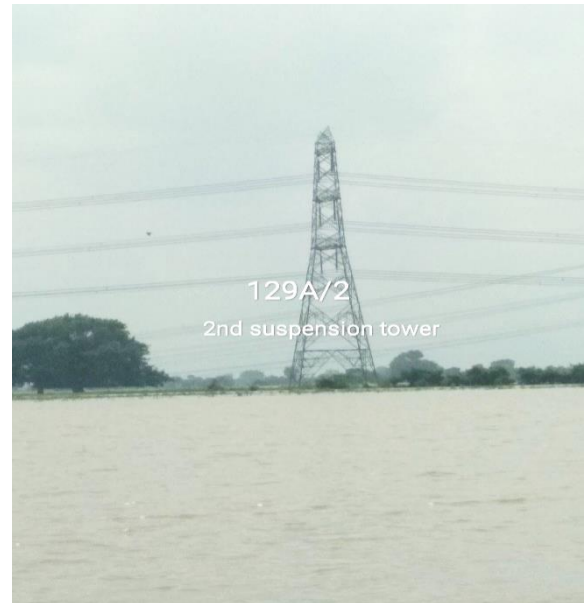
Tower at Loc. No. 129A/2
