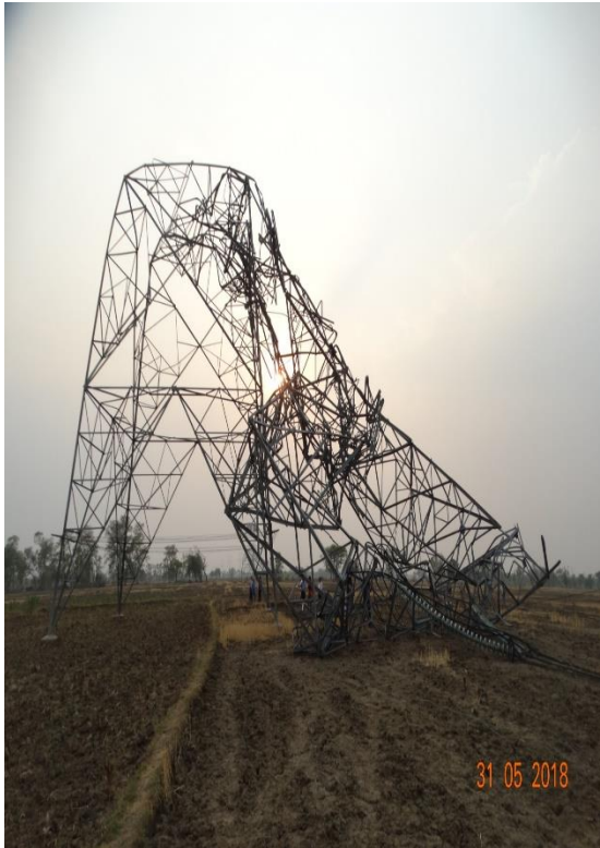
Tower at Loc. No. 184
