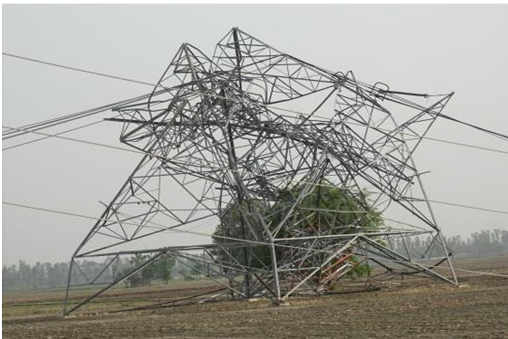
Tower at Loc. No. 60
