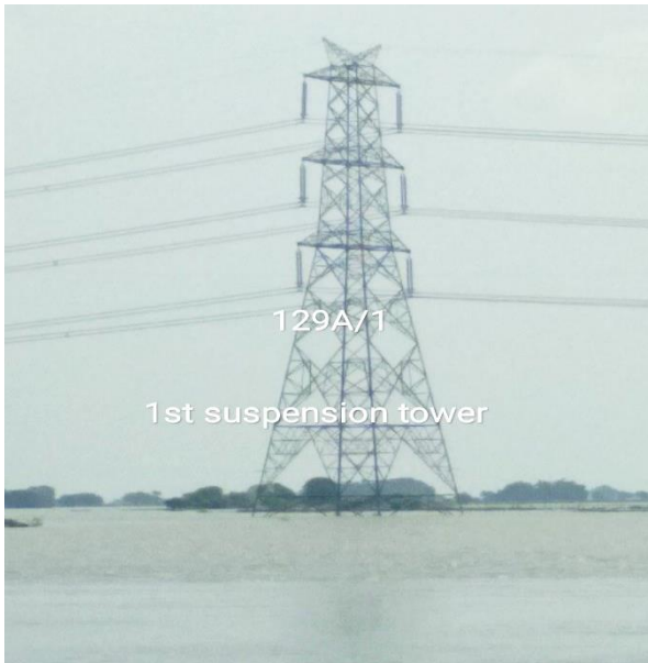
Tower at Loc. No. 129A/1
