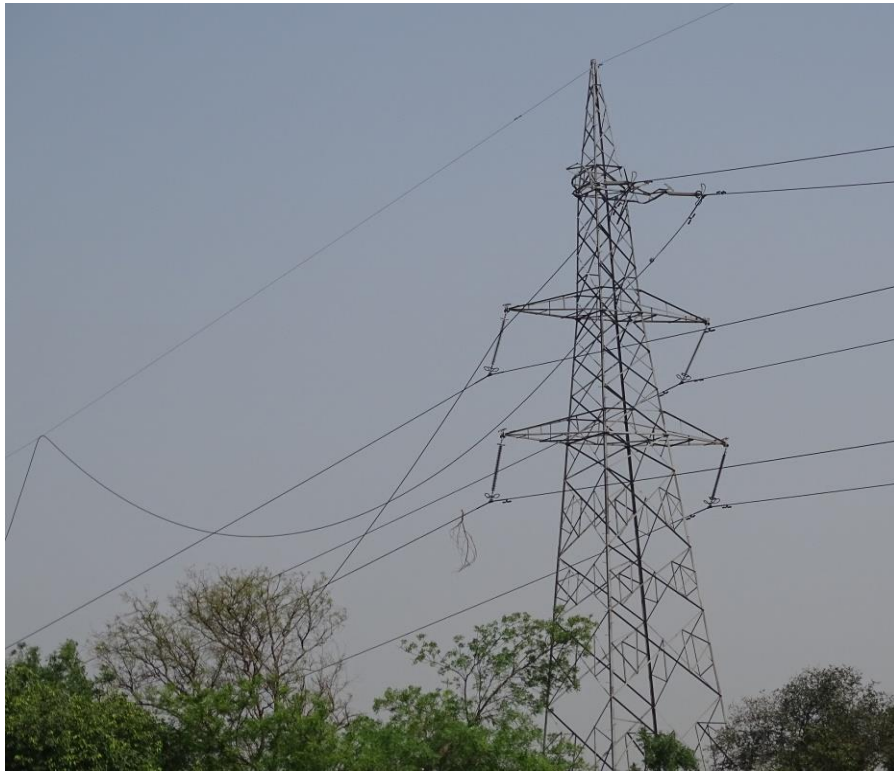
Tower at Loc. No. 269
