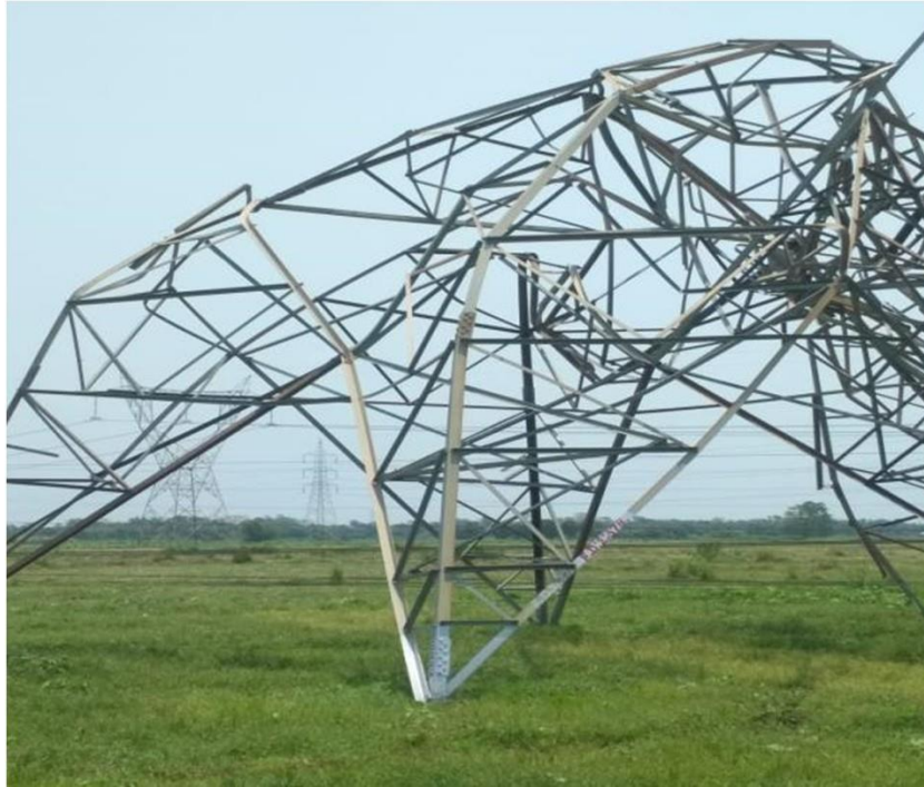
Tower at Loc. No. 378 (A+0)
