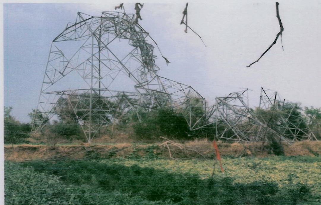
Tower at Loc. No. 122
