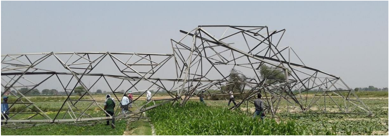
Tower at Loc. No. 271
