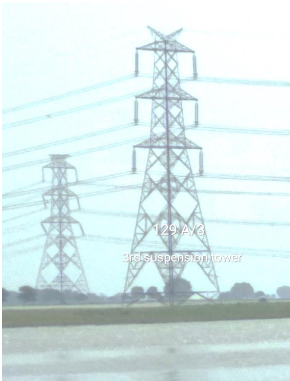
Tower at Loc. No. 129A/3
