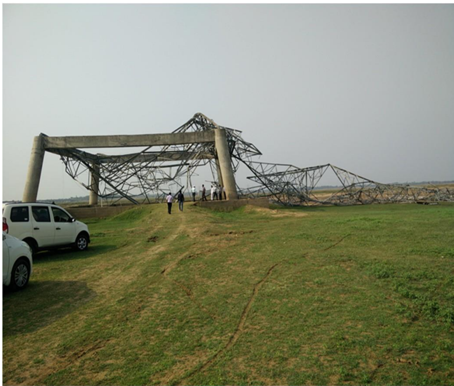
Tower at Loc. No. 64
