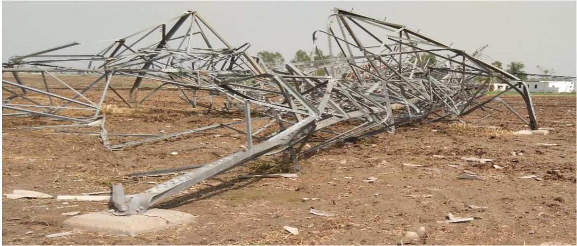
Tower at Loc. No. 55
