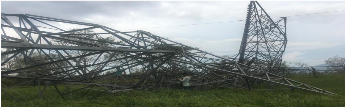
Tower at location no 952 (DA+3)
