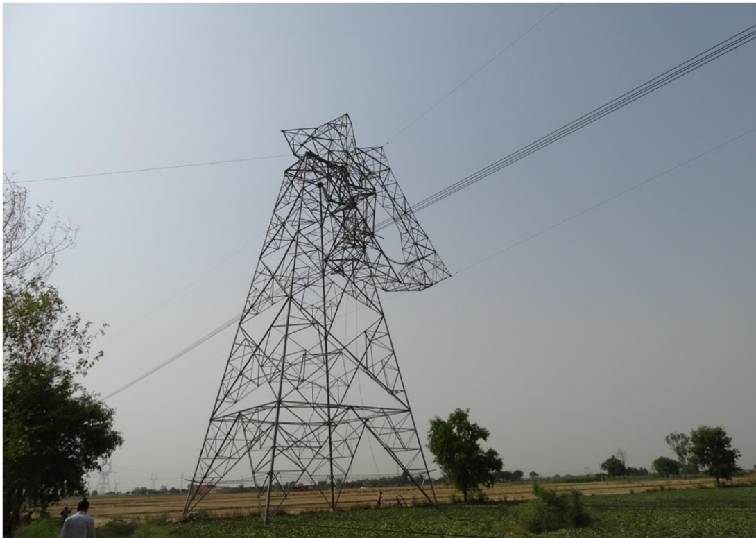
Tower at Loc. No 568 (A+0)
