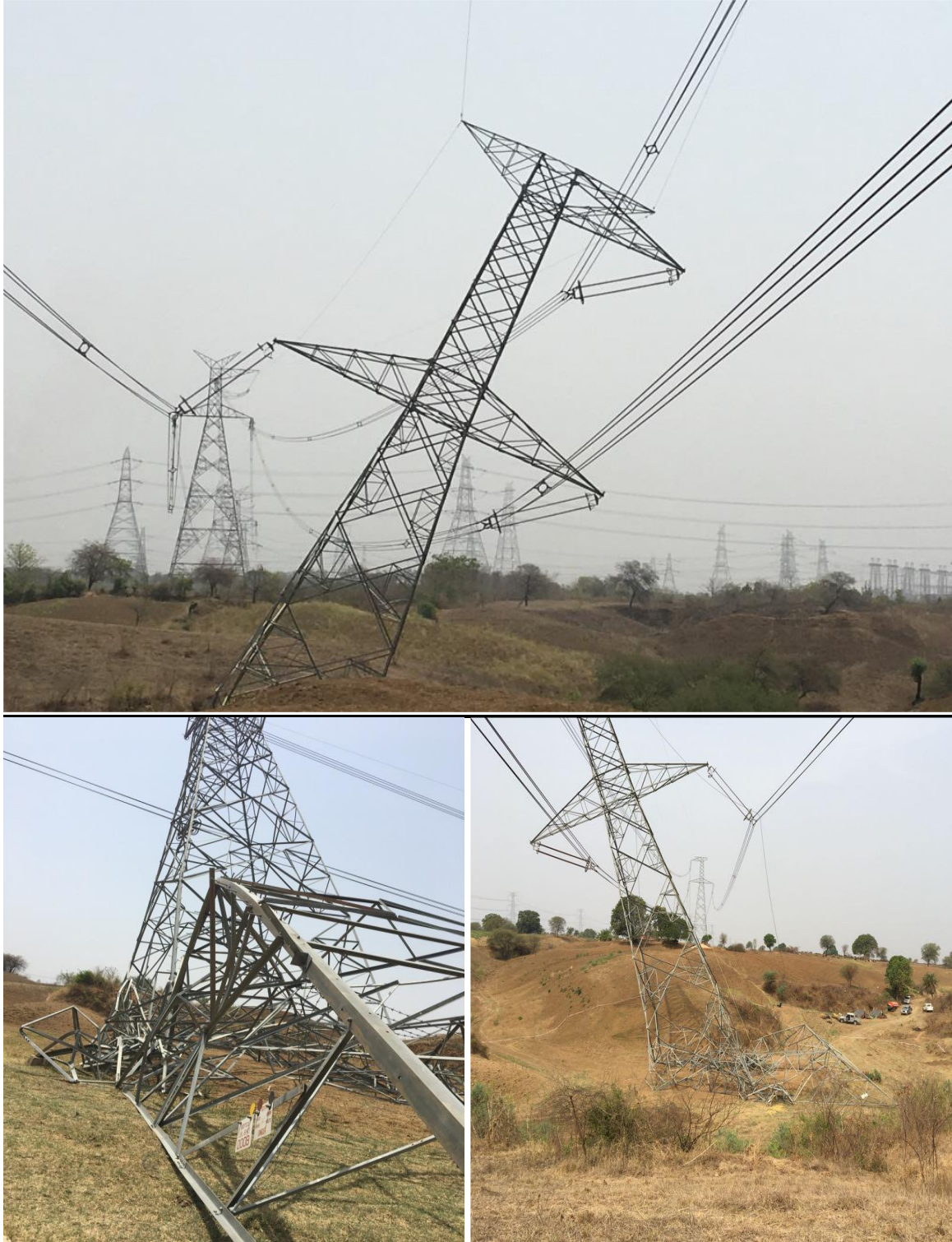
Tower at location no 2A/3
