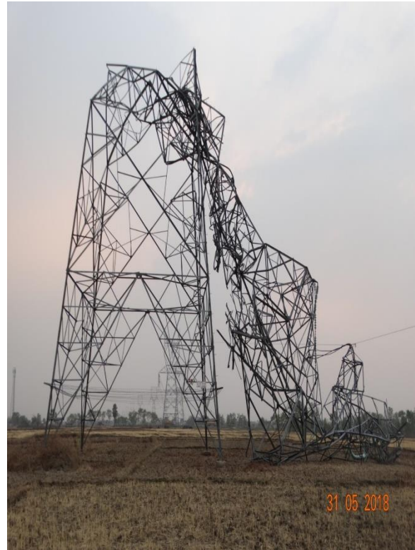
Tower at Loc. No. 186
