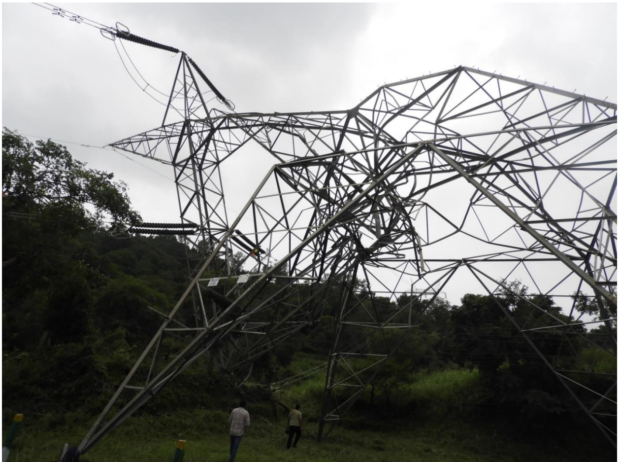
Tower at Loc. No. 238
