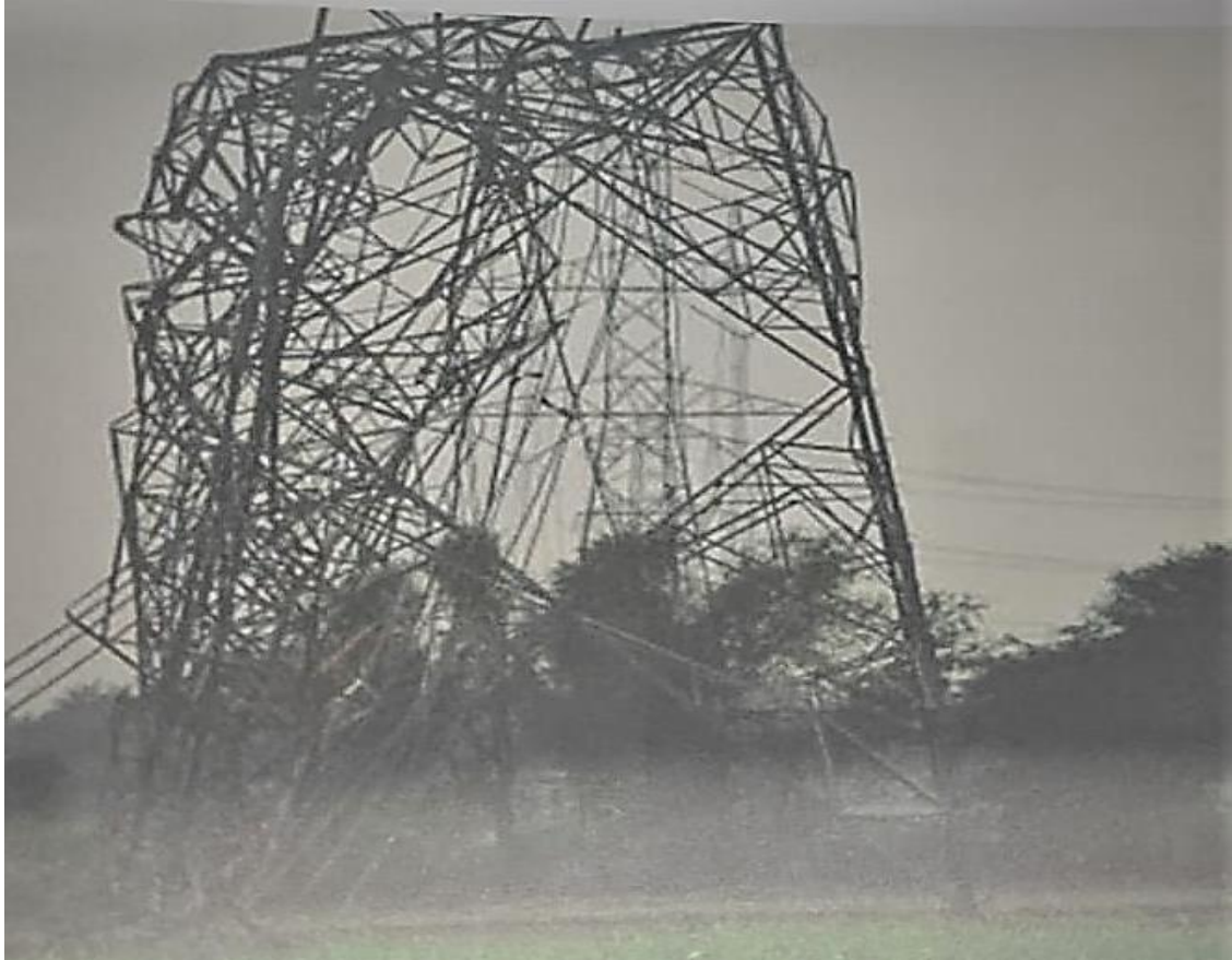
Tower at Loc. No. 63
