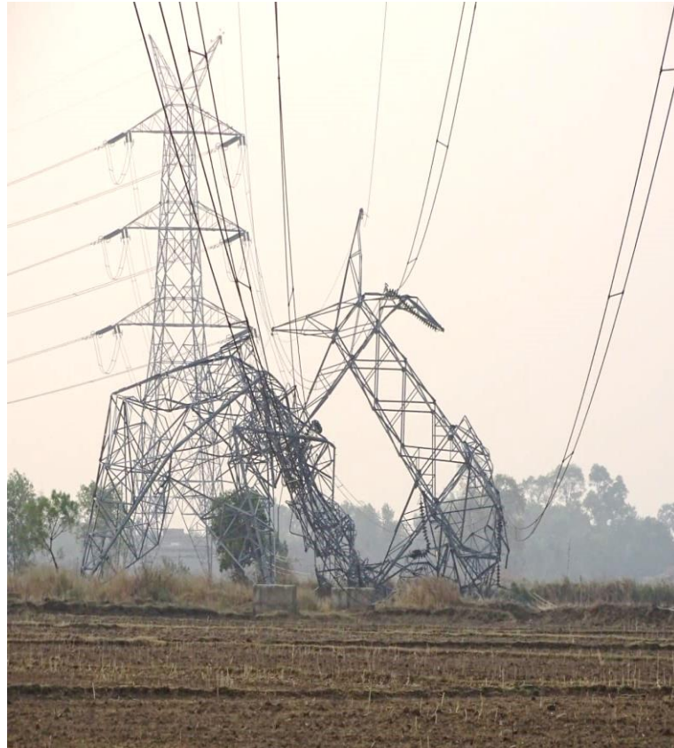
Tower at Loc. No. 36
