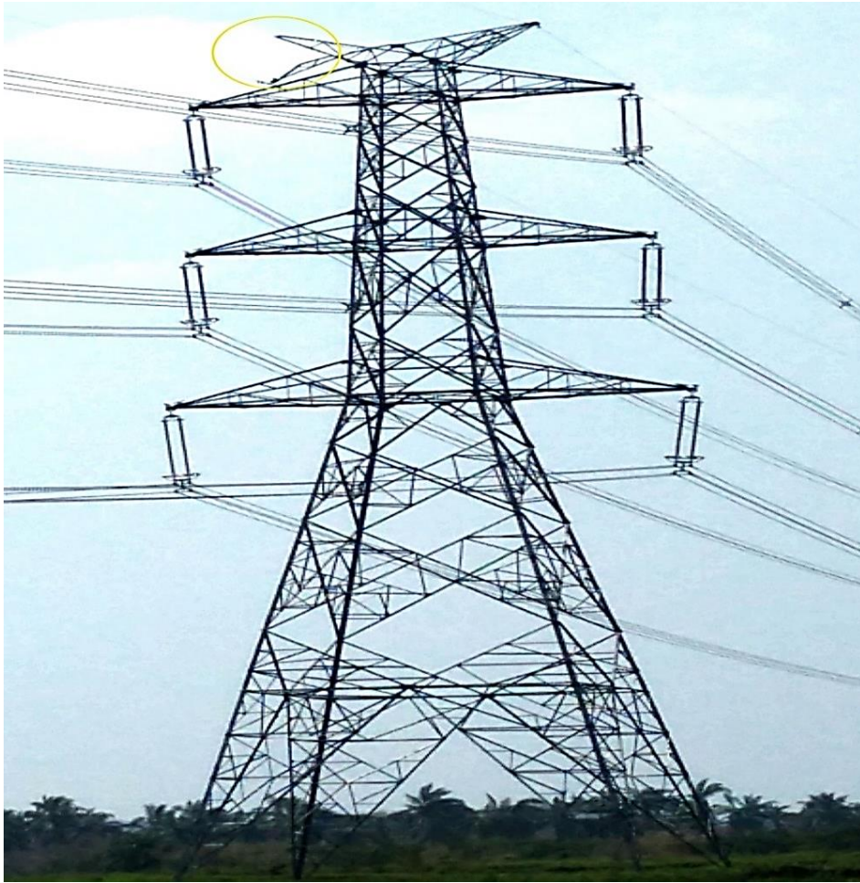
Tower at location no. 15/2
