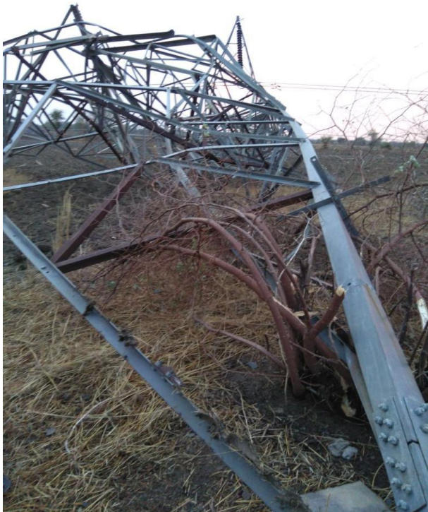
Tower at Loc. No. 570
