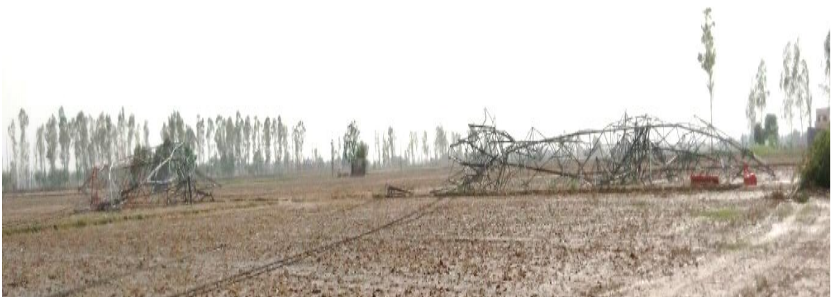
Tower at Loc. No. 56
