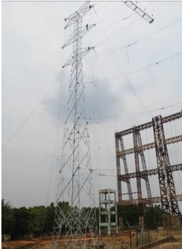
230 kV D/C Suspension tower
