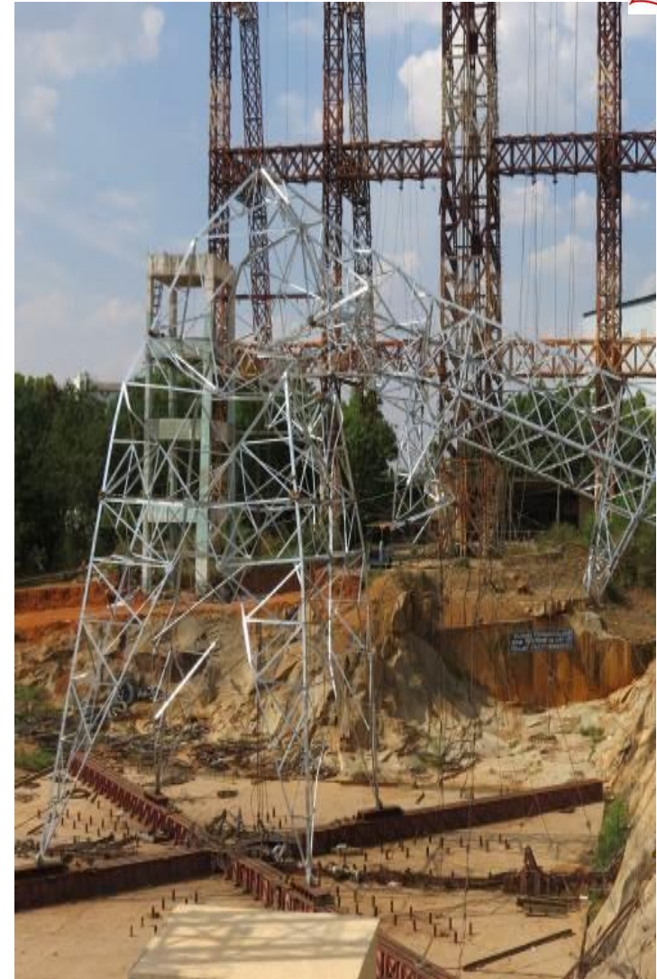
Failed during waiting period at 100 % loads
