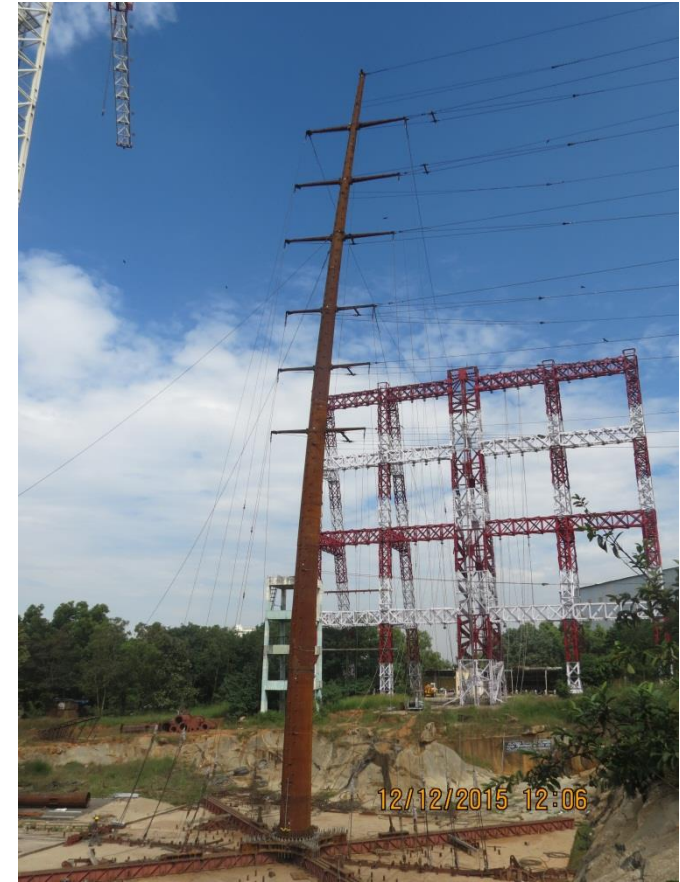
220/132 kV M/C Steel pole, MPPTCL Jabalpur First time in India
