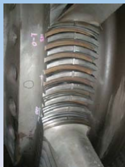
Blade groove after removing blades
