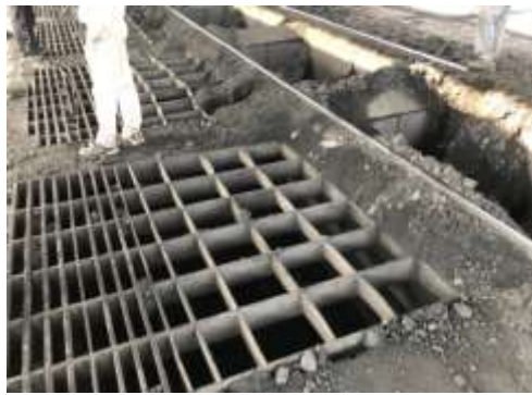
Underground pit for coal delivery
