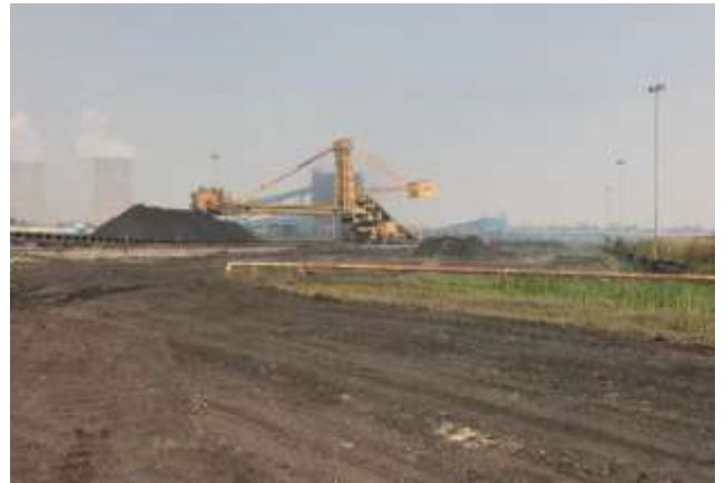
Coal storage area
