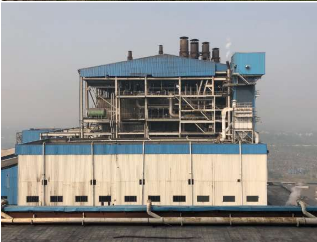
Figure 1-1 Full view of the power plant and boiler building (photo taken by the survey team)
