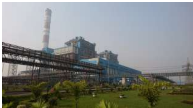
DVC Durgapur Steel power plant
