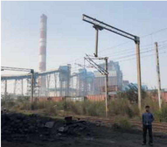
Full view of the power plant
