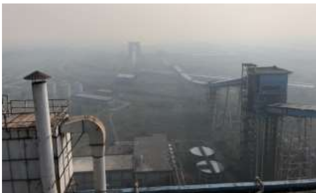
Coal conveyor from the coal storage area
