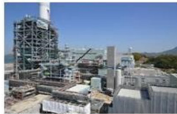
Osaki CoolGen (Construction underway)
