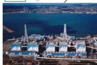
Chubu Electric Power's Hekinan Power Station (Unit 4 and 5 with MEEP)
