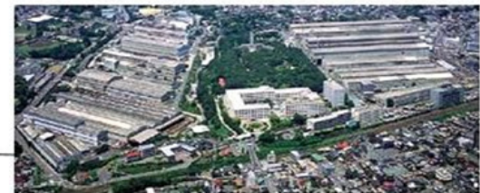
MHP's Hitachi Works
