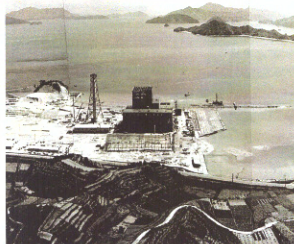
Construction view of No.1 Unit (using domestic coal) ··· Commencement of commercial operation in July 1967
