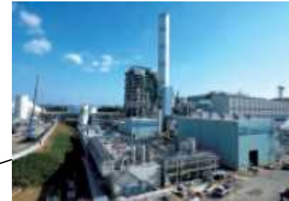
Demonstration plant for Oxy blown IGCC (Osaki CoolGen)
