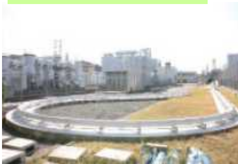
Test Facilities for Superconducting Cable
