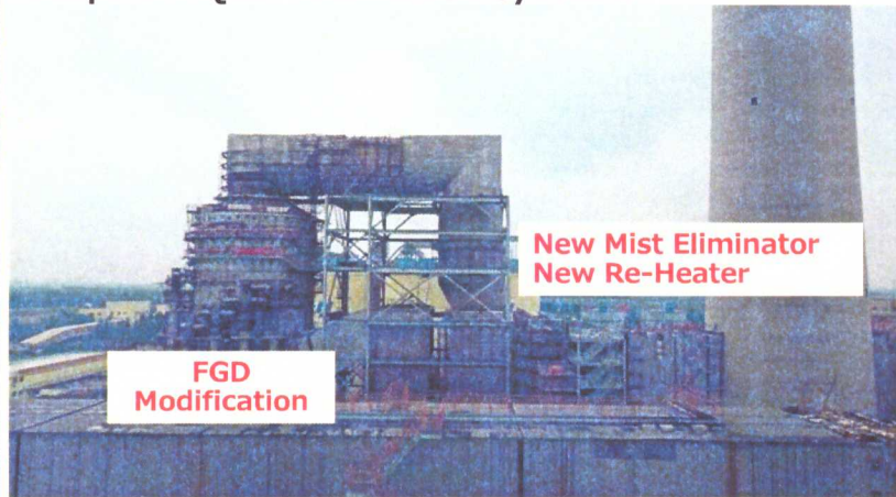
FGD Outlet After Upgrading
