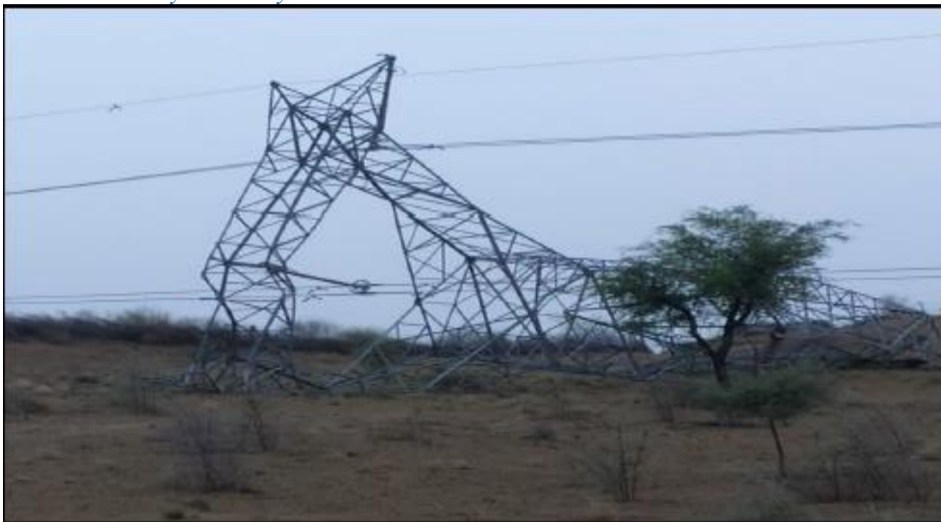
Fig 3(d). Tower at Location No.: 92 (A+0)
