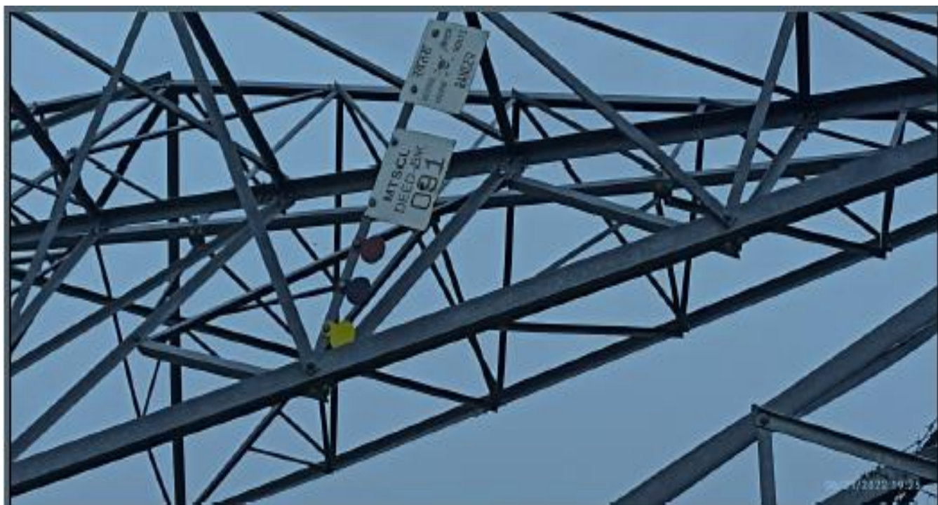
Fig 3(a). Tower at Location No.: 91 (A+3)
