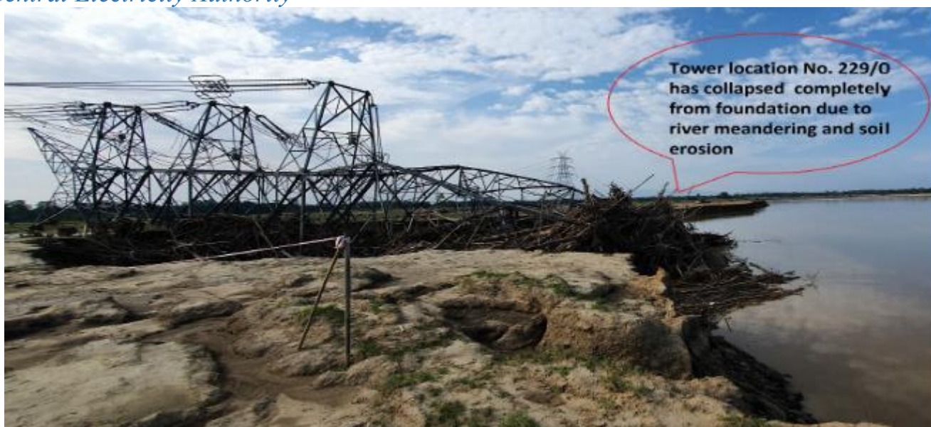
Fig 2(d). Tower at Location No.: 229/0 (DD+0)
