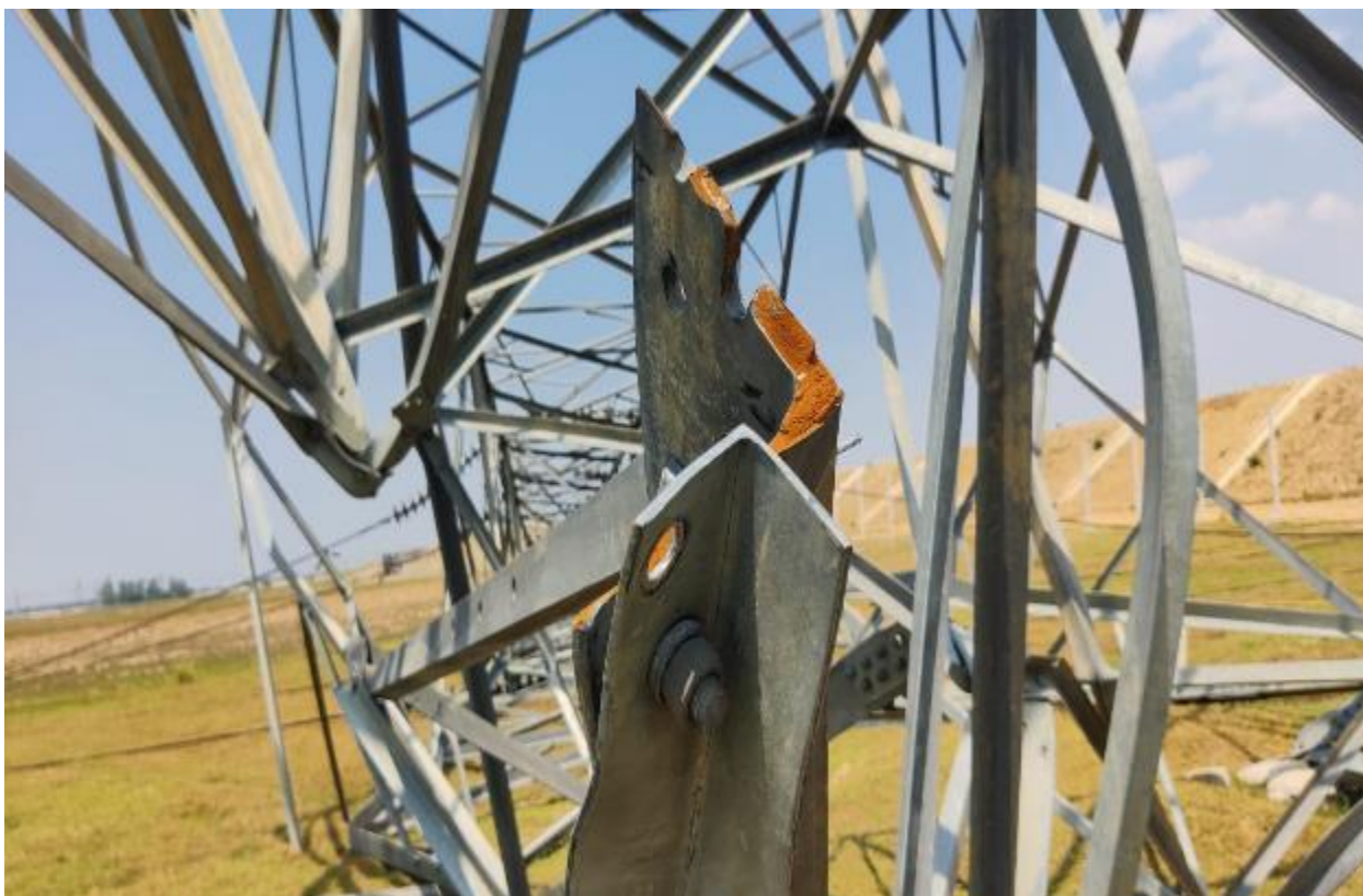
Tower no 59 stub:
