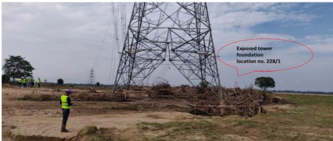
Fig 2(c). Tower at Location No.: 228/1 (DA+0)
