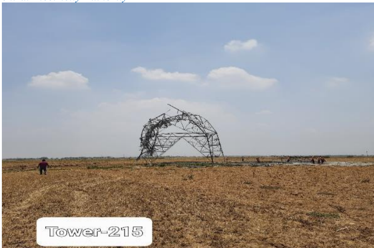
Fig.1(c). Tower at Location No.: 215 (DA+0)
