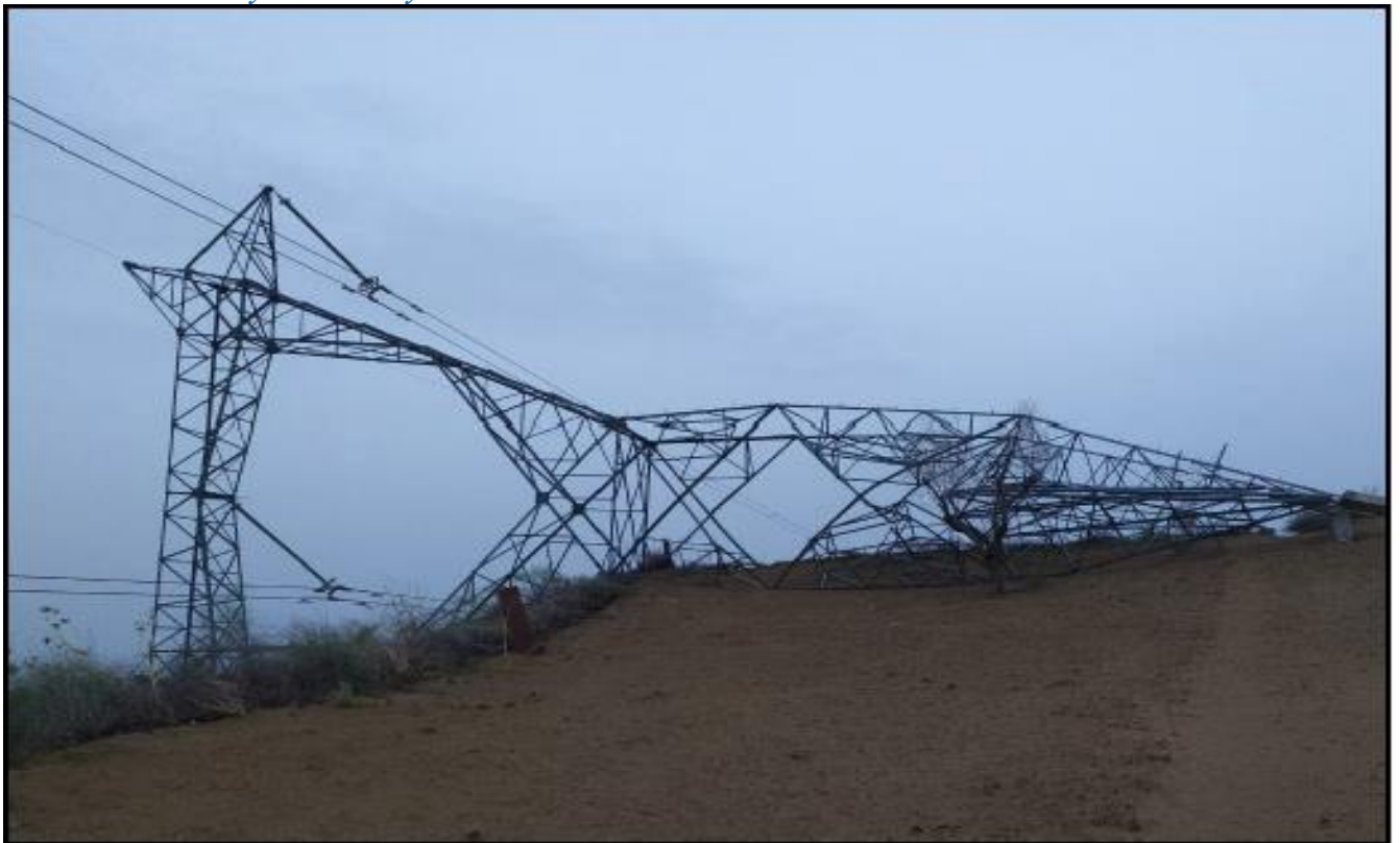
Fig 3(b). Tower at Location No.: 91 (A+3)
