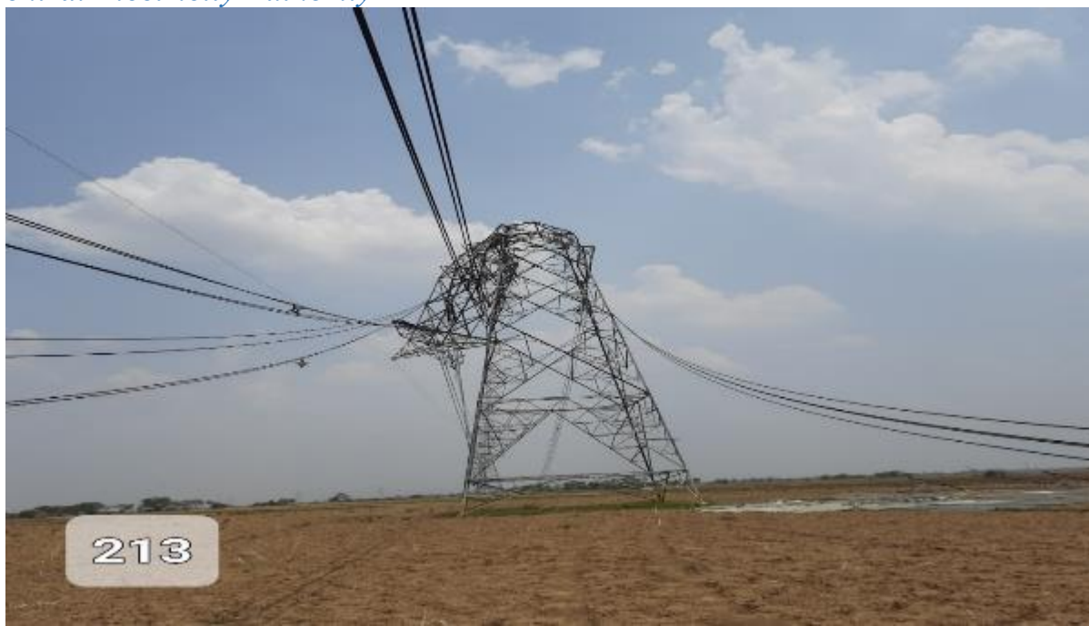
Fig 1(a). Tower at Location No.: 213 (DA+3)
