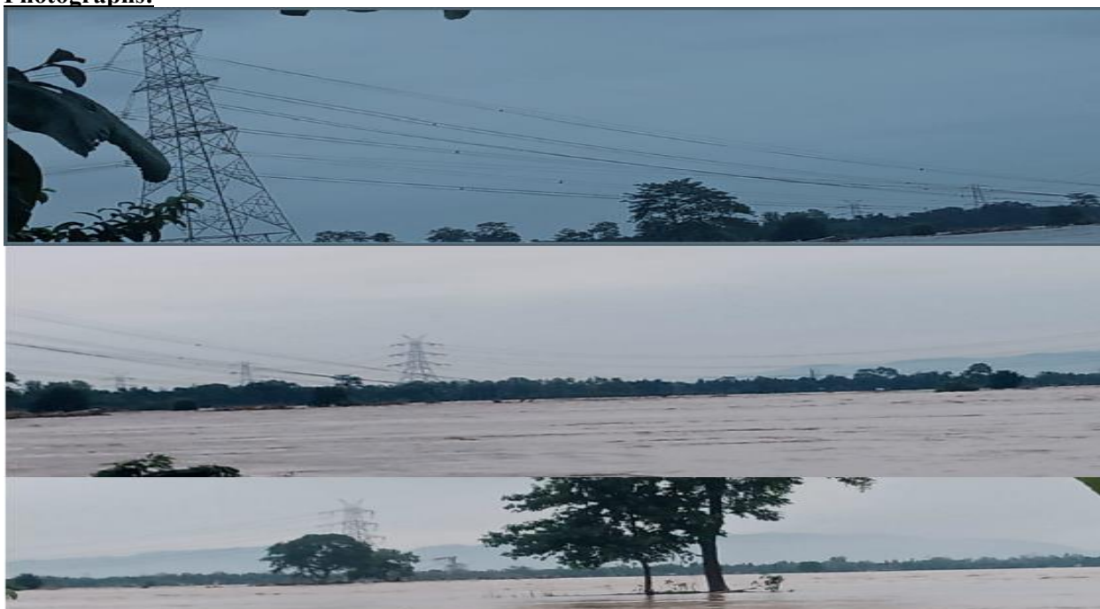
Fig 2(a). Surrounding Area to Damaged Towers
