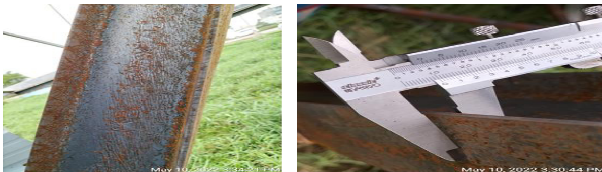
Fig 7(c). The roofs steel sections.
