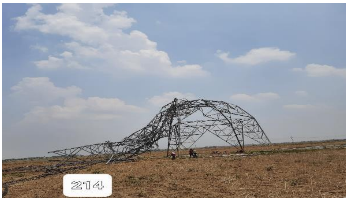
Fig 1(b). Tower at Location No.: 214 (DA+0)
