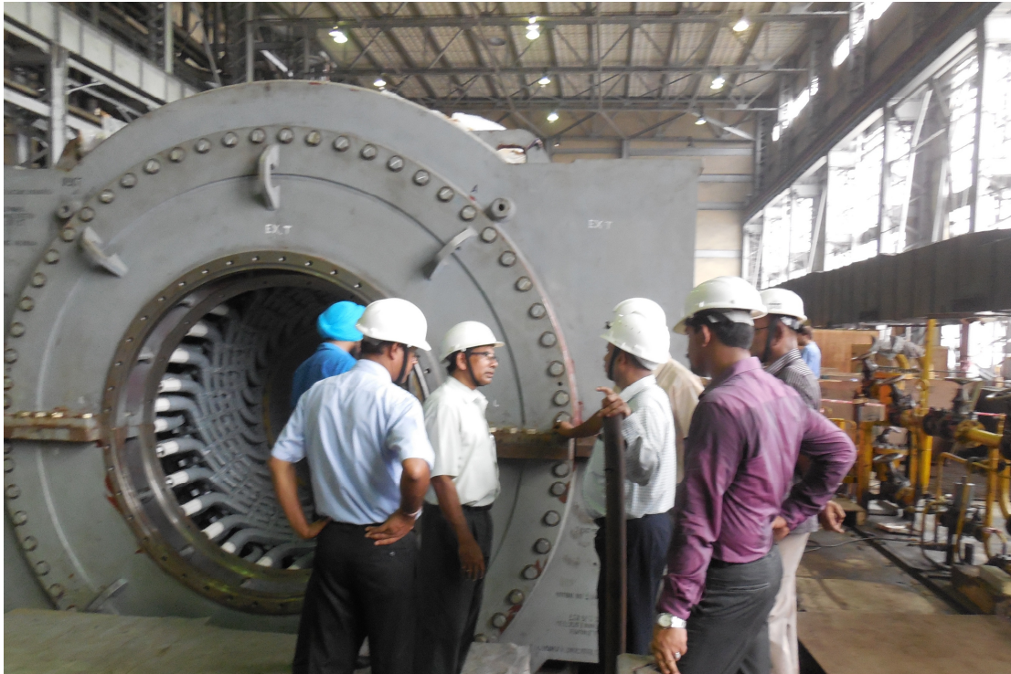
Energy Efficiency R&M Works at Bandel TPS Unit-5 (210 MW)
