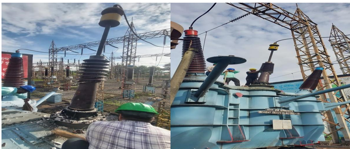
Damaged Bushing
