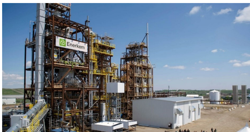
Figure 9-3: Enerkem MSW to Methanol plant. [11]
