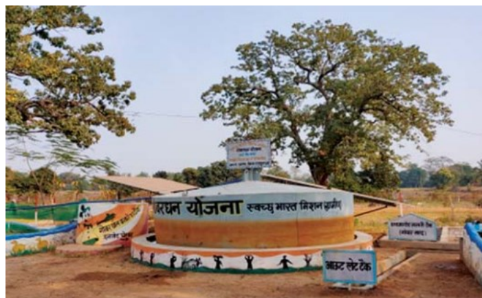
Figure 6-3: Community biogas plant at Bancharouda, Raipur, Chhattisgarh. [18]
