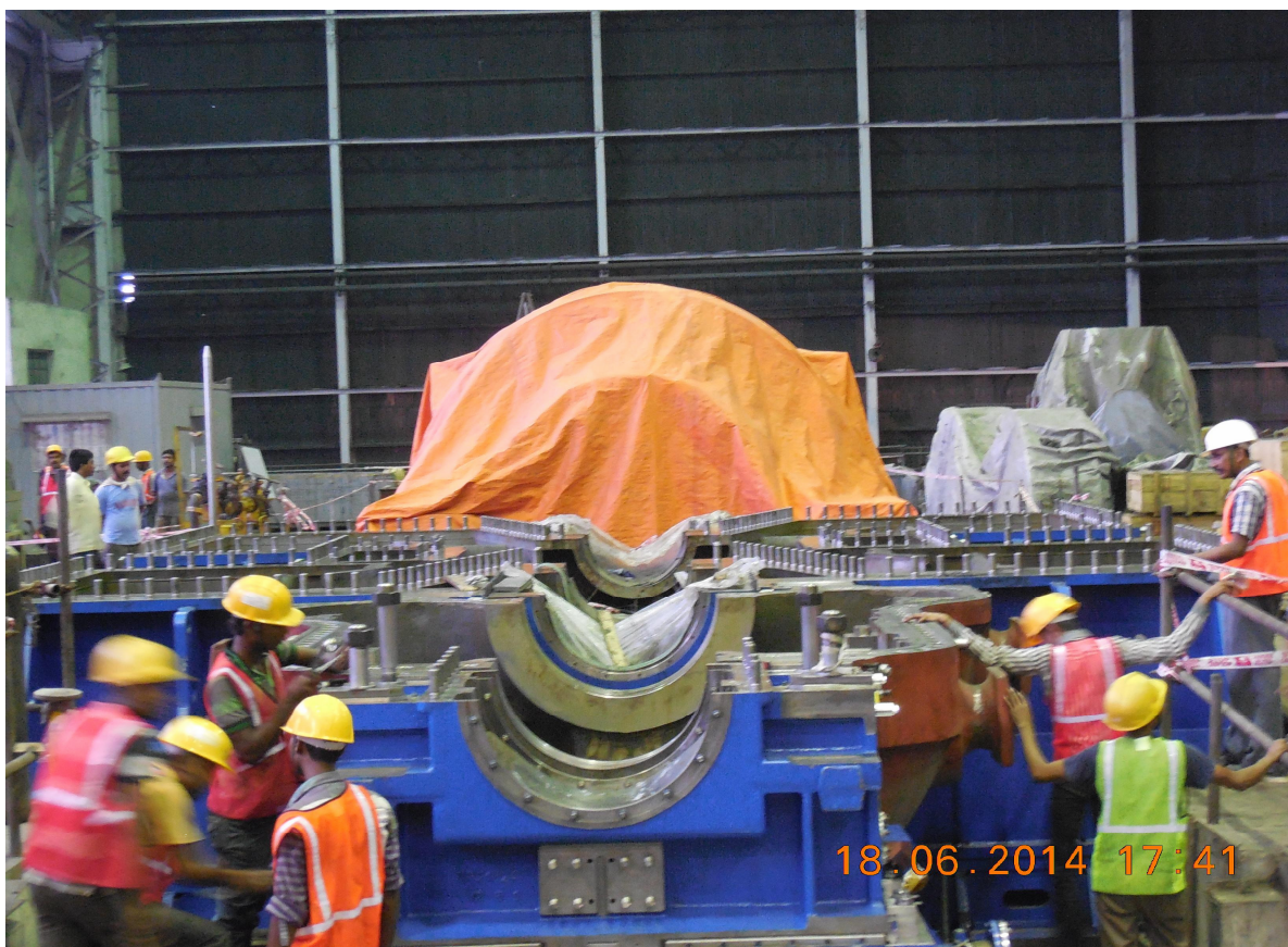
Energy Efficiency R&M Works at Bandel TPS Unit-5 (210 MW)
