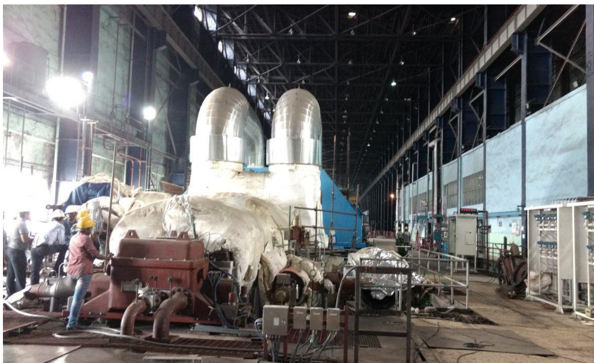
R&M of Unit-4 (200 MW) of Ukai TPS of GSECL
