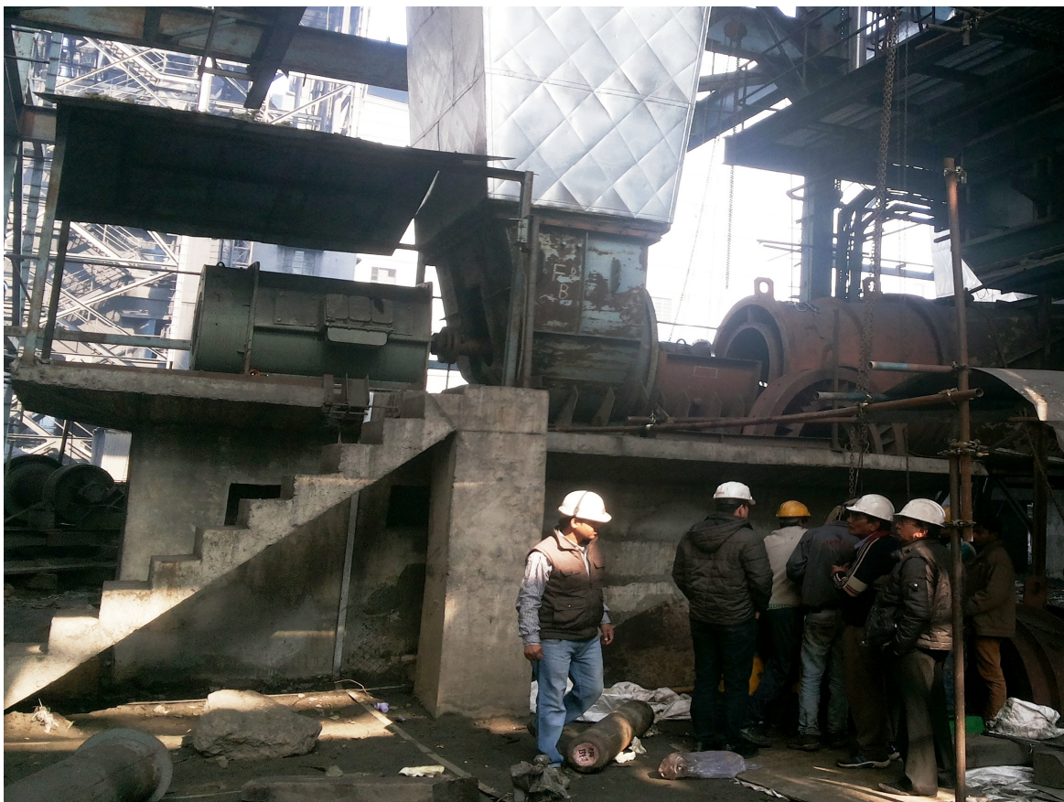
R&M Works at FD Fan-7 of Harduaganj TPS Unit-7(110 MW)
