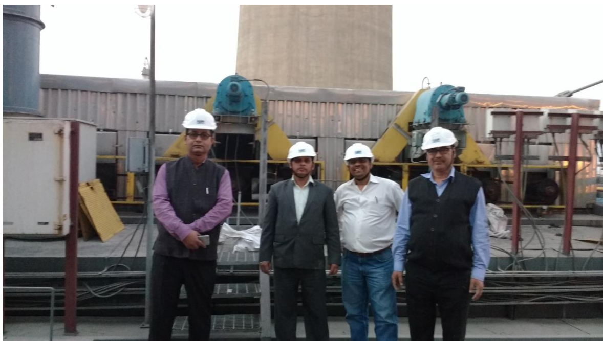
Retrofitting of Moving Electrode Electrostatic Precipitator at Rinhand TPS of NTPC
