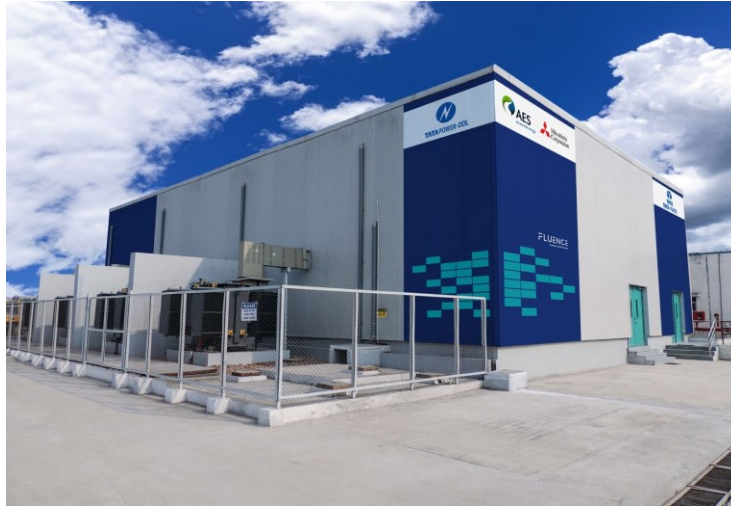
Figure 2-10: TATA Li-ion (NMC) Plant in Delhi.
