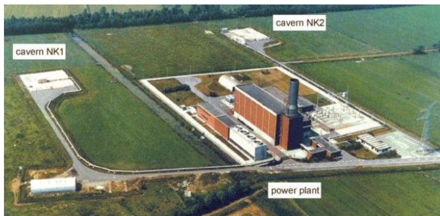
Figure 6-5: Aerial photo of the Huntorf facility [14].
