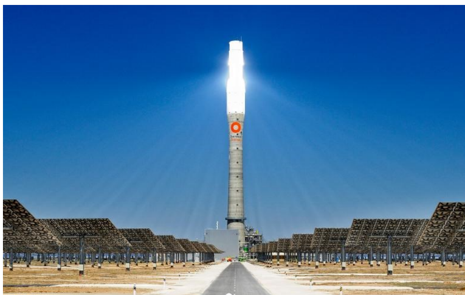
Figure 7-3: Central tower receiver surrounded by heliostat mirror arrangement [20].
