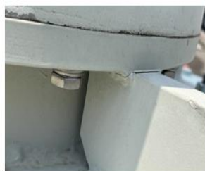
Crack observed on HV Bushings Flange
