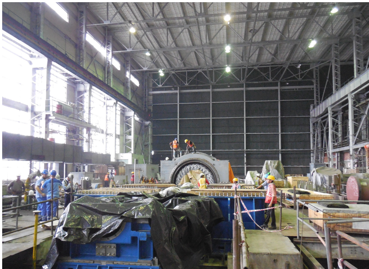
R&M Works at Unit-5 (210 MW) of Bandel TPS
