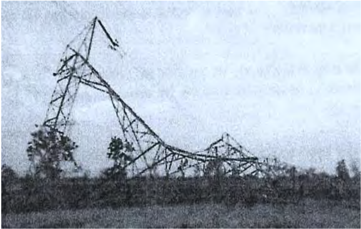
Tower at Loc. No. 320 (A+3)
