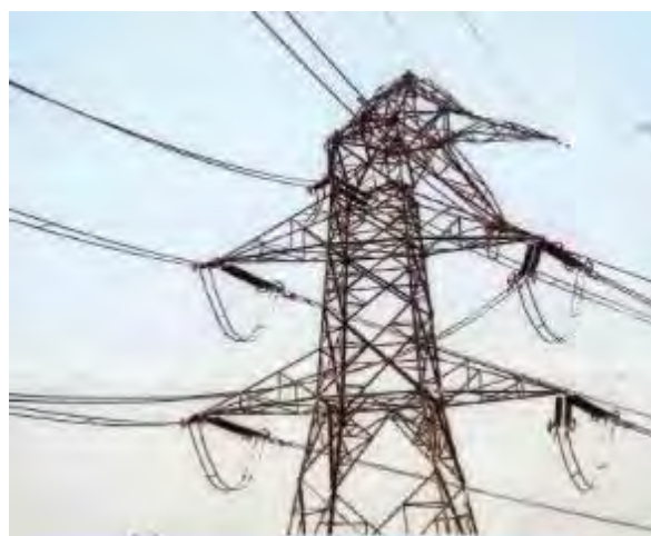
Tower at loc. No. 138 (FD 30)
