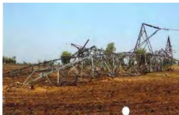
Tower at loc. No. 136 (FD 0)
