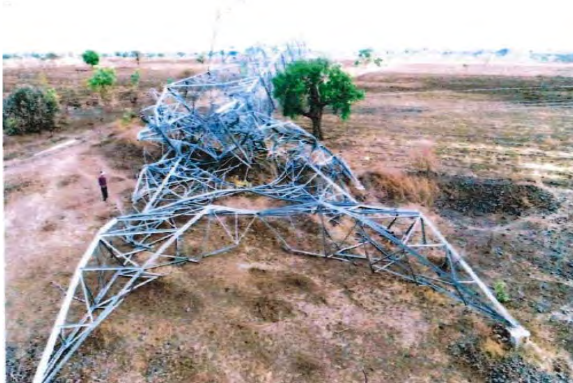
Tower at Location No. 321 (DA+3)
