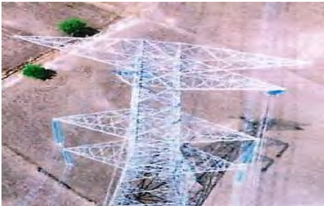
Tower at Location No. 318 (DA+3)
