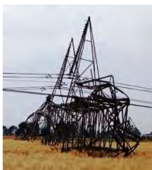
Tower at location No. 19 (FD0)
