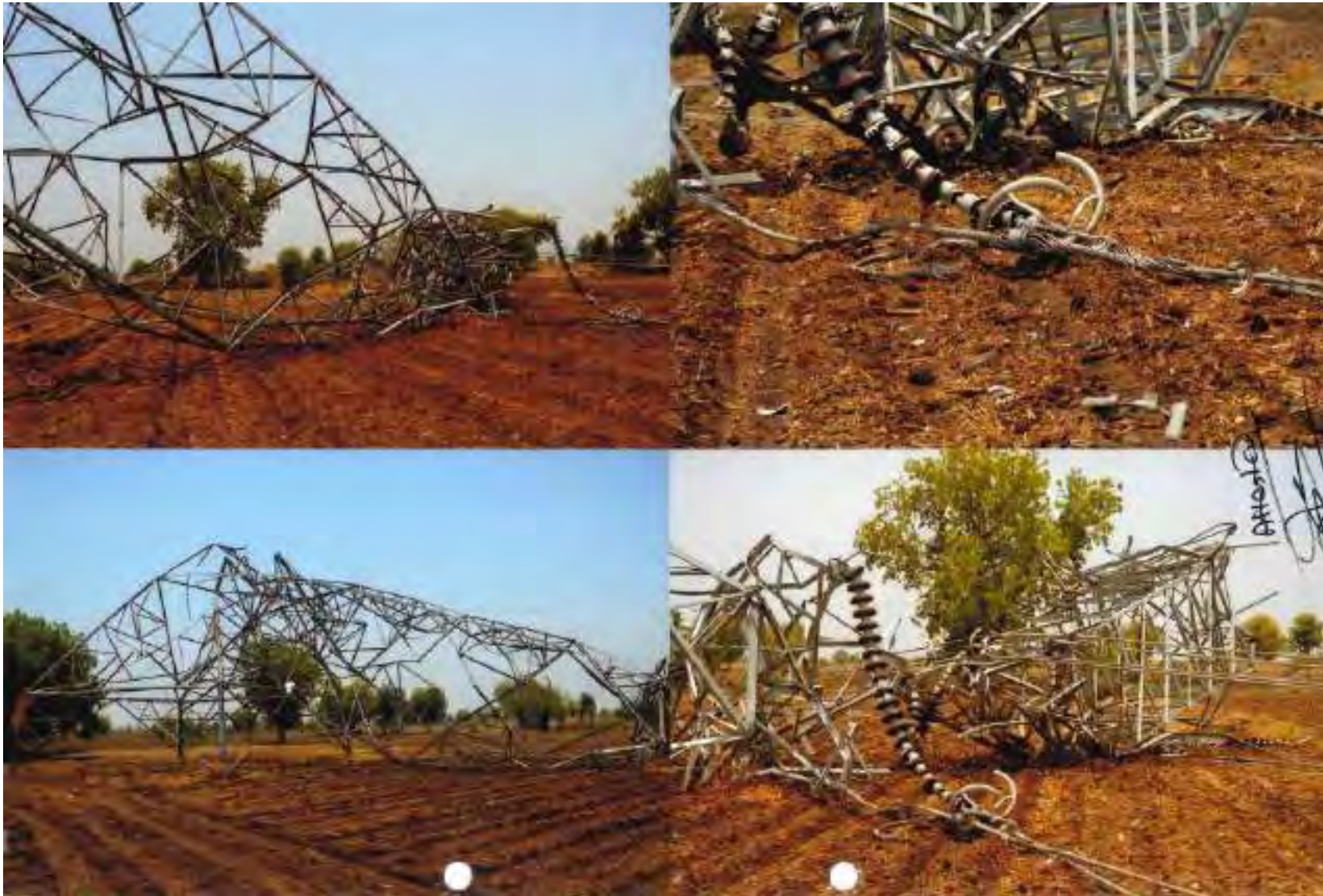
Tower at Location 135
