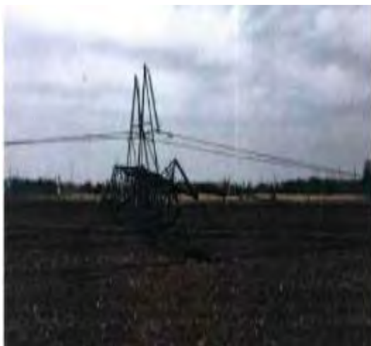
Tower at loc. No. 92
