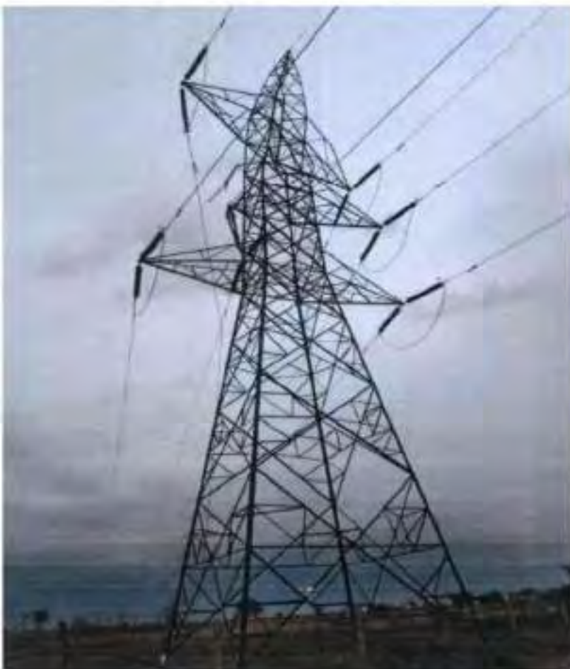
Tower at location 90
