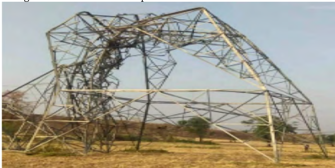
Tower at Loc. No.147 (A+6)
