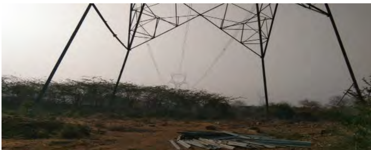
Tower at Loc. No.612 (A+0)
