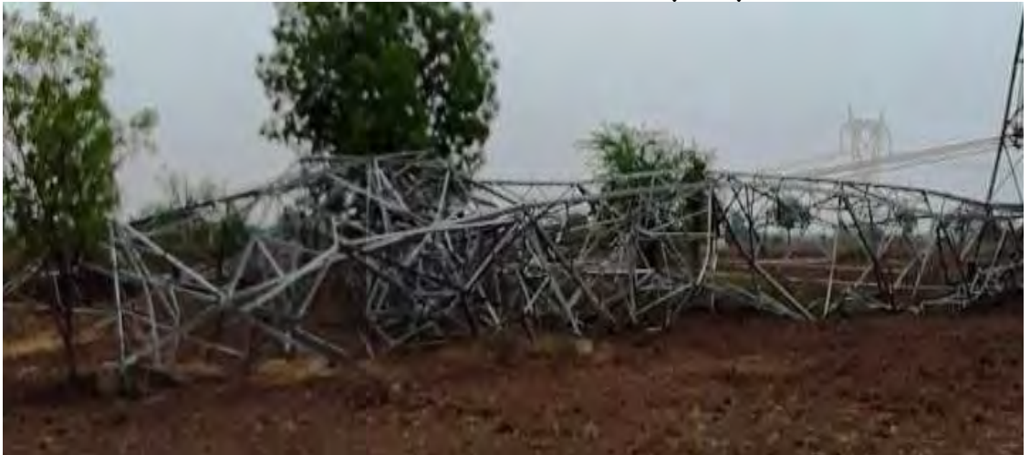
Tower at location No. 432 (A+3)
