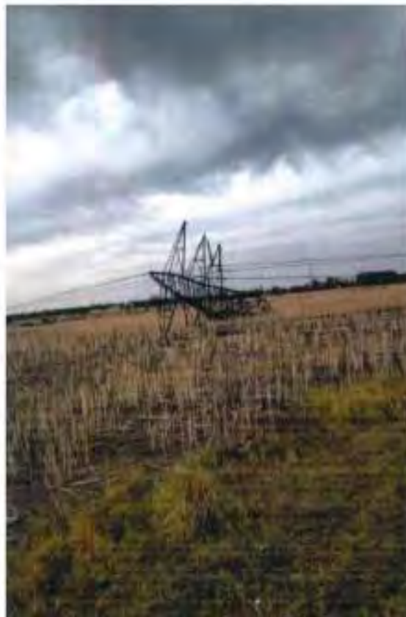
Tower at location 93
