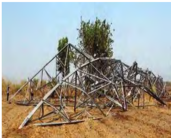
Tower at loc. No. 132 (FD 60)
