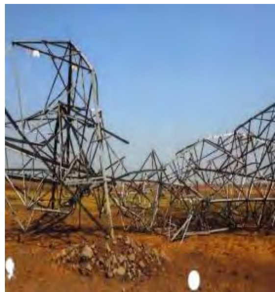
Tower at loc. No. 162 (FD0)
