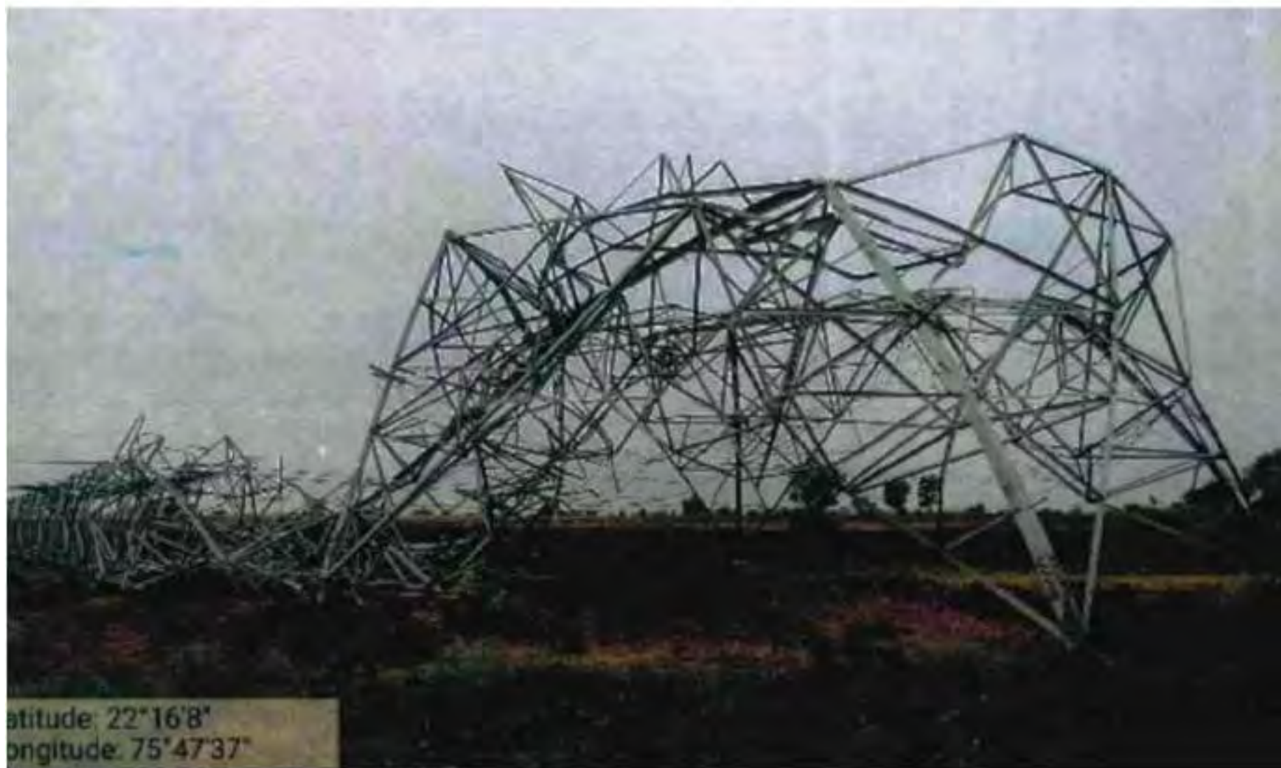
Tower at location 150
