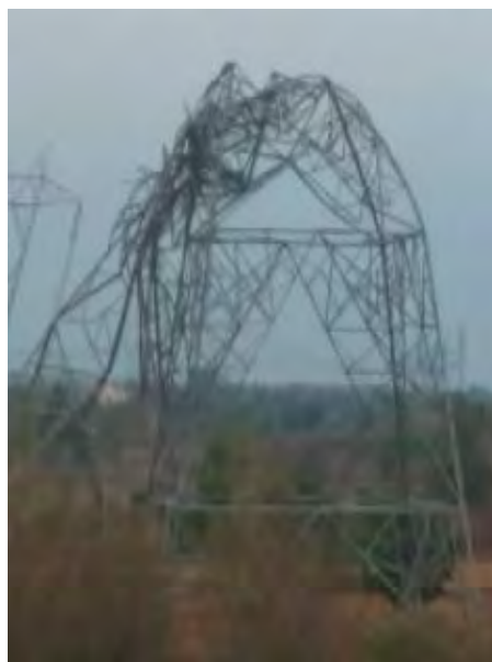
Tower at Loc. No.162 (A+6)
