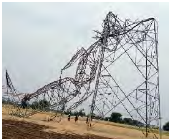
Tower at location No. 16 (FD0)
