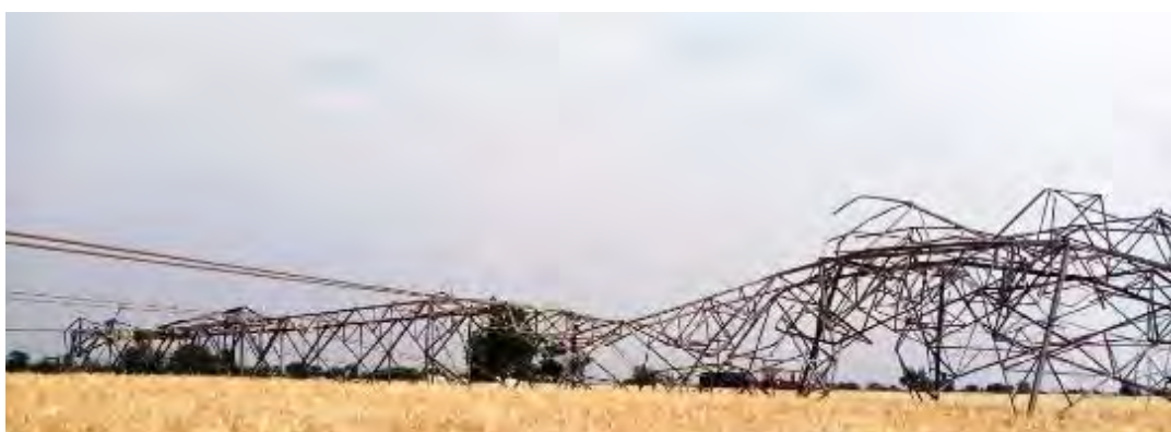
Tower at location No. 17 (FD0+6)
