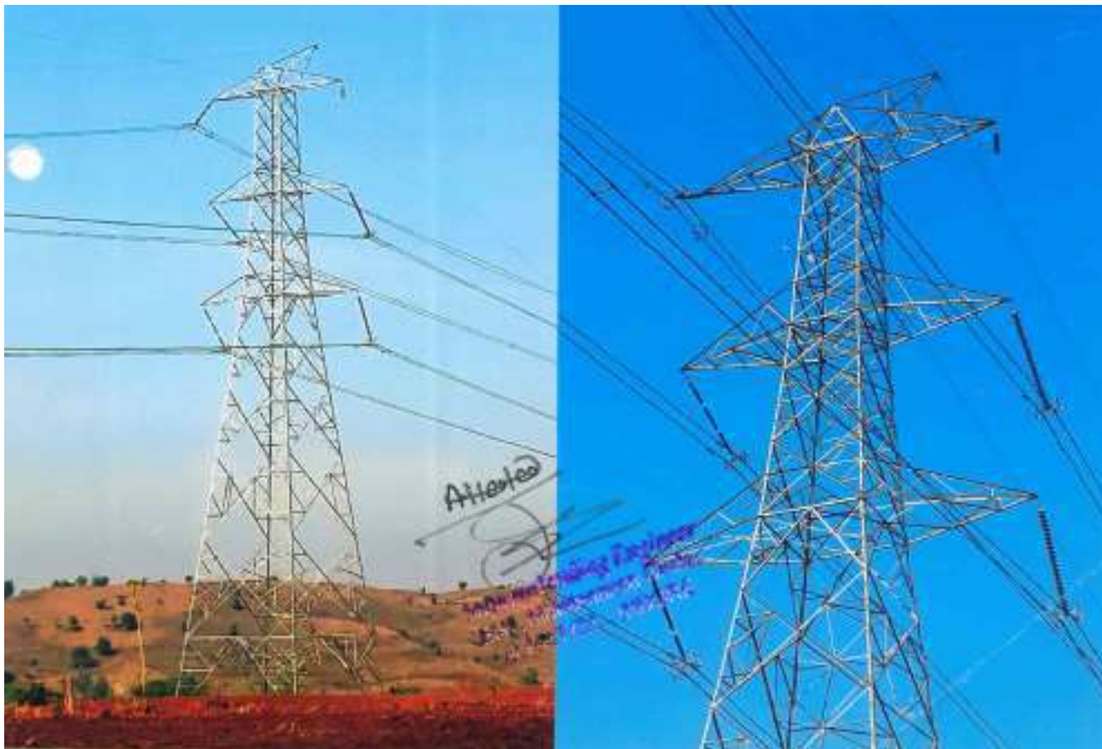
Tower at location 563
