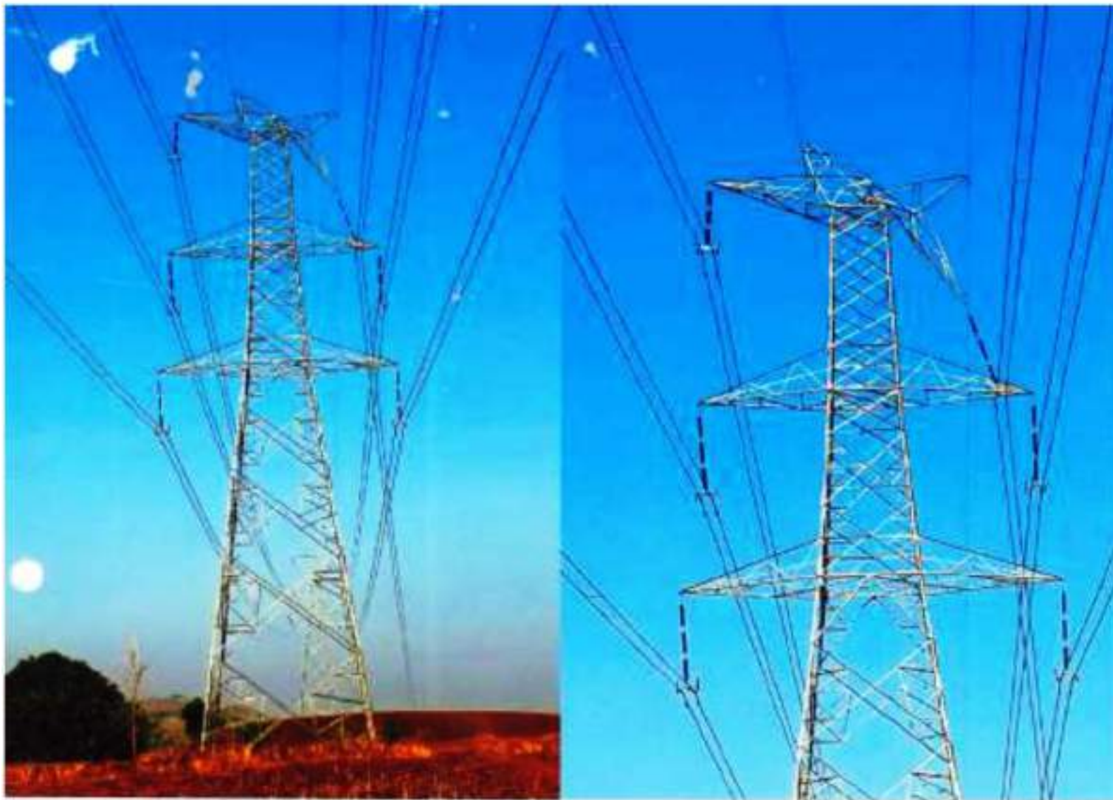
Tower at location 562
