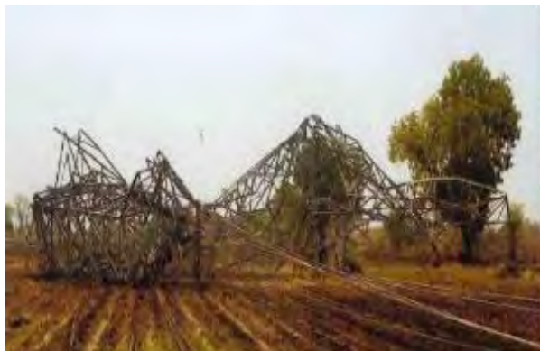
Tower at loc. No. 130 (FD0+3)
