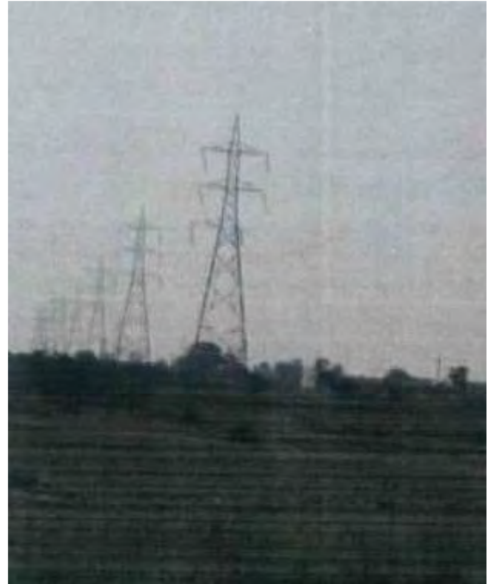
Tower at location 33
