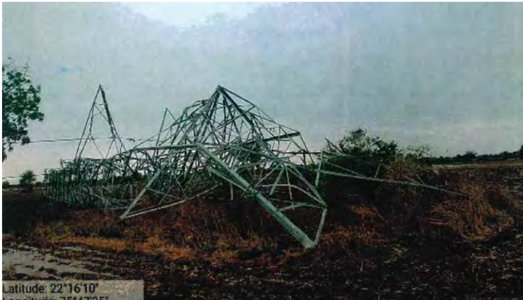
Tower at location 149
