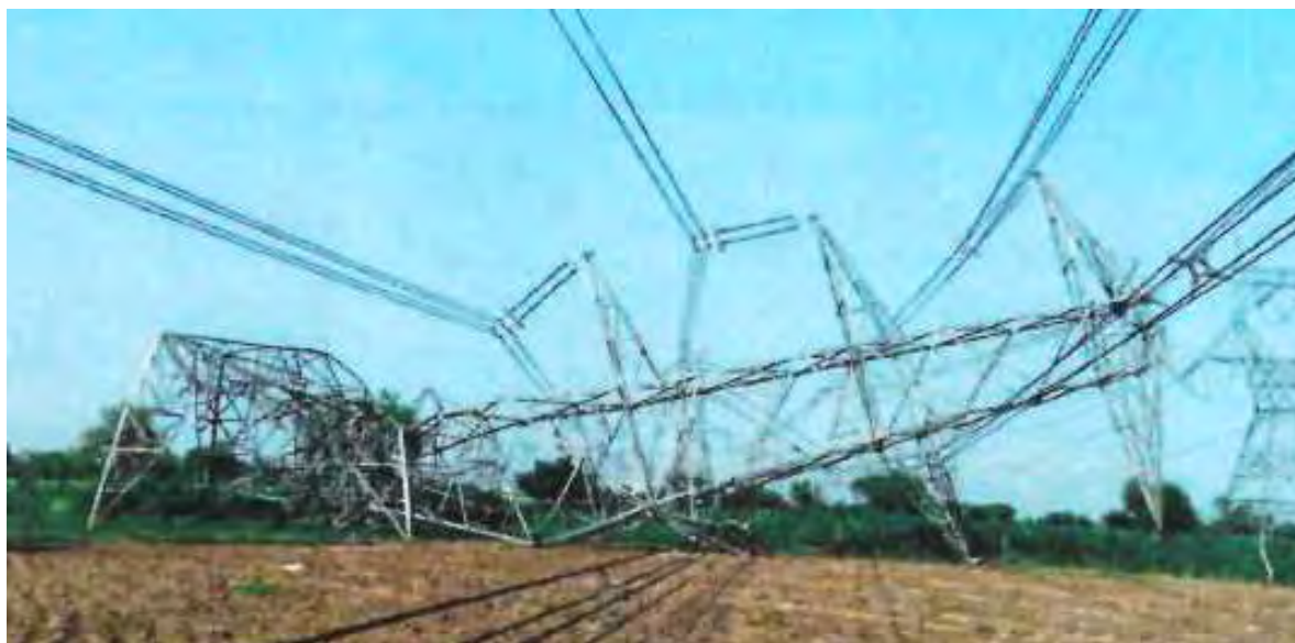
Tower at Location No. 12 (DA+0)
