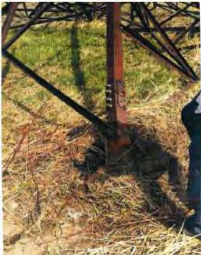
Tower at location 19
