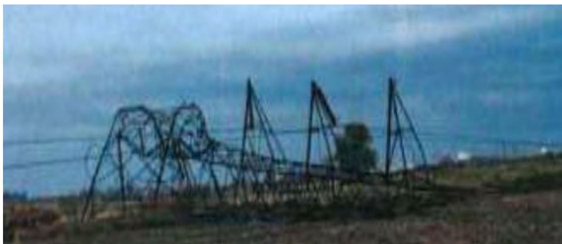
Tower at location No. 91
