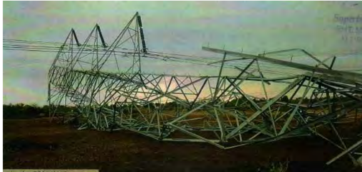
Tower at location 148
