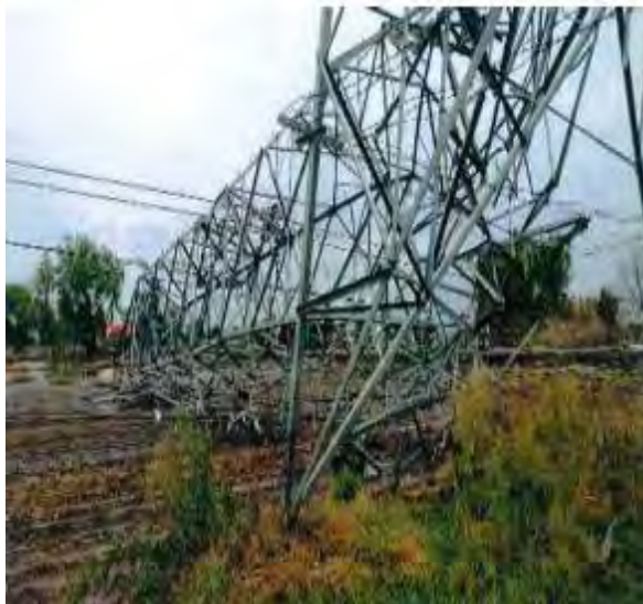
Tower at location No. 151 (FD0)
