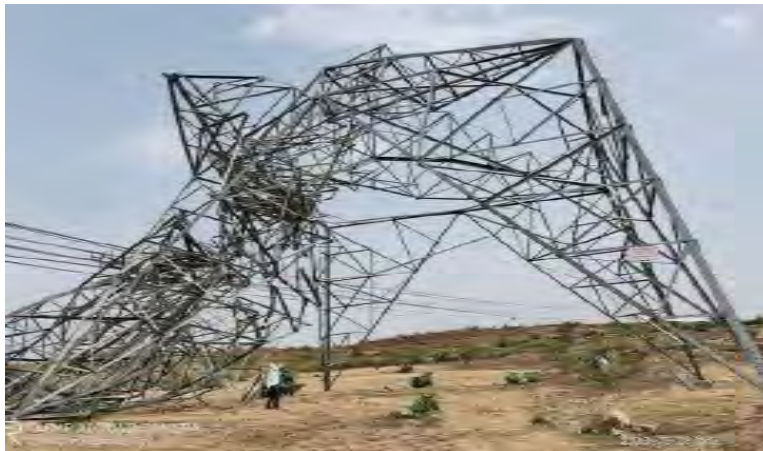
Tower at Loc. No.181 (A+9)
