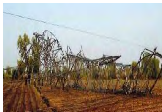
Tower at loc. No. 137 (FD0)
