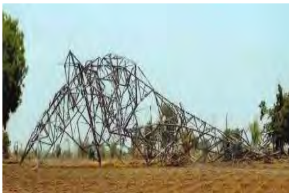
Tower at loc. No. 134 (FD 0)
