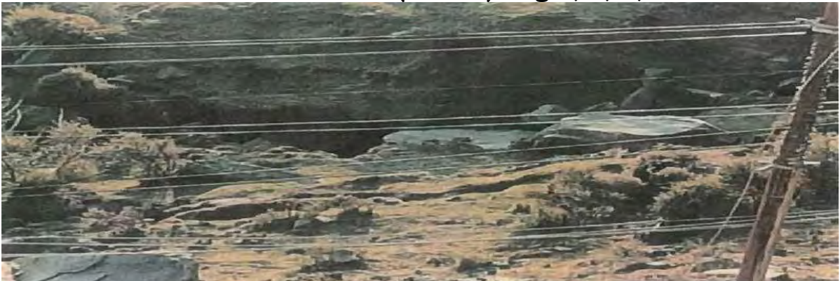
Tower at Loc. No.145 (DC+3R): Leg-A, B, C, D
