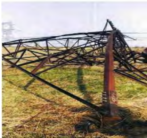
Tower at location No. 14
