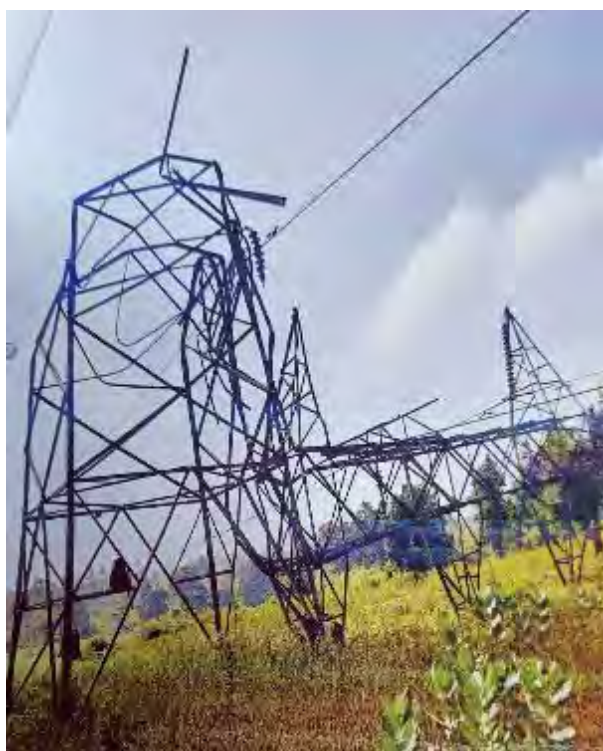
Tower at location No. 84
