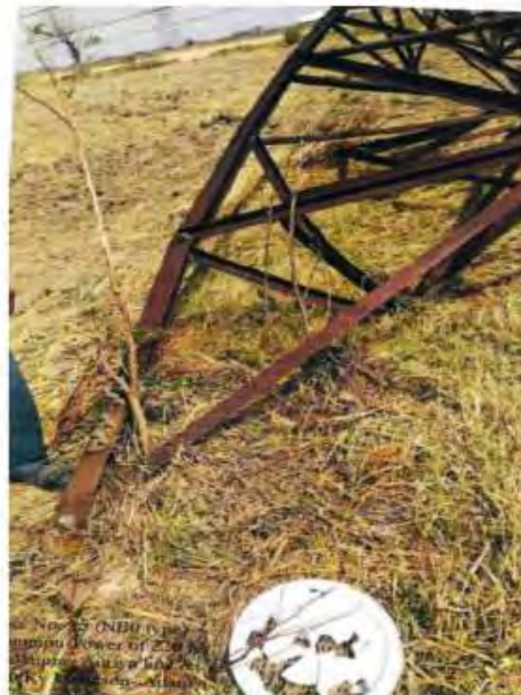
Tower at location 15
