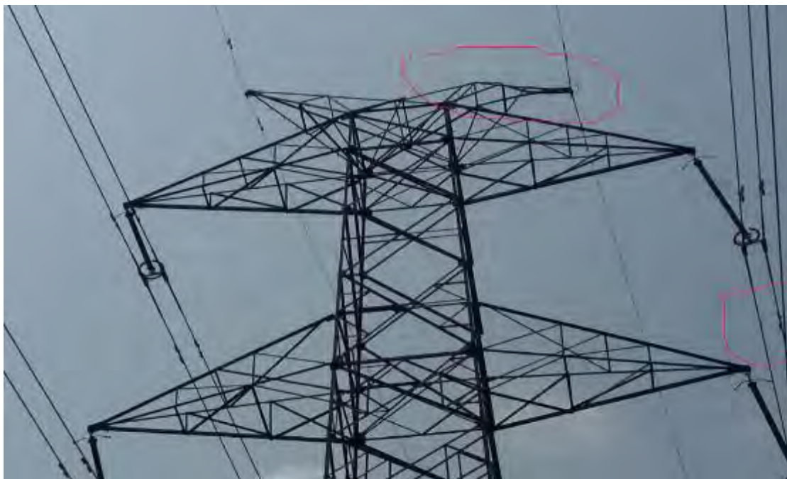
Tower at location No. 360 (DA+0)
