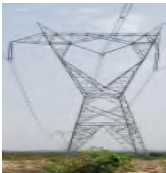
Tower at Loc. No.180 (A+3)
