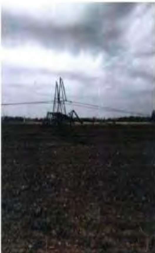
Tower at location 92
