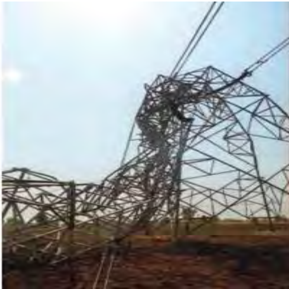
Tower at loc. No. 128 (FD0)
