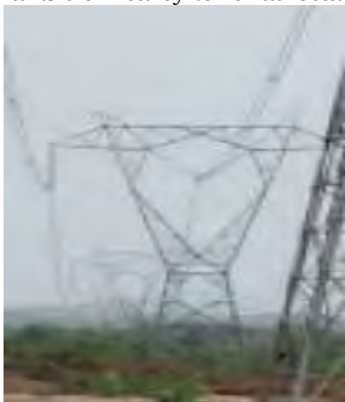
Tower at Loc. No.179 (A+3)
