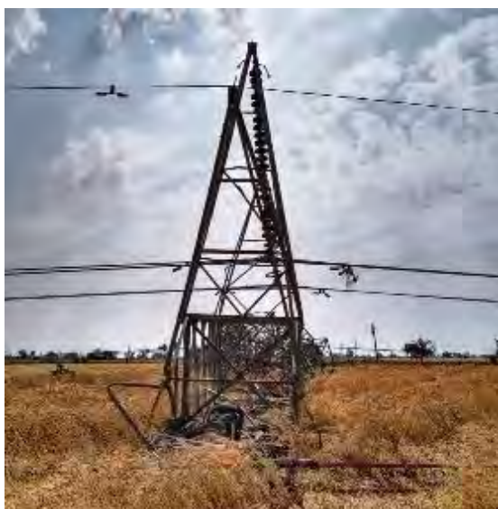
Tower at location No. 18 (FD0+3)
