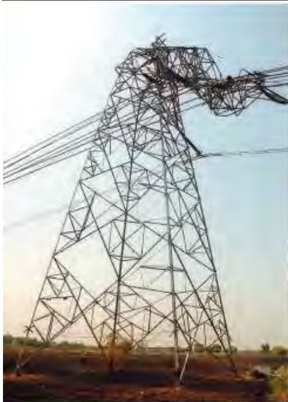
Tower at loc. No. 126 (FD0)
