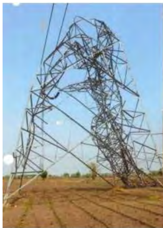
Tower at loc. No. 127 (FD0)
