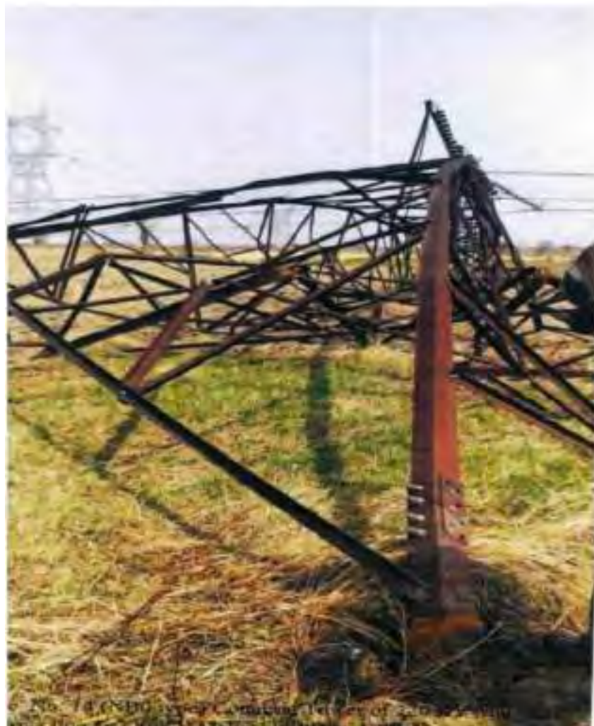
Tower at location 14
