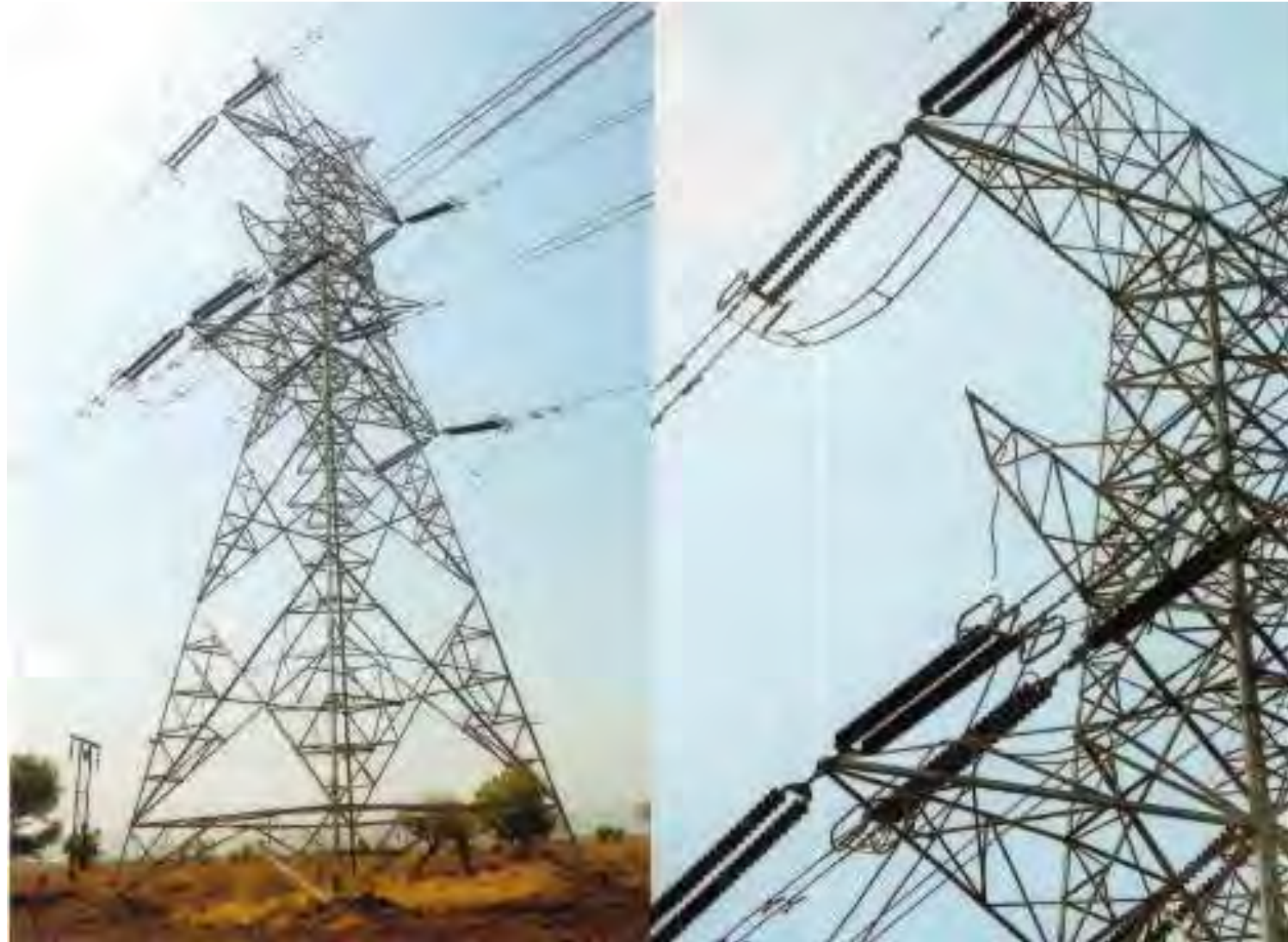
Tower at Location 159
