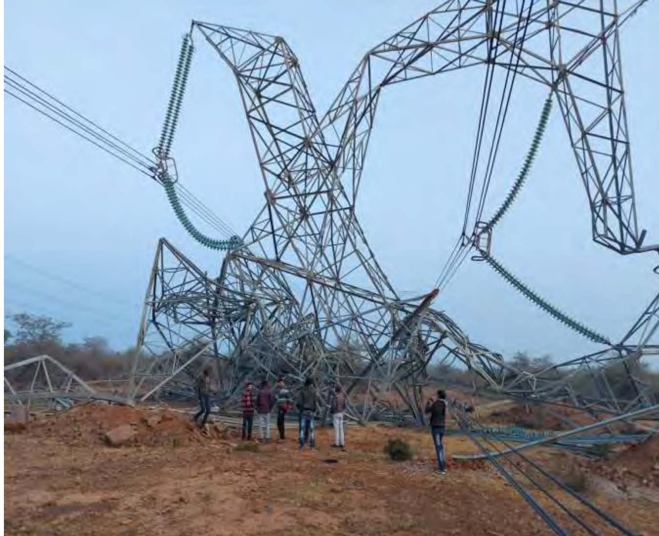
Tower at location 611
