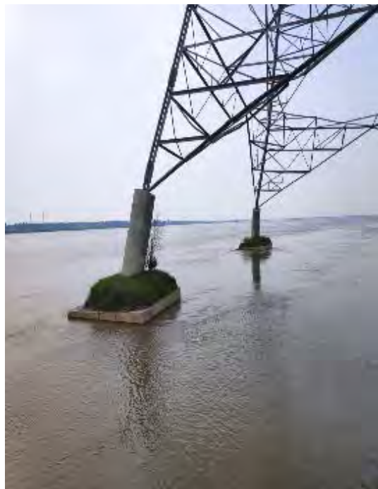
Location No. 409 (DC+0) (Just before Collapse of Tower)
