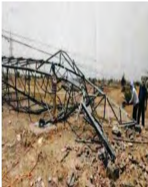
Tower at location No. 17
