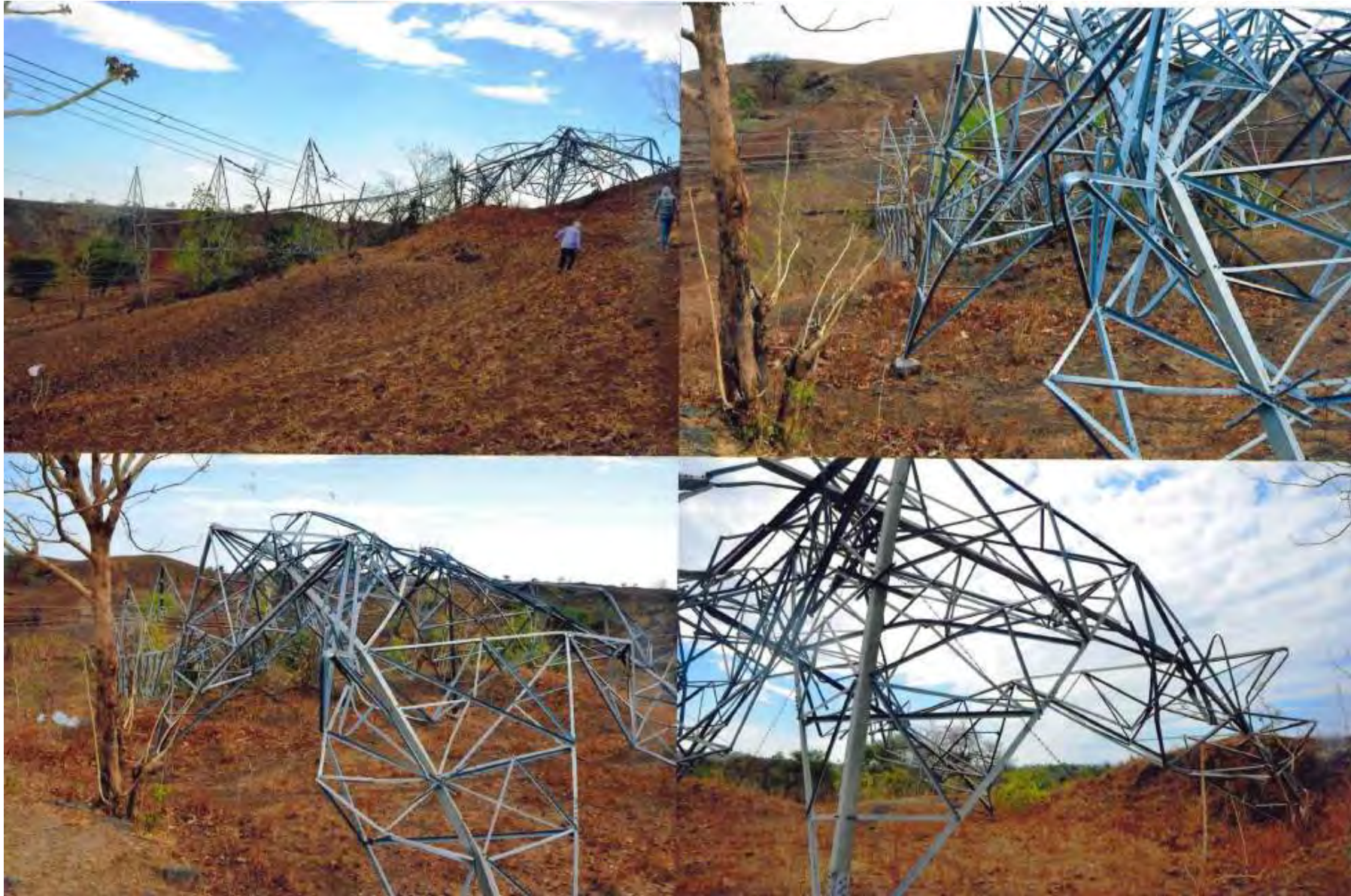
Tower at location 565
