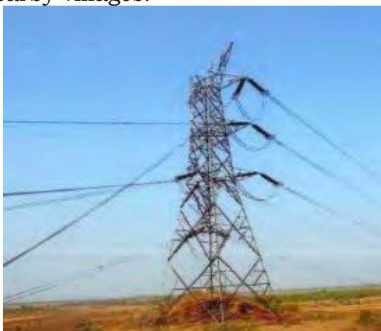
Tower at loc. No. 168 (FD 30)
