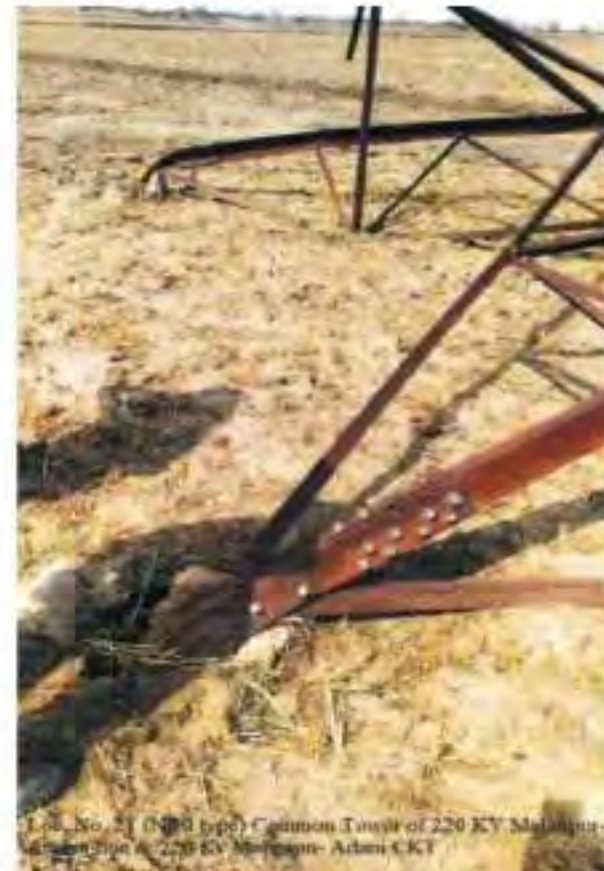
Tower at location 21
