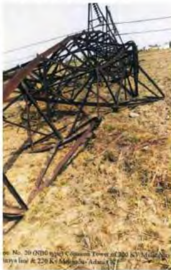
Tower at location 20
