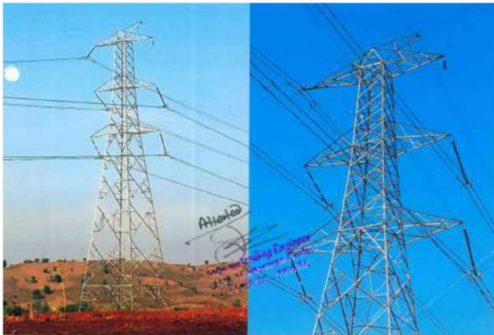
Tower at location 563
