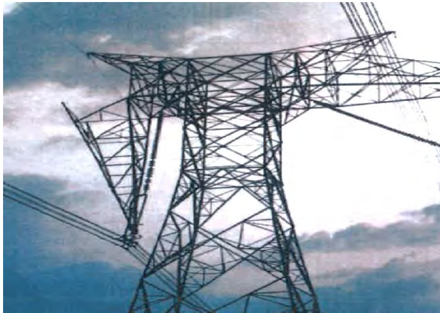
Tower at Loc. No. 3118 (A+0)
