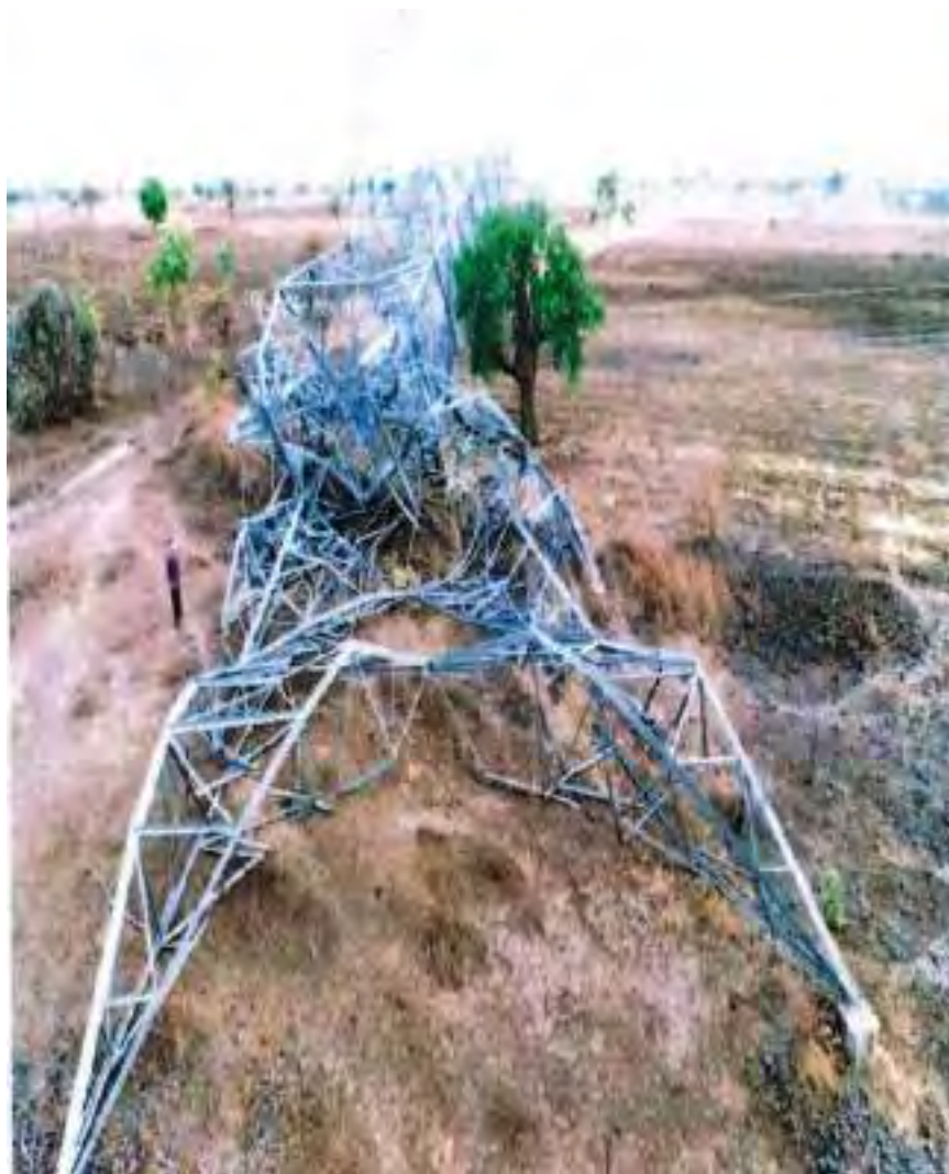
Tower at location 321
