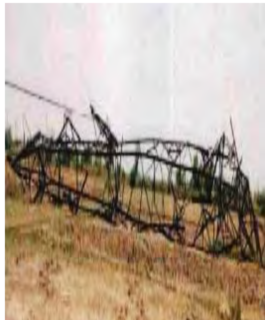
Tower at location No. 18
