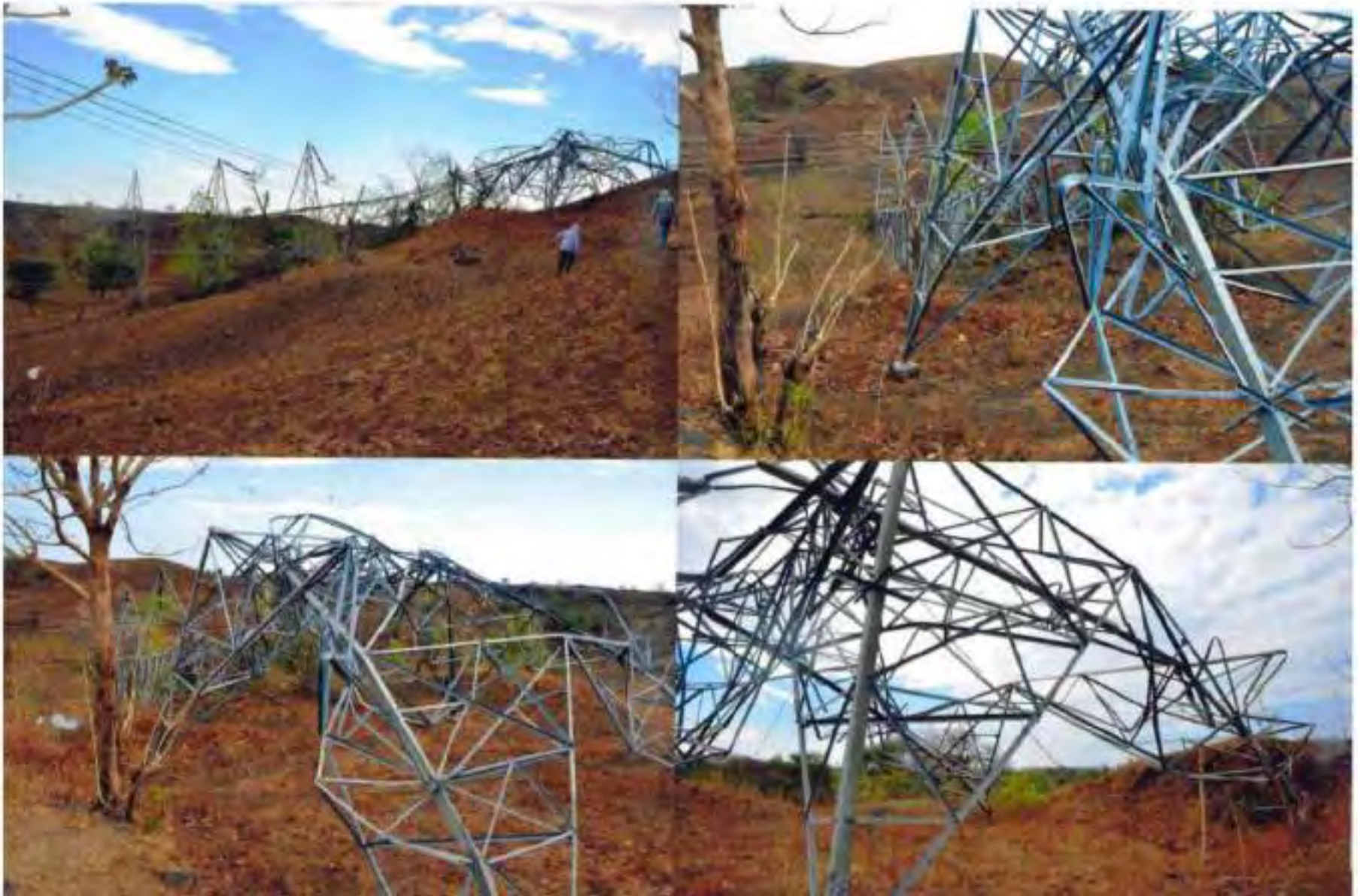
Tower at location 565
