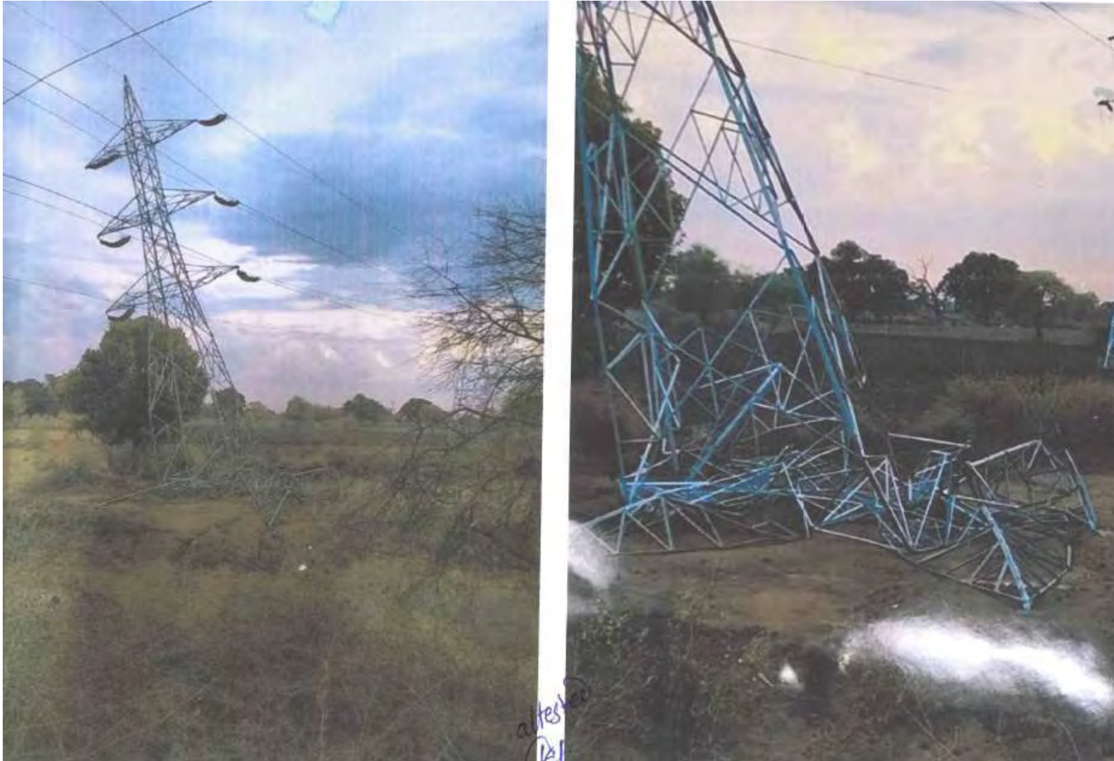
Tower at location 11A
