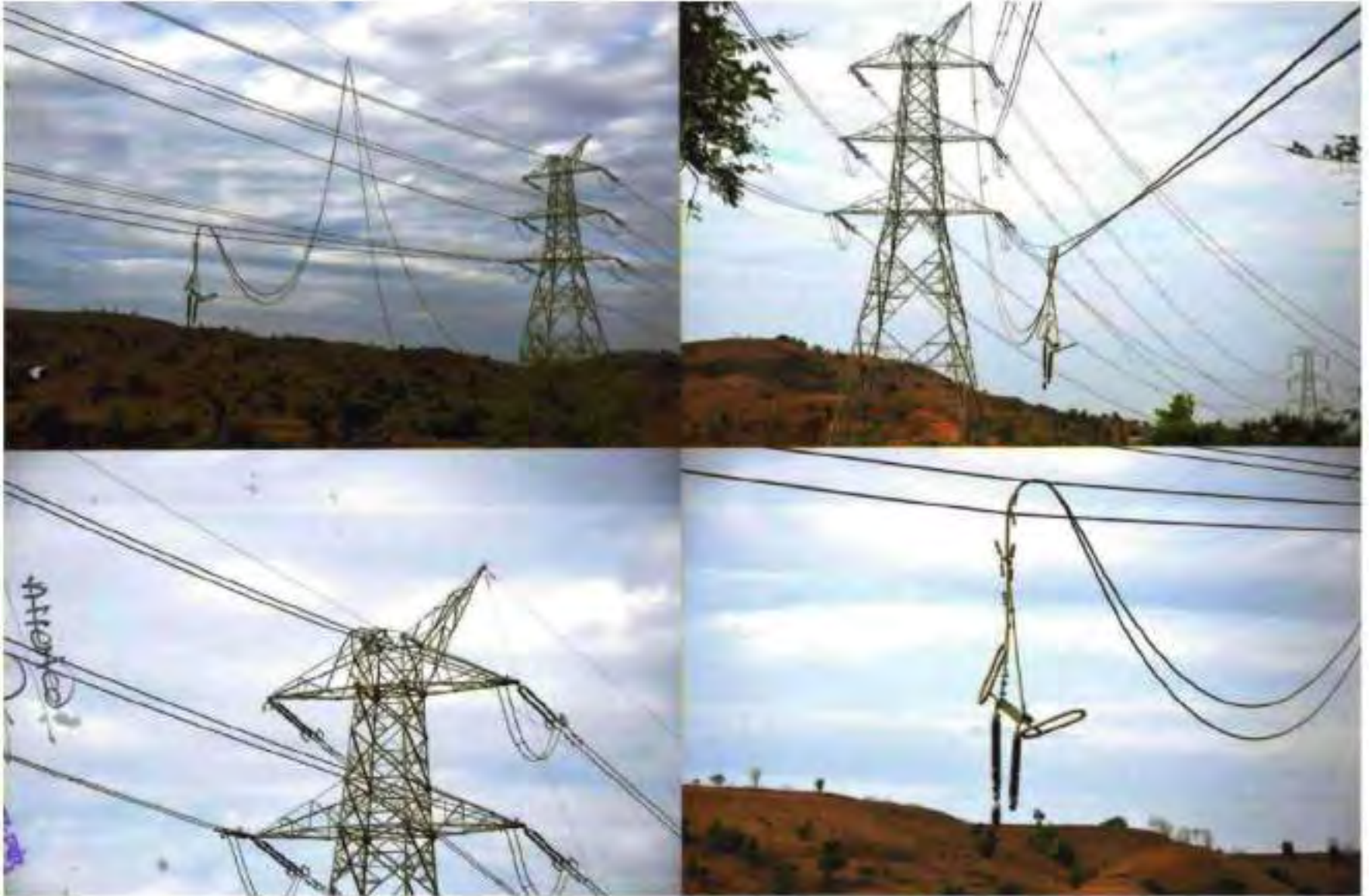
Tower at location 566
