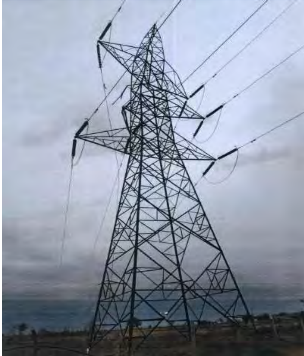
Tower at location 90
