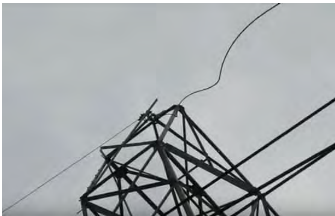
Tower Location No. 90 (A+3)
