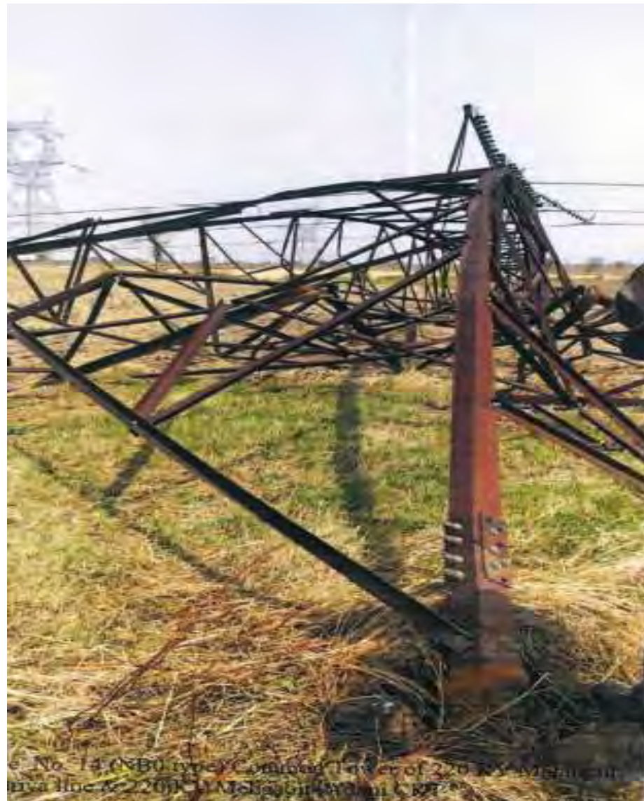
Tower at location 14
