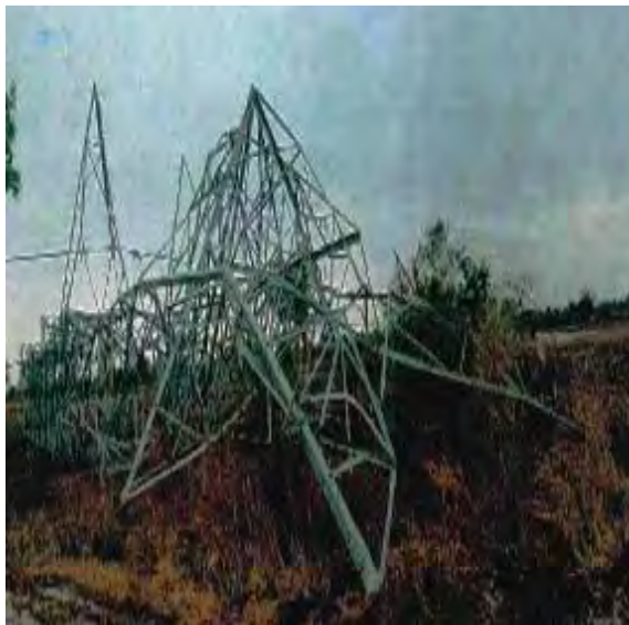
Tower at location No. 149 (FD0)
