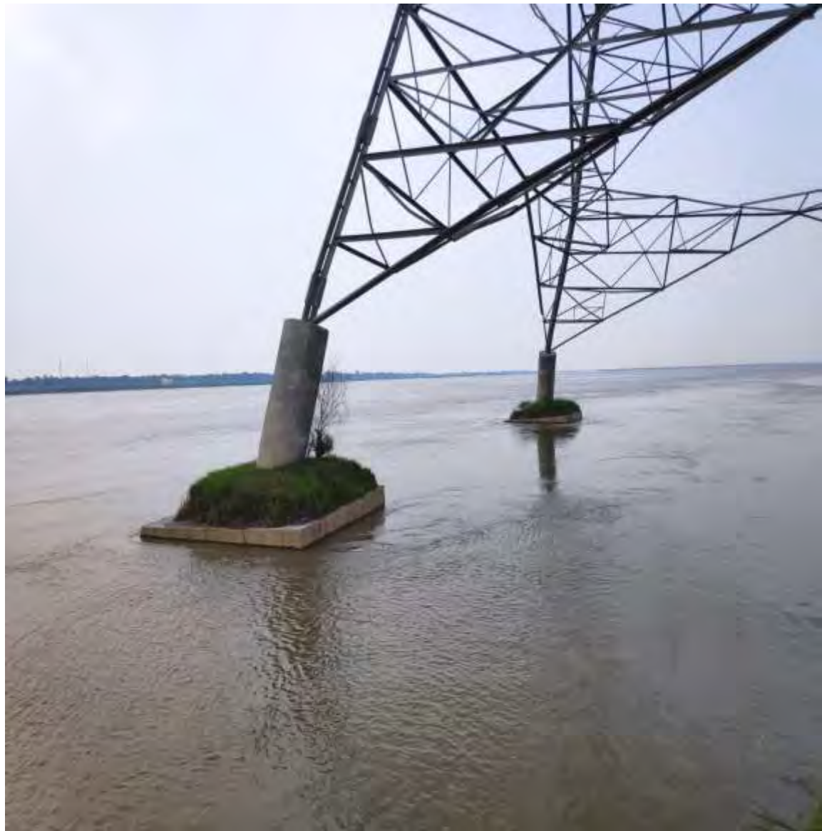
Tilt in tower legs causing bending of members
