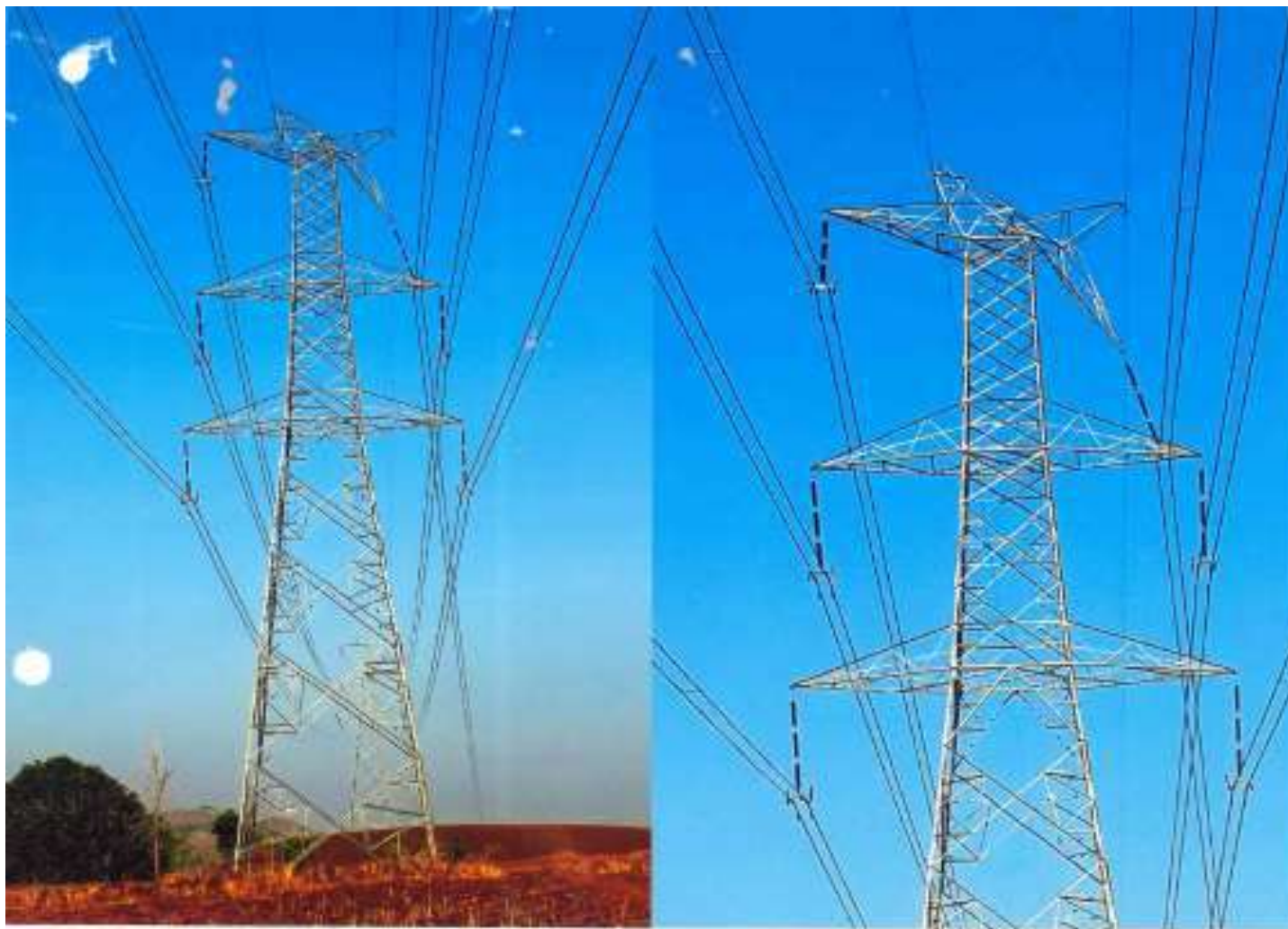
Tower at location 562
