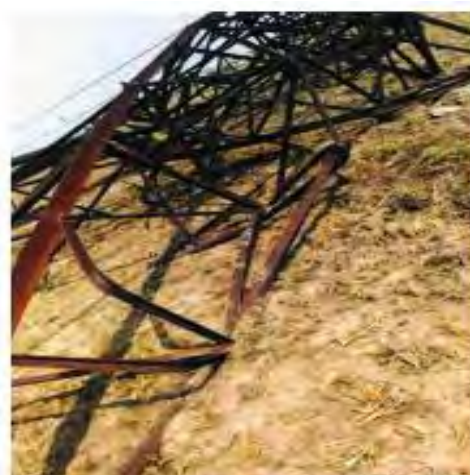
Tower at location No. 23
