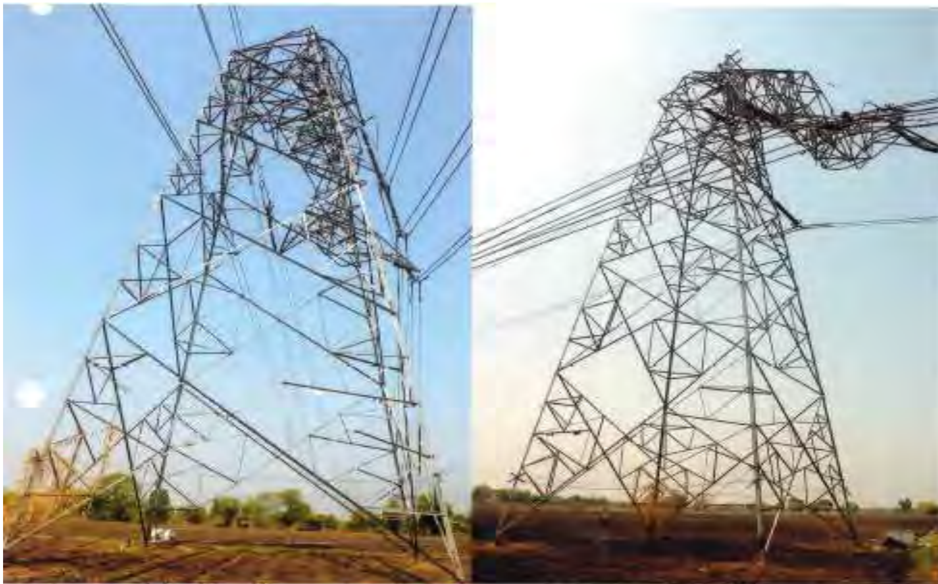
Tower at Location 126
