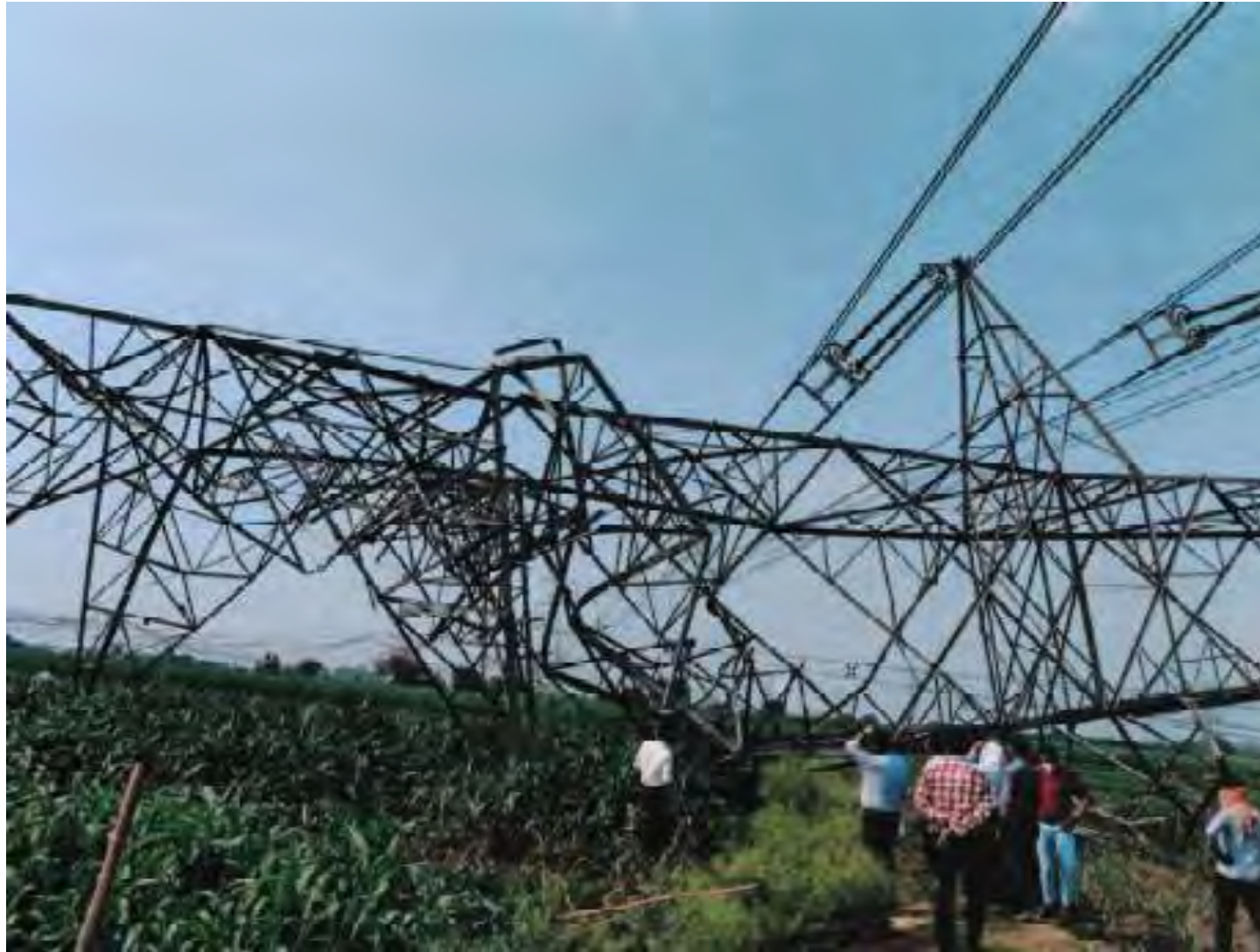
Tower at location 389
