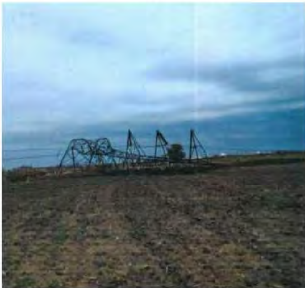
Tower at location 91
