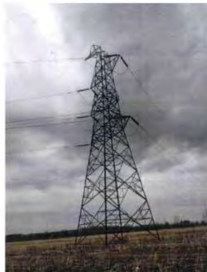
Tower at location 94
