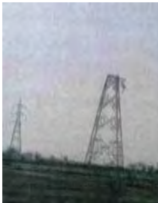
Tower at loc. No. 31 (B0 +3)
