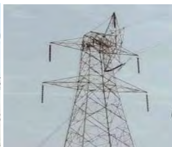
Tower at loc. No. 139 (FD0+6)
