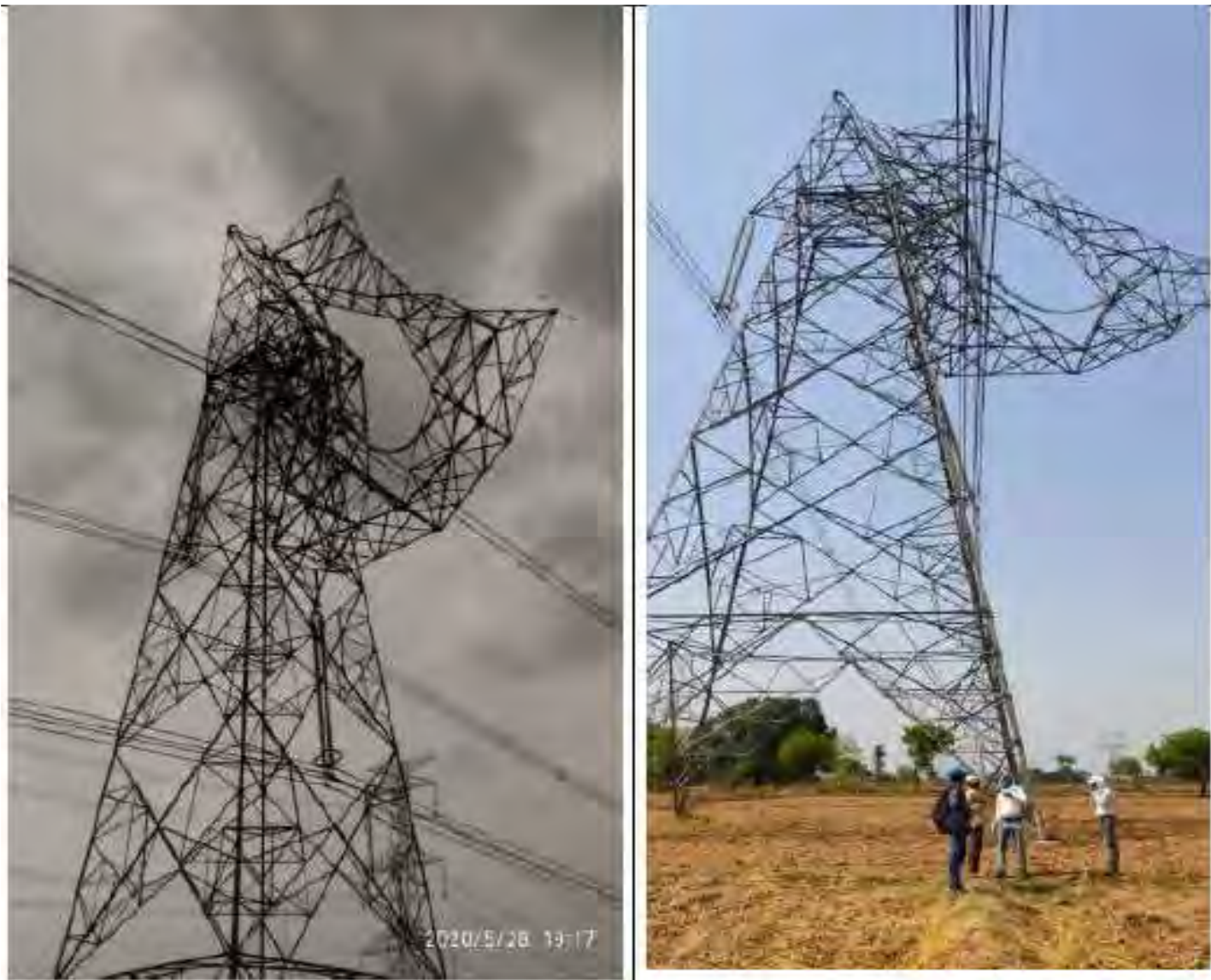
Tower at location 673
