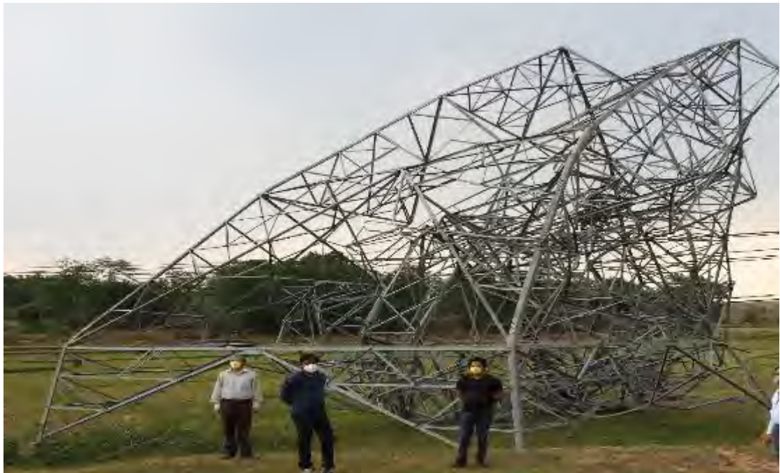
Tower Location No. 92 (A+3)
