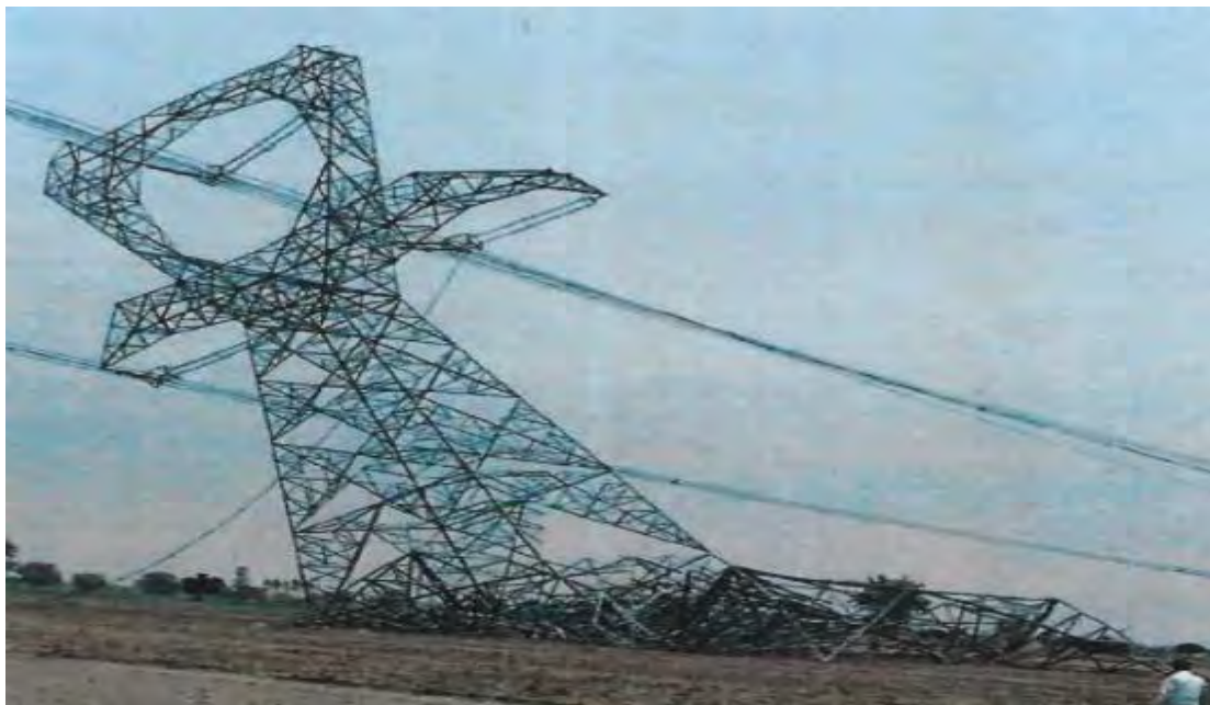
Tower at Loc. No.293 (B+25)
