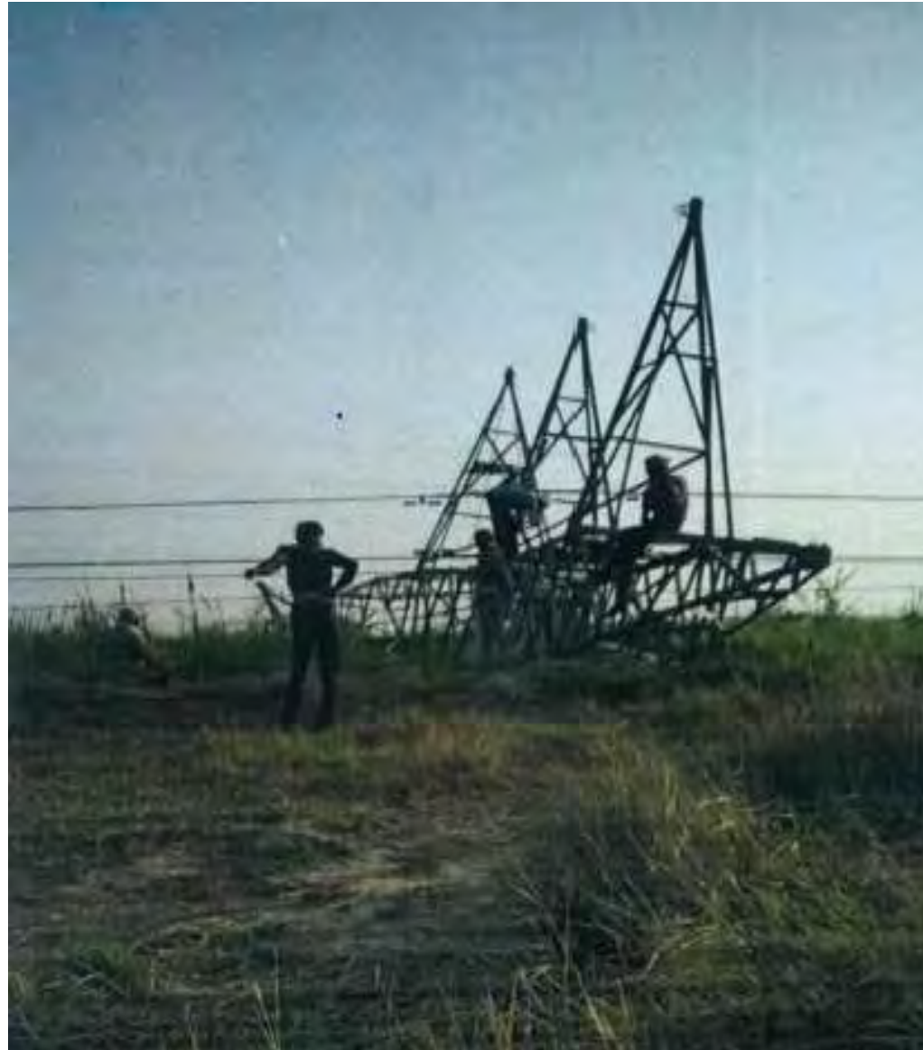
Tower at location 31
