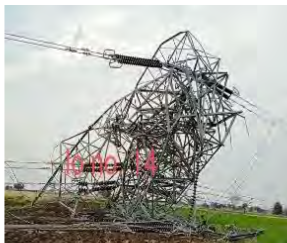
Tower at location No. 14 (FTP 30)
