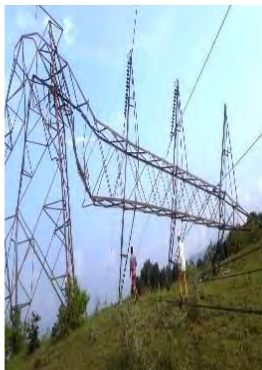
Tower at location No. 85
