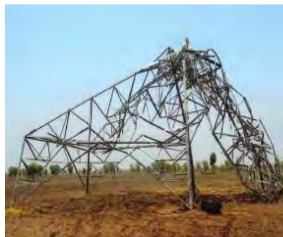
Tower at loc. No. 133 (FD0+3)
