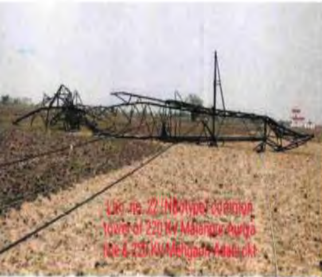
Tower at location 22
