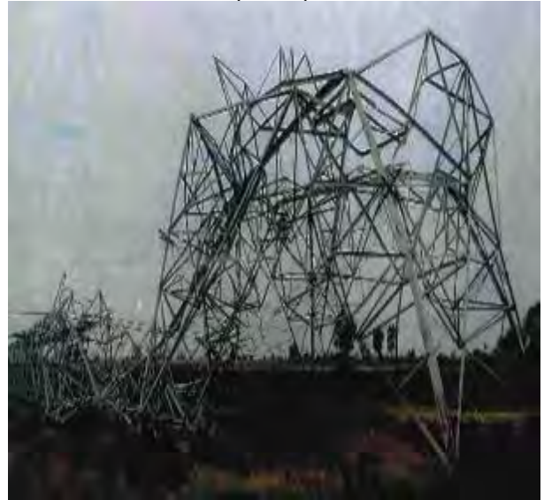
Tower at location No. 150 (FD0+6)
