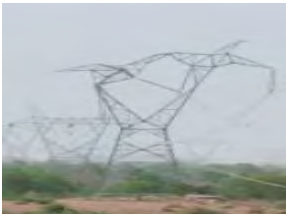
Tower at Loc. No.182 (B+6)
