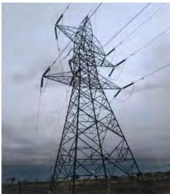
Tower at location No. 90
