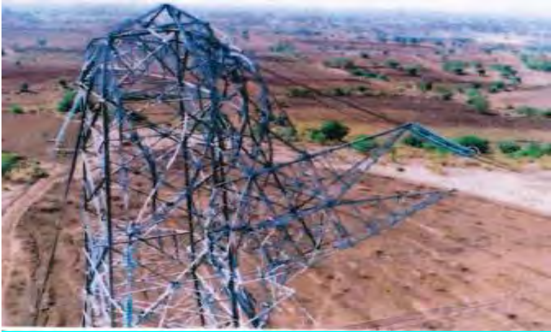
Tower at Location No. 319 (DA+0)
