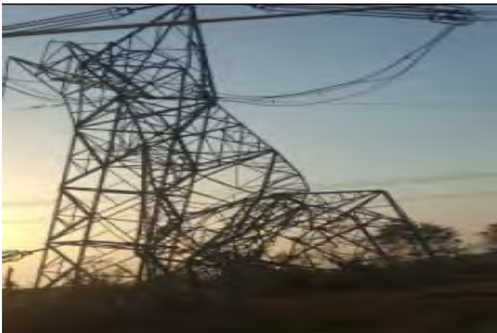
Tower at Loc. No.164 (D+3)
