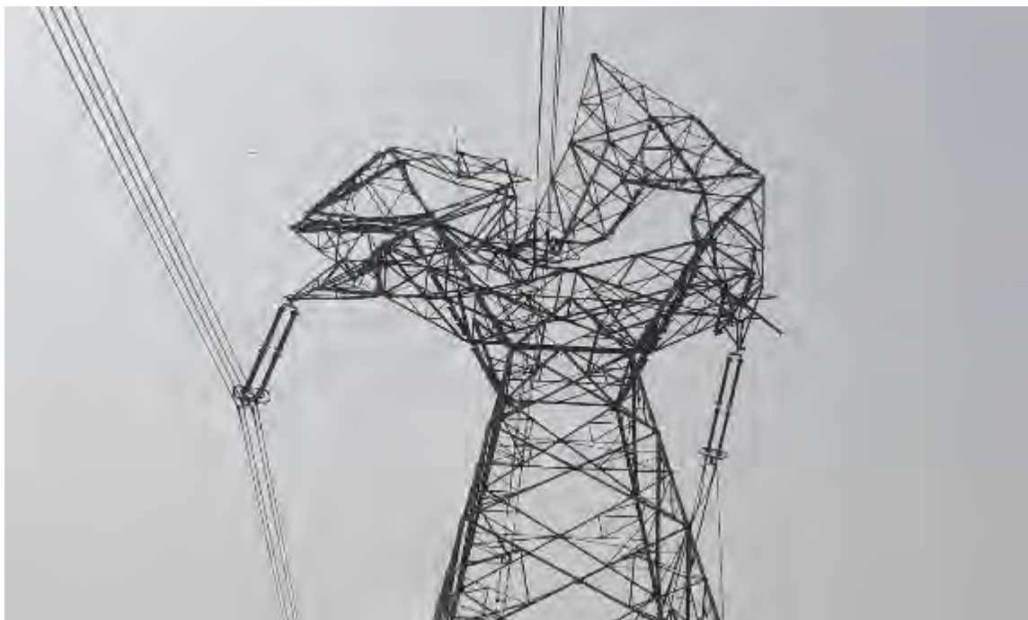
Tower at Loc. No.559 (A+3)
