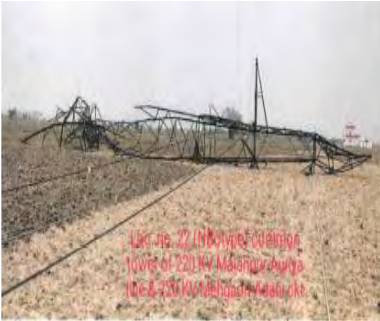
Tower at location 22
