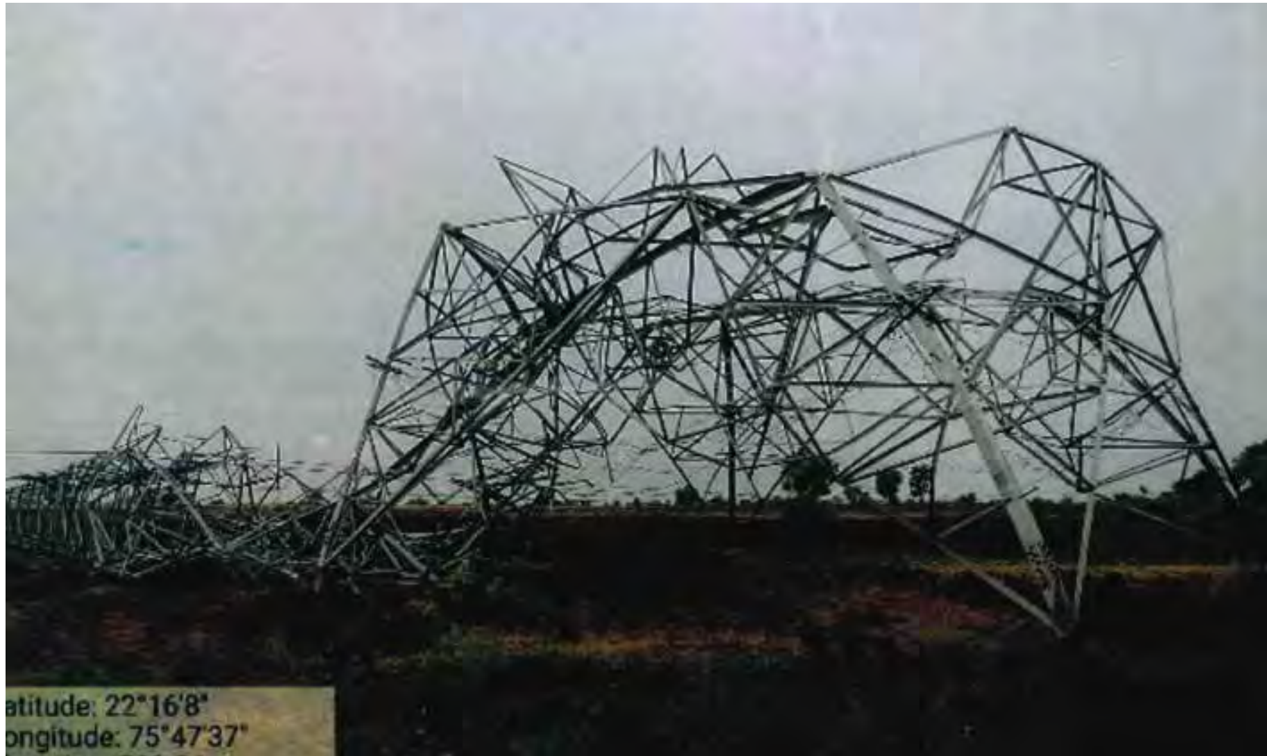
Tower at location 150
