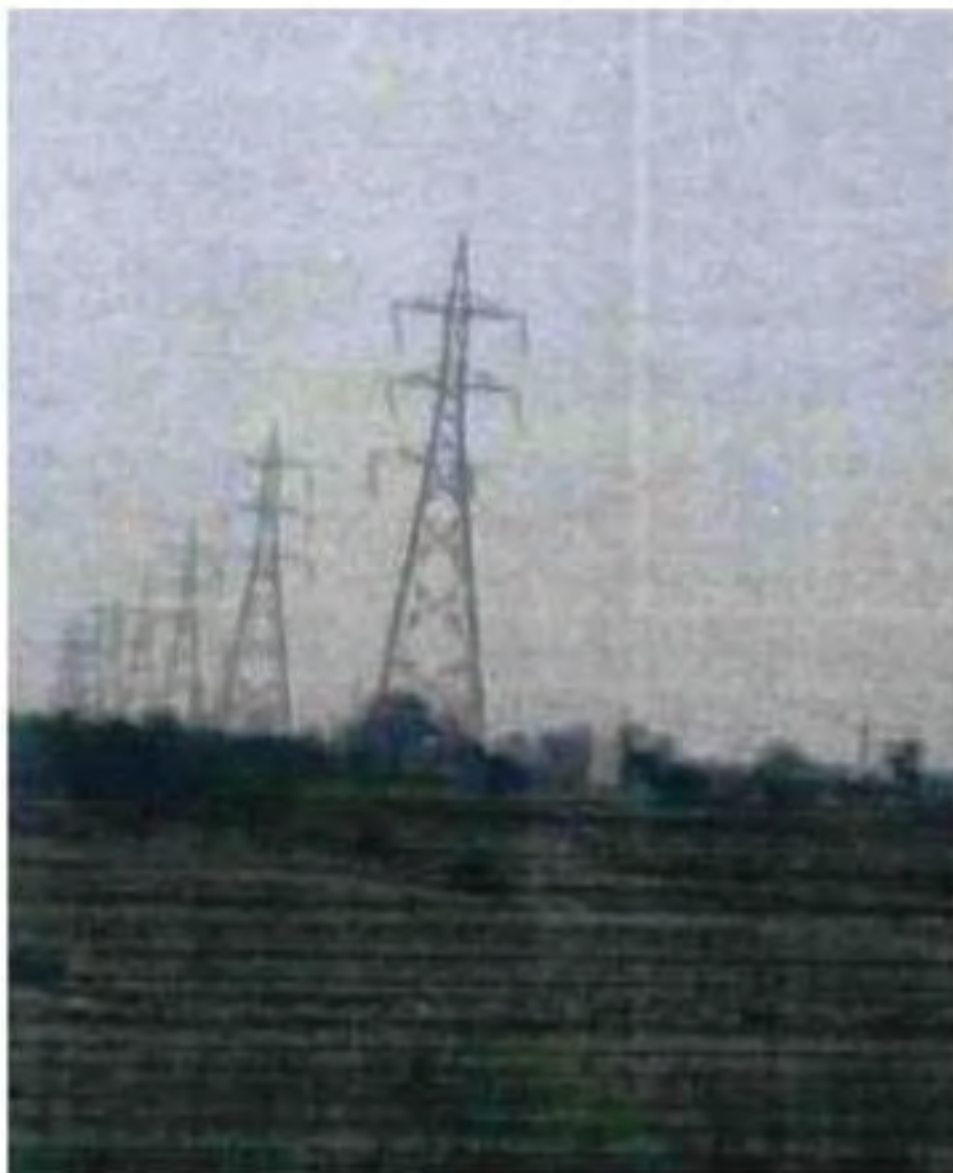
Tower at location 33
