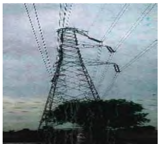
Tower at location No. 152 (FD0+3)
