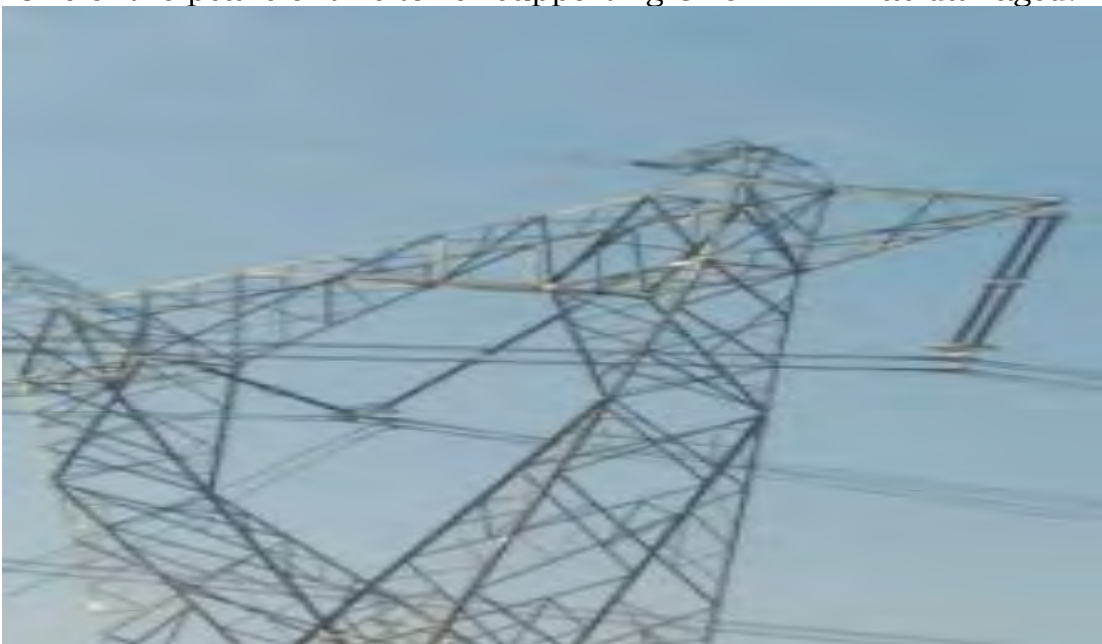
Tower at Loc. No.146 (A+0)
