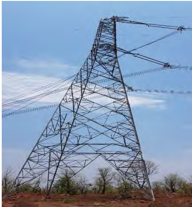
Tower at location No. 18/0 (SD+0)
