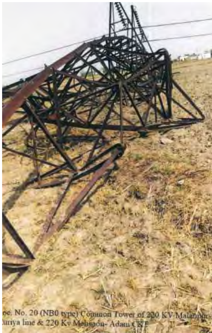
Tower at location 20
