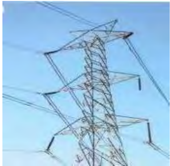
Tower at loc. No. 160 (FD0)
