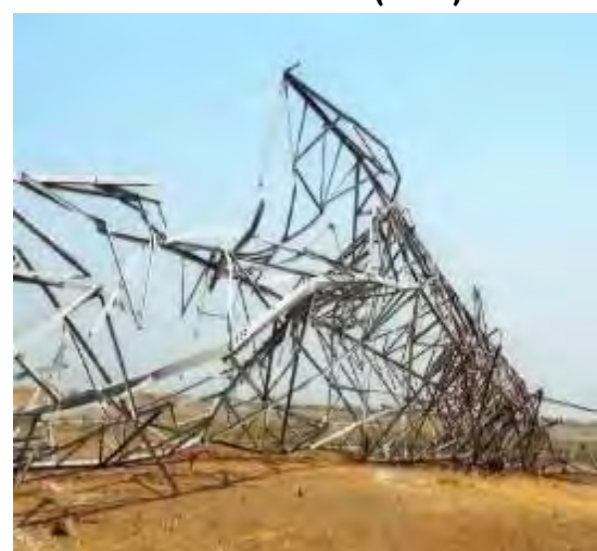
Tower at loc. No. 164 (FD0)
