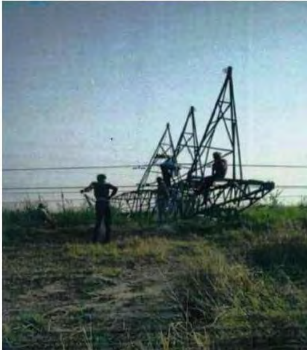
Tower at location 31
