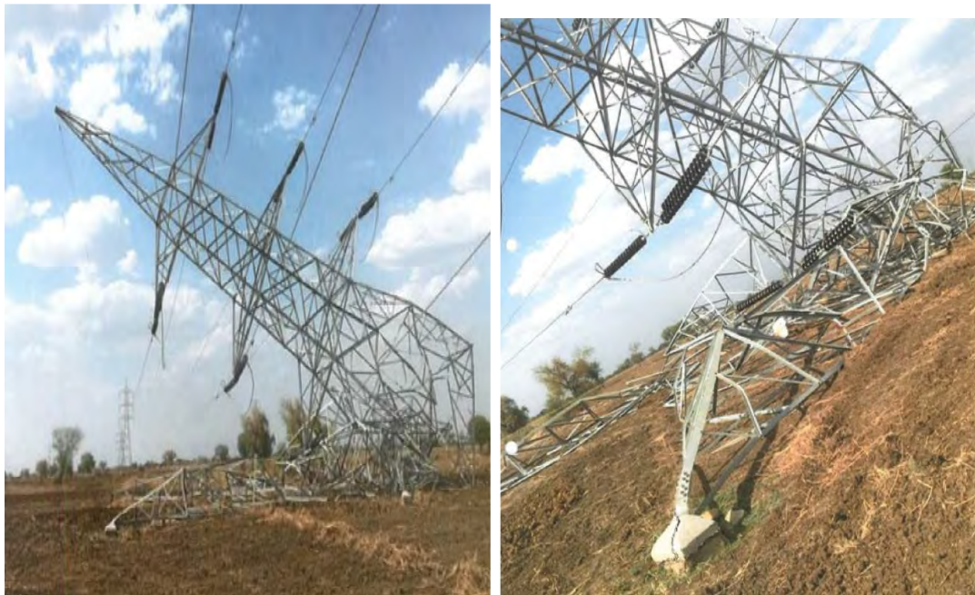
Tower at location No. 390 (DC+15)
