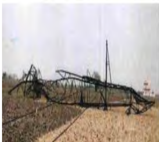
Tower at location No. 22
