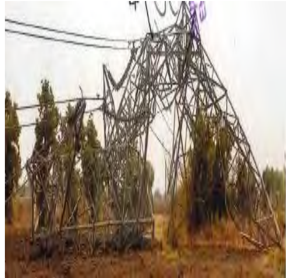
Tower at loc. No. 129 (FD0)
