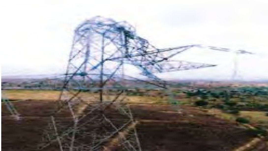
Tower at Location No. 320 (DA+0)
