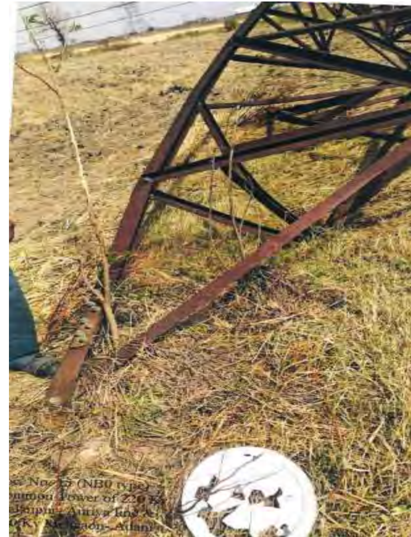
Tower at location 15
