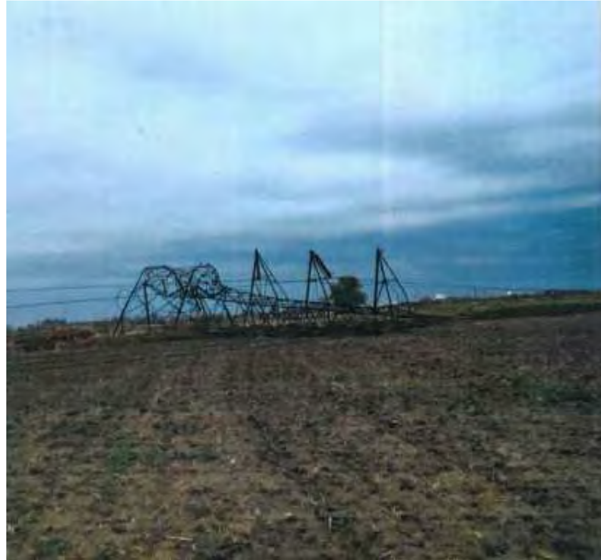
Tower at location 91
