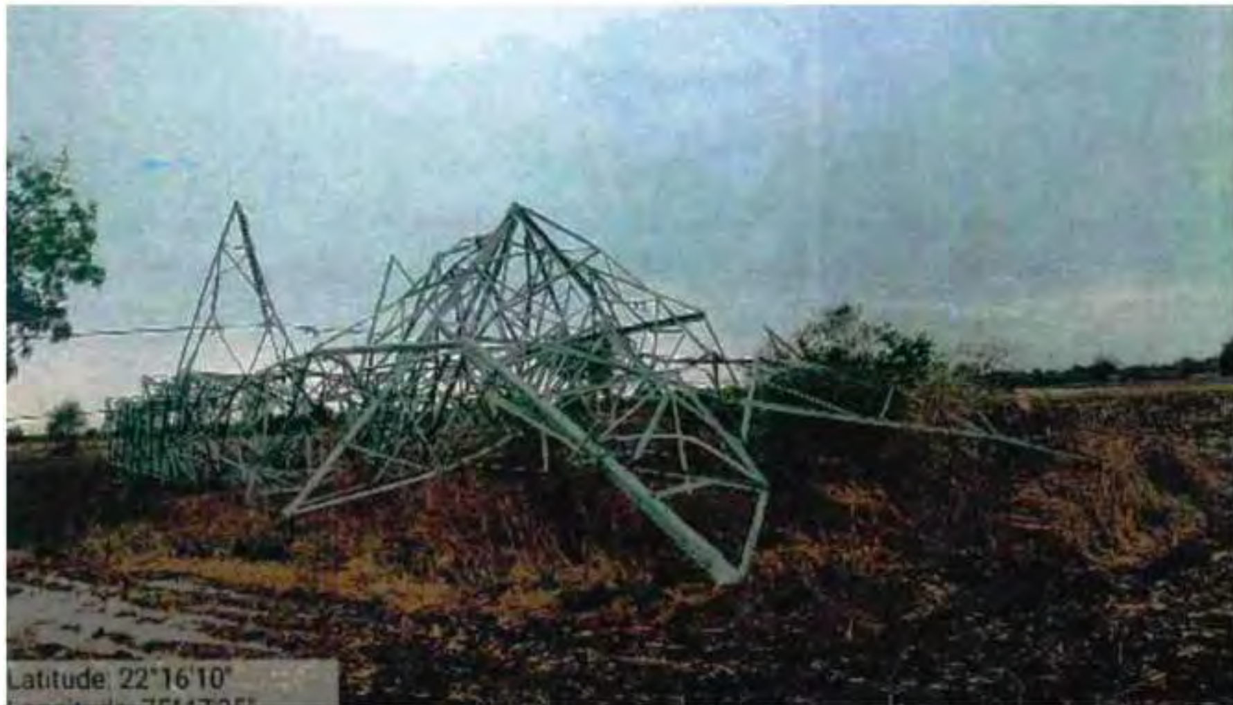
Tower at location 149
