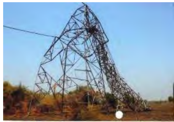
Tower at loc. No. 131 (FD0)
