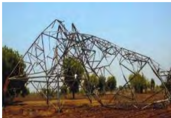
Tower at loc. No. 135 (FD0)
