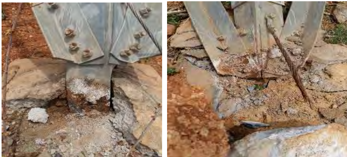
Tower at location No. 365 (DB+0)
