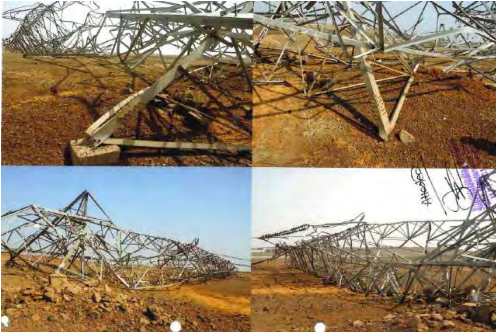
Tower at Location 165
