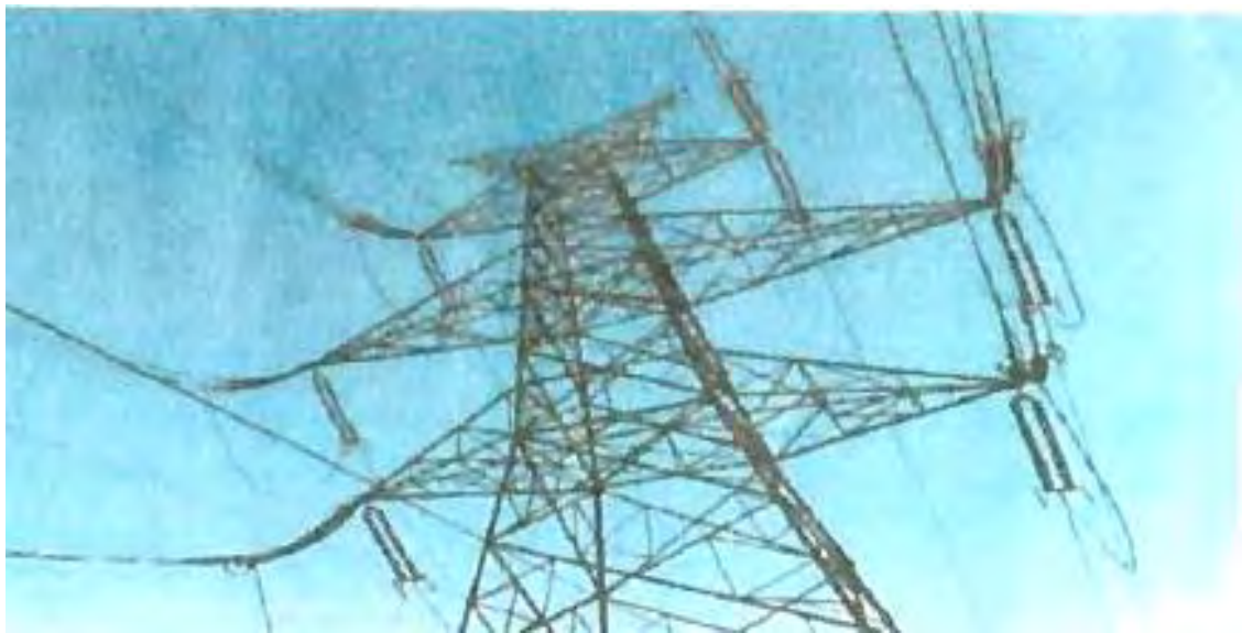
Insertion of Extra Polymer Insulators for Tower at Loc. No.144 (DB+0)
