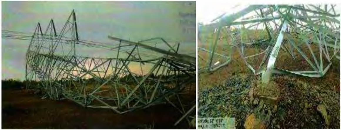
Tower at location No. 148 (FD0)
