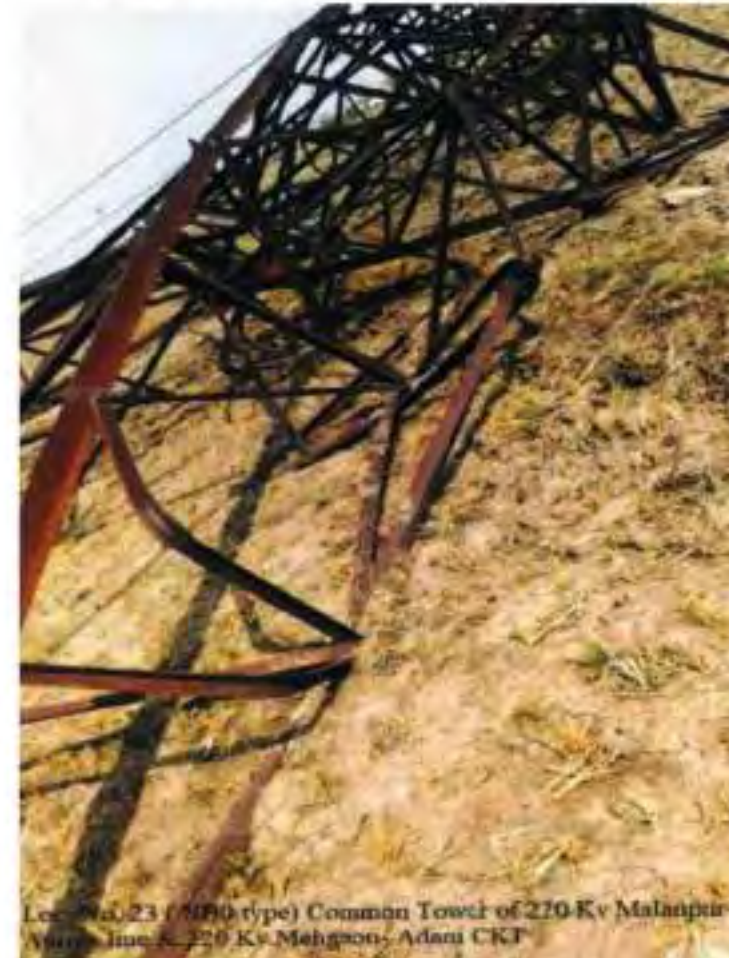
Tower at location 23
