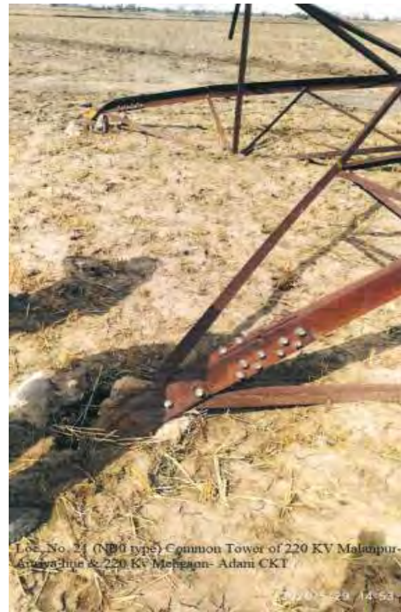
Tower at location 21
