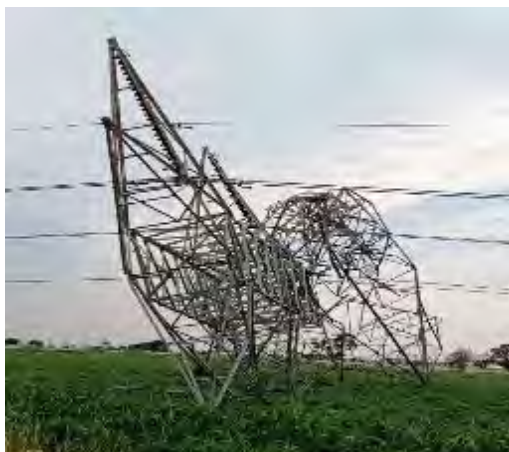
Tower at location No. 15 (FD0)
