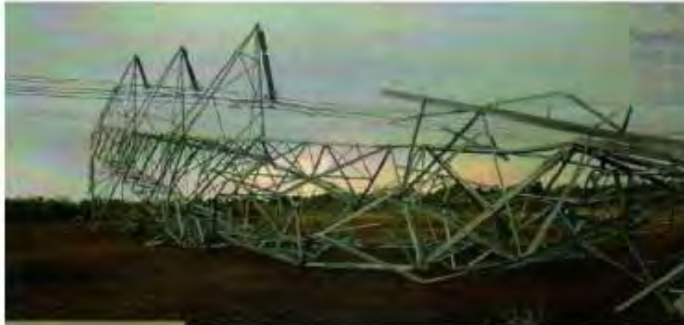
Tower at location 148
