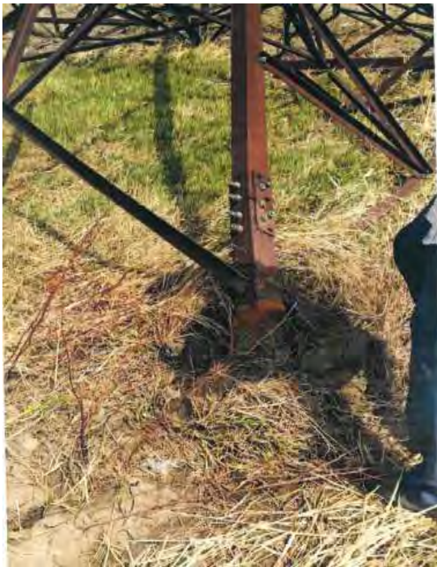
Tower at location 19
