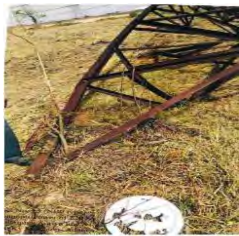
Tower at location No. 15
