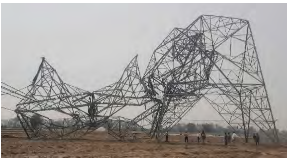
Tower at Loc. No.558 (A+0)
