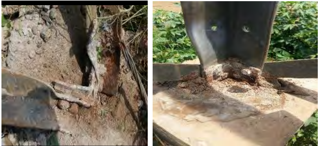
Tower at location No. 361 (DA+3)
