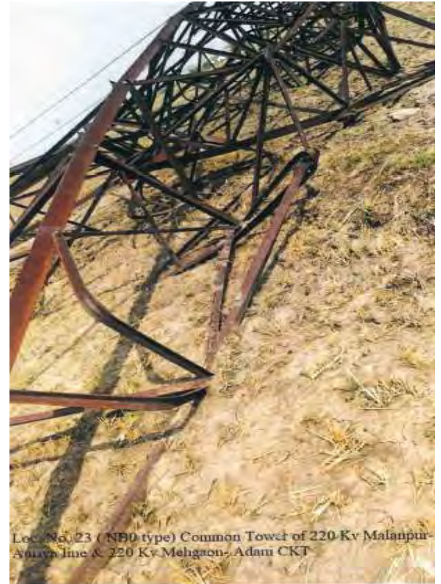
Tower at location 23
