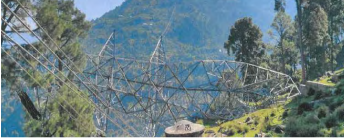
Tower at Location No. 261(DB+6)
