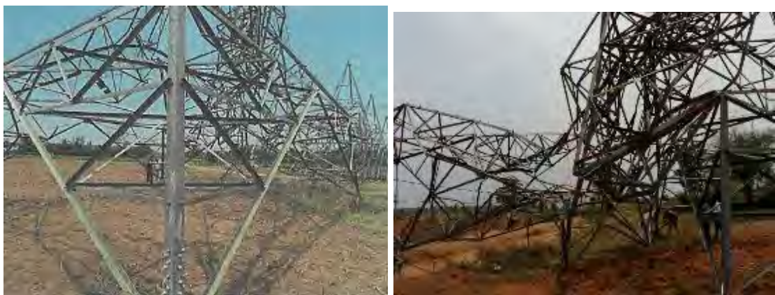
Tower at location No. 362 (DA+3)
