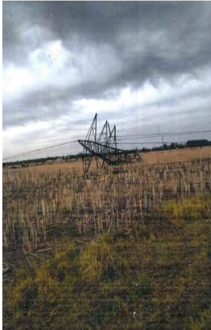
Tower at location 93
