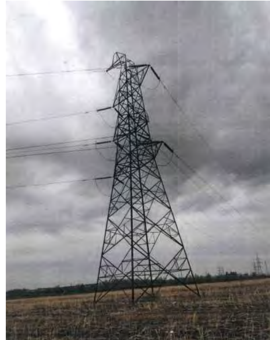
Tower at location 94
