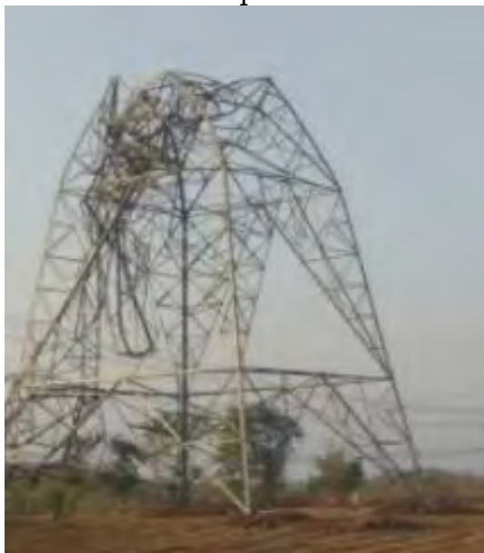
Tower at Loc. No.161 (A+6)
