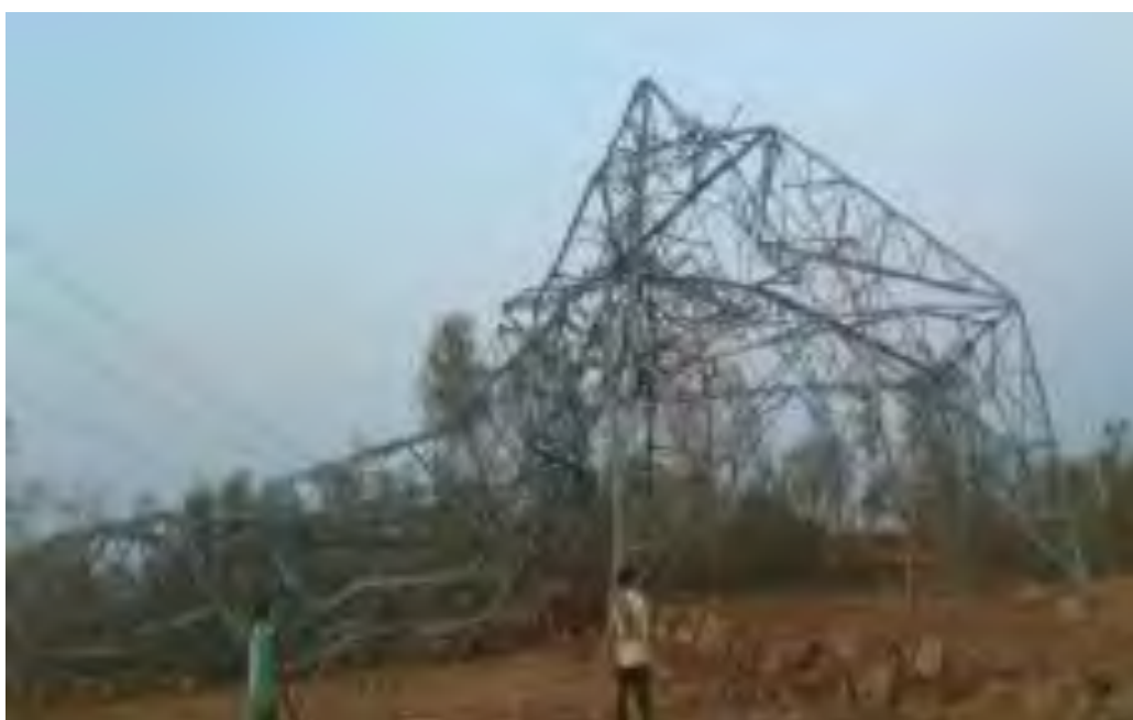
Tower at Loc. No.163 (A+0)
