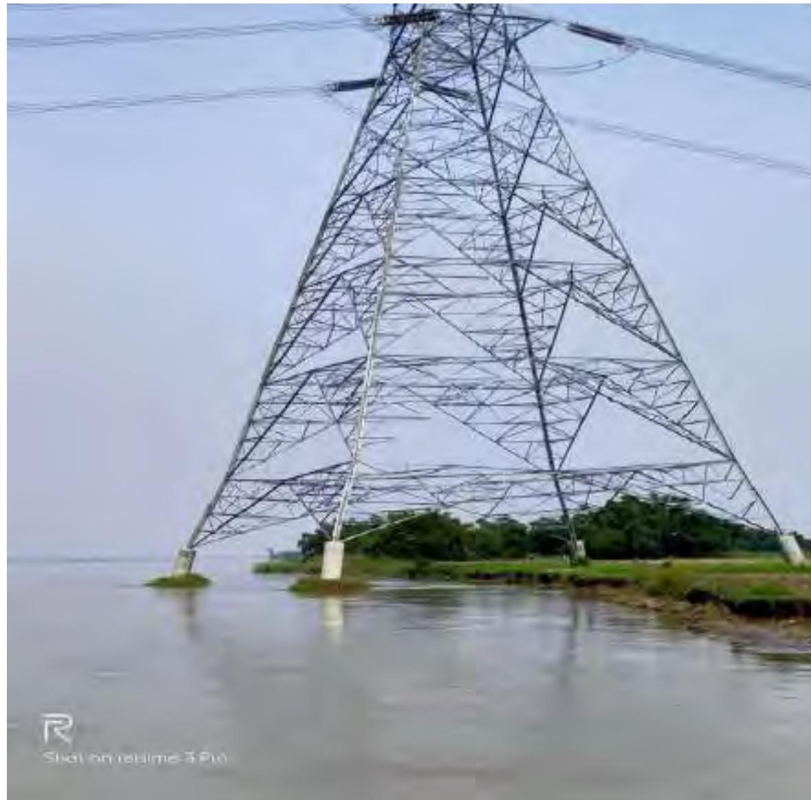
Tilt in tower legs causing bending of members
