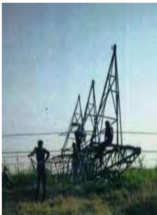
Tower at loc. No. 31 (B0)
