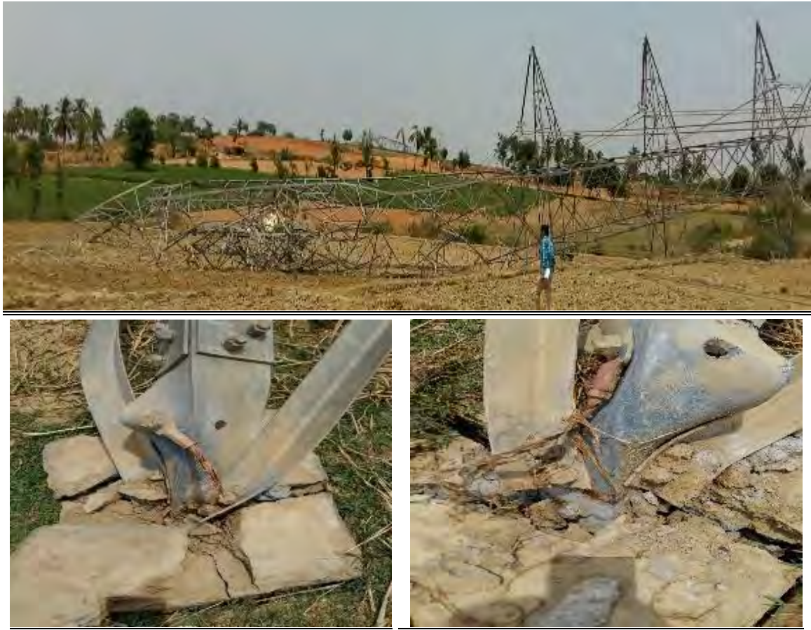
Tower at location No. 364 (DA+9)
