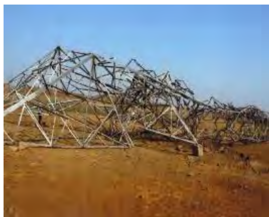
Tower at loc. No. 166 (FD0)
